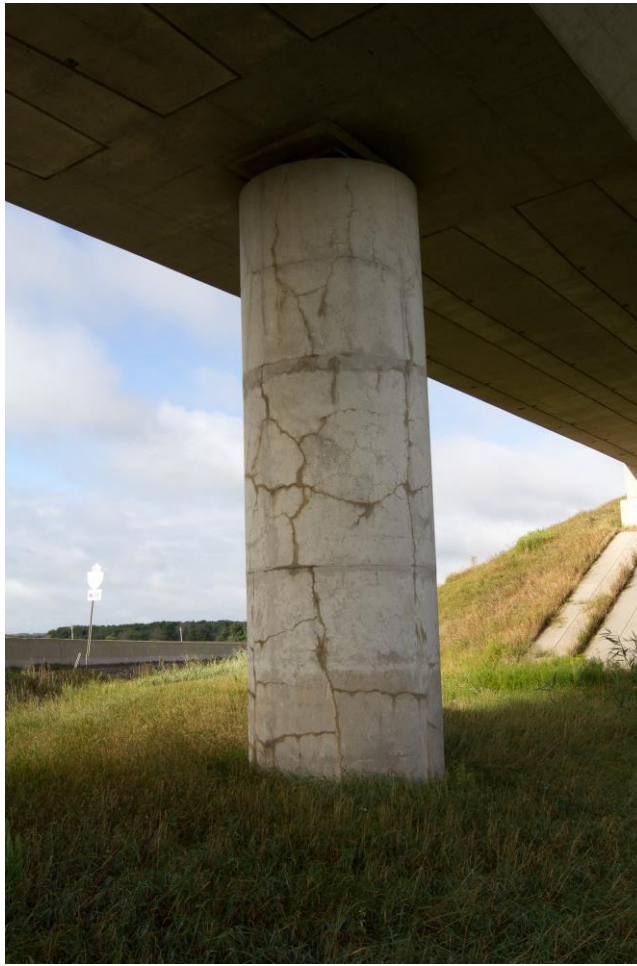
Photograph 4: Looking west at the west pier. Numerous random cracks were observed on the pier. The ground around the pier was well vegetated (August 28, 2015).
