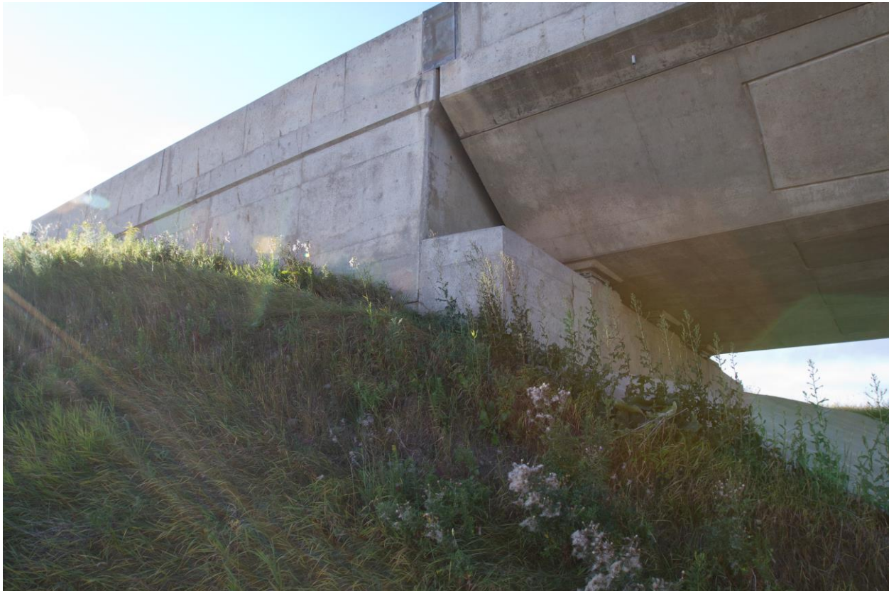
Photograph 6: Looking at the north wingwall and the adjacent slope of the east abutment of the structure. Surficial vertical cracks were observed on the wingwall. The slope is vegetated and effect of erosion on the slope face was not observed (August 28, 2015).
