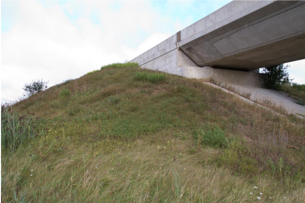
Photograph 7: Looking at the south wingwall and the adjacent slope of the west abutment of the Highway 401 Underpass Structure. Surficial cracks were observed on the wingwall. The slope is vegetated and effect of erosion on the slope face was not observed (August 28, 2015).
