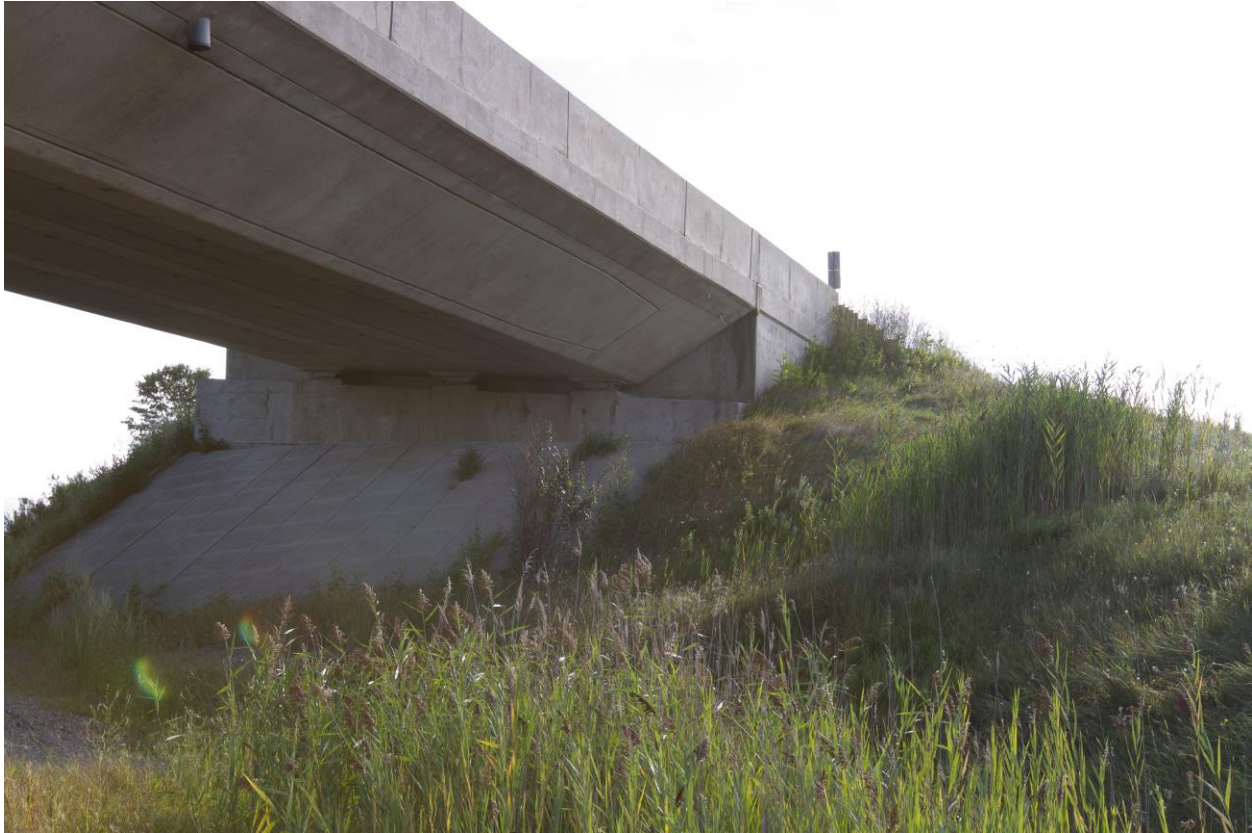
Photograph 5: Looking at the south wingwall and the adjacent slope of the east abutment of the Highway 401 Underpass Structure. Surficial cracks were observed on the wingwall. The slope is vegetated and effect of erosion on the slope face was not observed (August 28, 2015).
