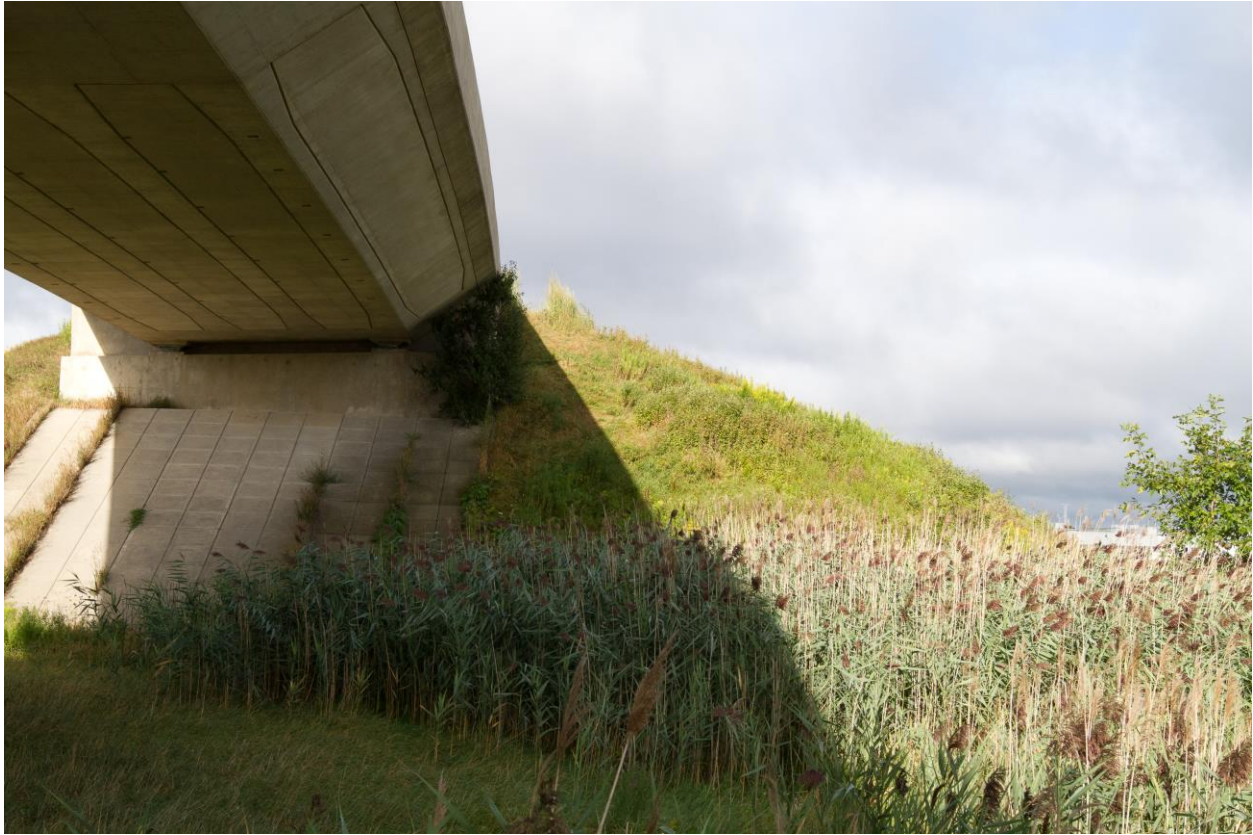
Photograph 8: Looking at the north wingwall and the adjacent slope of the west abutment of the Highway 401 Underpass Structure. Minor surficial cracks were observed on the wingwall. The slope is vegetated and effect of erosion on the slope face was not observed (August 28, 2015).
