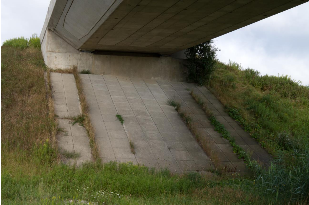
Photograph 2: Looking at the west abutment of the Highway 401 Underpass Structure. Random cracks were observed on the abutment wall. Sealant between the concrete panels appeared degraded at locations where grasses are growing. The toe of the front slope was vegetated at ground surface (August 28, 2015).
