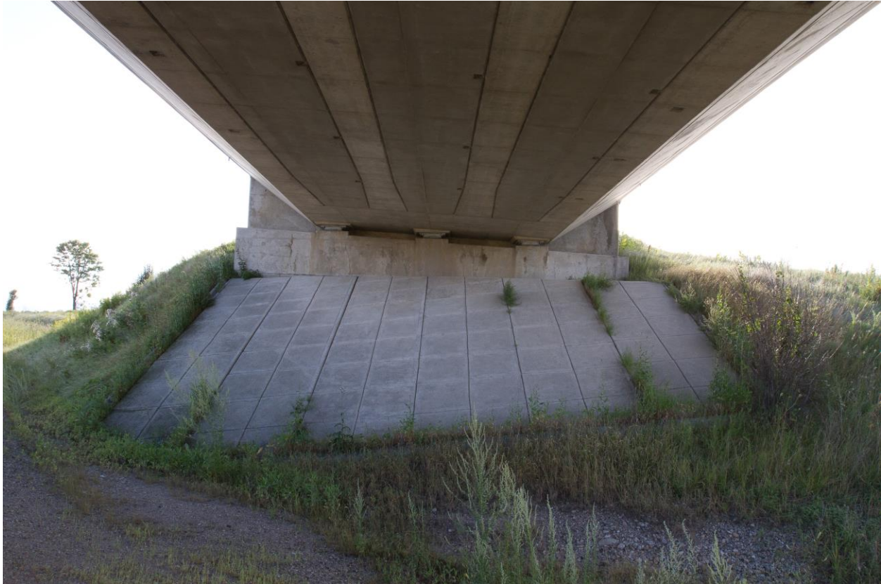
Photograph 1: Looking at the east abutment of the Highway 401 Underpass Structure. Random cracks were observed on the abutment wall. Sealant between the concrete panels appeared degraded at locations where grasses are growing. The toe of the front slope was vegetated with localized erosion of soil at ground surface (August 28, 2015).
