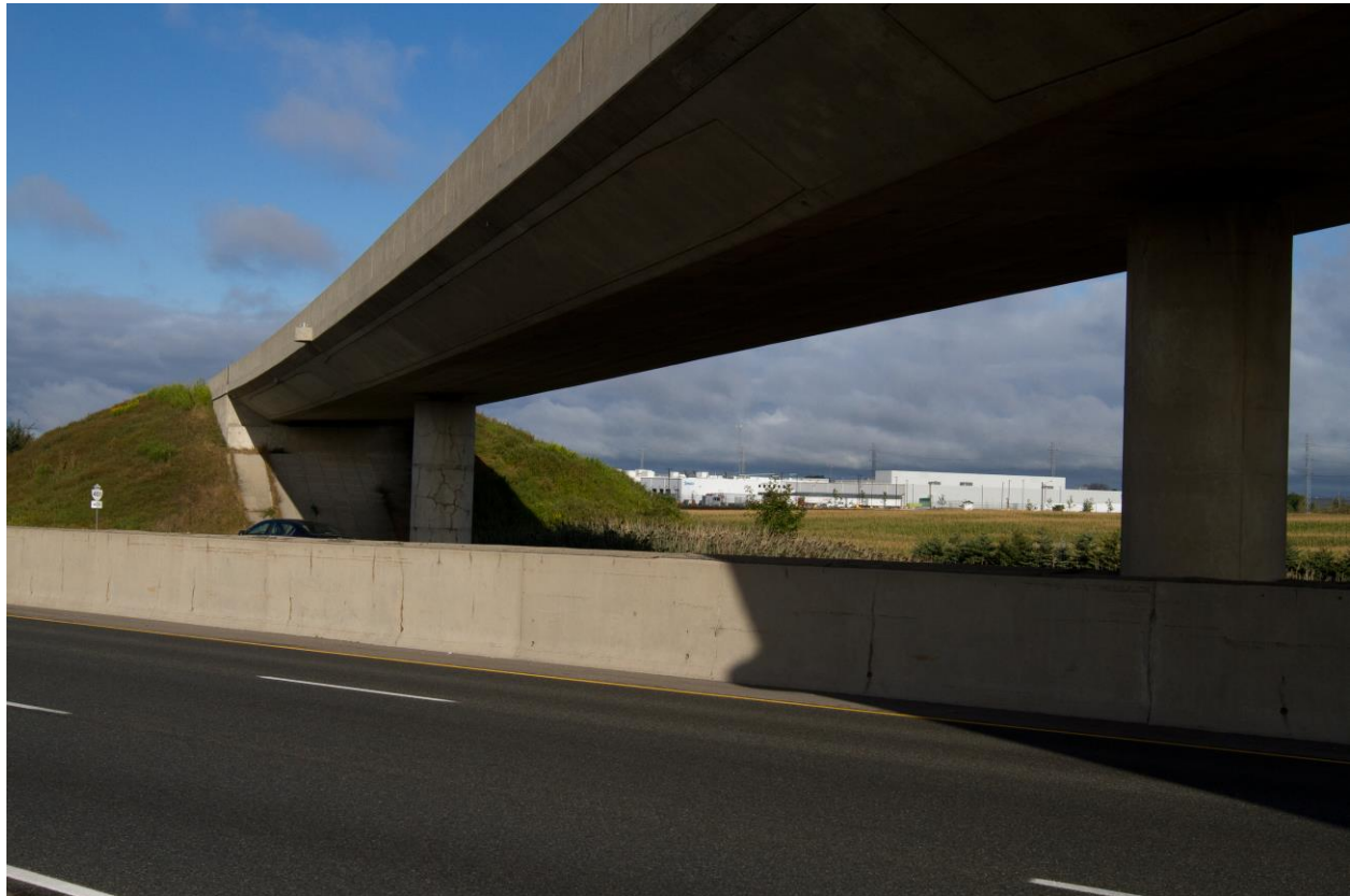
Photograph 3: Looking west at the piers of the Highway 401 Underpass Structure. Numerous cracks were observed on the west pier. (August 28, 2015).
