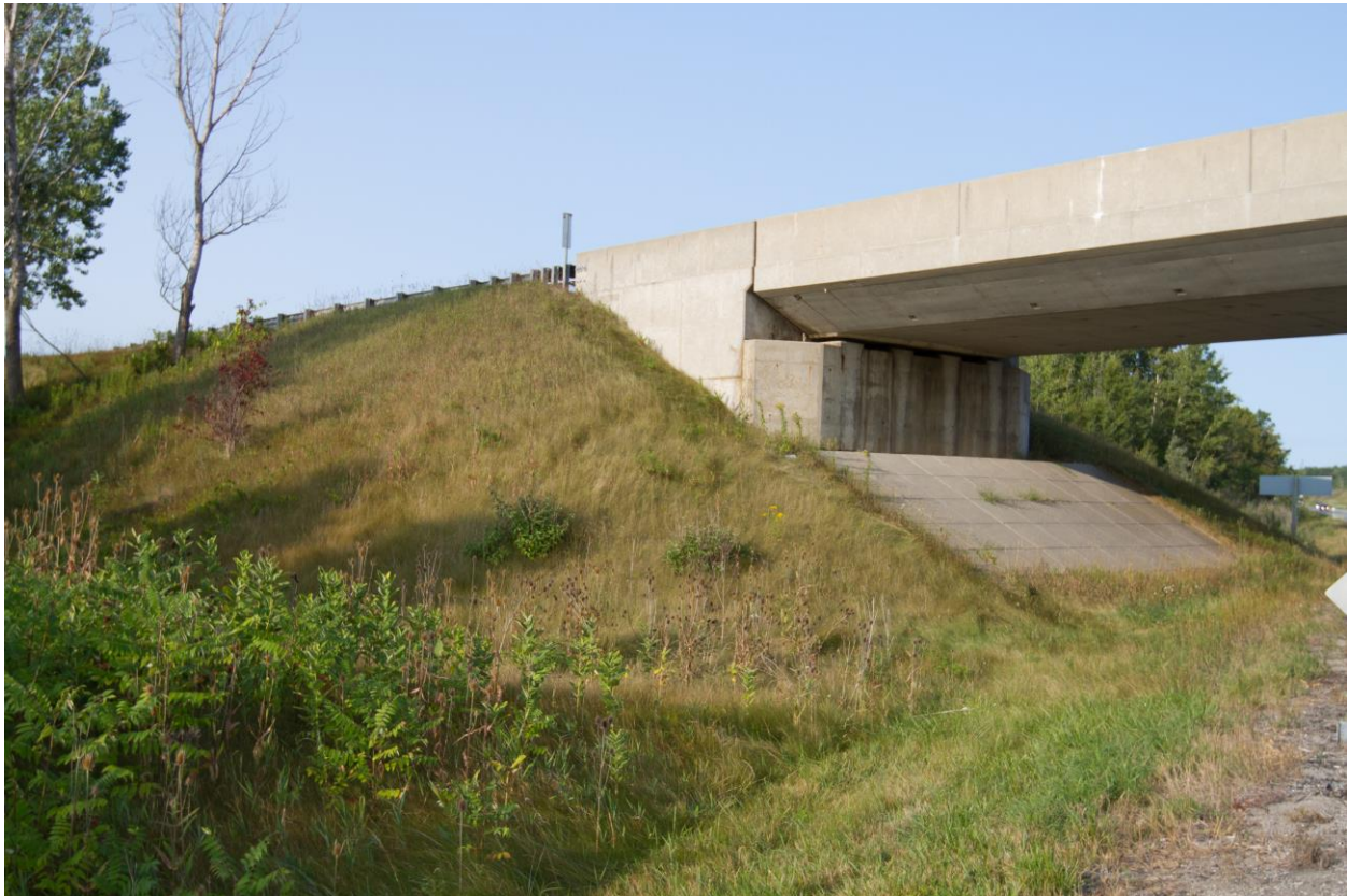
Photograph 5: Looking at the east wingwall and the adjacent slope of the south abutment of the Brant Road 16 Underpass Structure. Minor surficial cracks were observed on the wingwall. The slope is vegetated and effect of erosion on the slope face was not observed (August 28, 2015).
