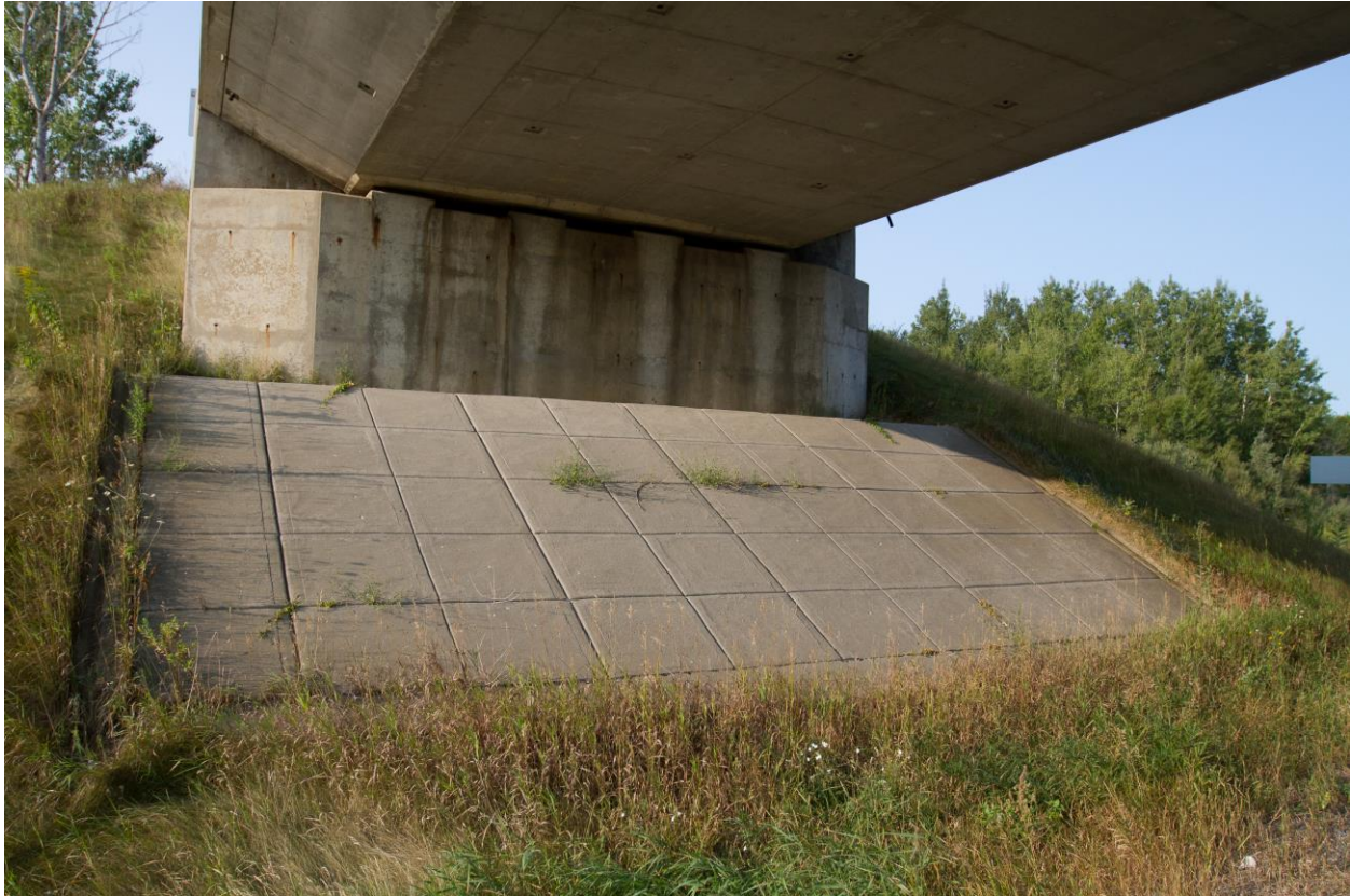
Photograph 1: Looking at the south abutment of the Brant Road 16 Underpass Structure. No damages were observed on the front slope concrete panels. Minor surficial cracks were observed on the abutment walls. Weep holes were observed in the abutment wall. The adjacent slopes and the toe of the front slope were vegetated. Erosion of the slopes was not observed (August 28, 2015).
