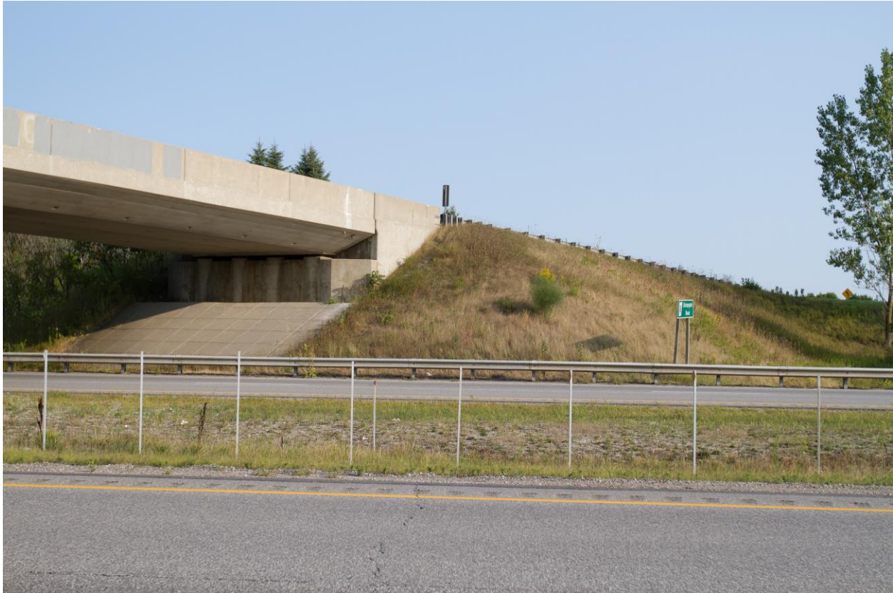
Photograph 8: Looking at the east wingwall and the adjacent slope of the north abutment of the Brant Road 16 Underpass Structure. Minor surficial cracks were observed on the wingwall. The slope is vegetated and effect of erosion on the slope face was not observed (August 28, 2015).
