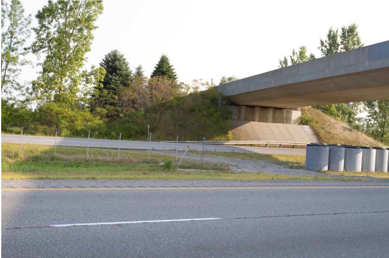
Photograph 7: Looking at the west wingwall and the adjacent slope of the north abutment of the Brant Road 16 Underpass Structure. Minor surficial cracks were observed on the wingwall. The slope is vegetated and effect of erosion on the slope face was not observed (August 28, 2015).
