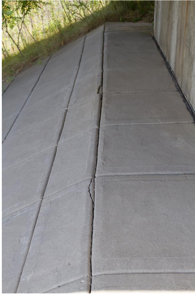
Photograph 3: Minor cracks observed on the concrete panels of the north abutment of the Brant Road 16 Underpass Structure (August 28, 2015).
