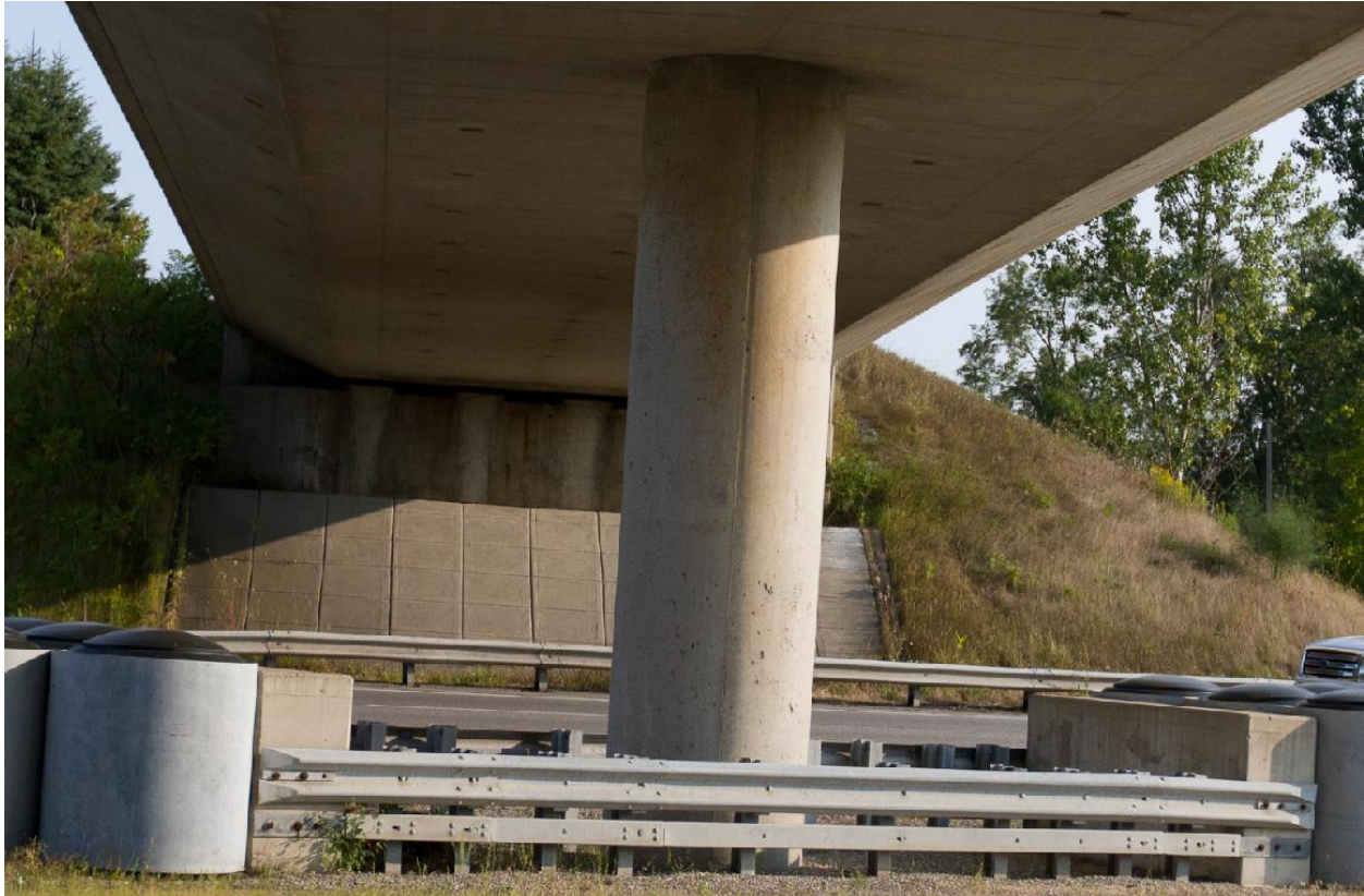
Photograph 4: Looking north at the centreline pier of the Brant Road 16 Underpass Structure. Minor surficial cracks were observed on the pier (August 28, 2015).
