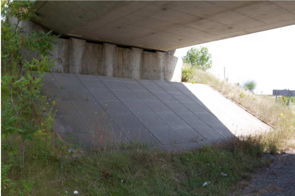
Photograph 2: Looking at the north abutment of the Brant Road 16 Underpass Structure. Minor damages were observed on the front slope concrete panels. Minor surficial cracks were observed on the abutment walls. Weep holes were observed in the abutment wall. The adjacent slopes and the toe of the front slope were vegetated. Erosion of the slopes was not observed (August 28, 2015).
