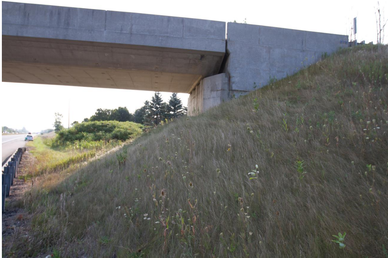
Photograph 6: Looking at the west wingwall and the adjacent slope of the south abutment of the Brant Road 16 Underpass Structure. Minor surficial cracks were observed on the wingwall. The slope is vegetated and effect of erosion on the slope face was not observed (August 28, 2015).
