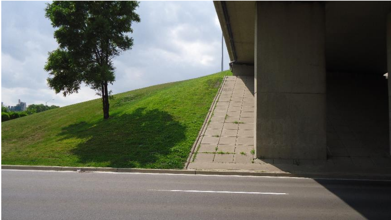
Photograph 1: Looking west at the adjacent south slope of the structure. The slope was covered with vegetation. No erosion effect was observed on the slope face and toe (July 31, 2014).
