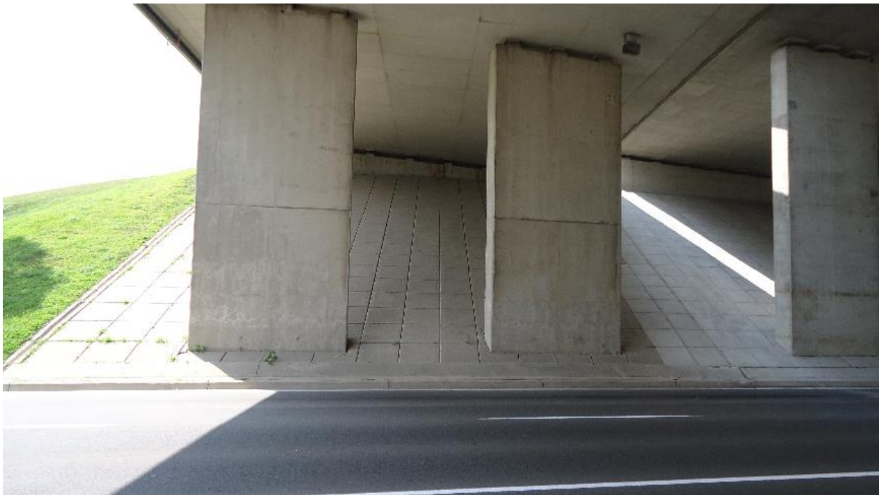
Photograph 4: Looking at the west piers. No obvious major cracks were observed except some surface cracks (July 31, 2014).
