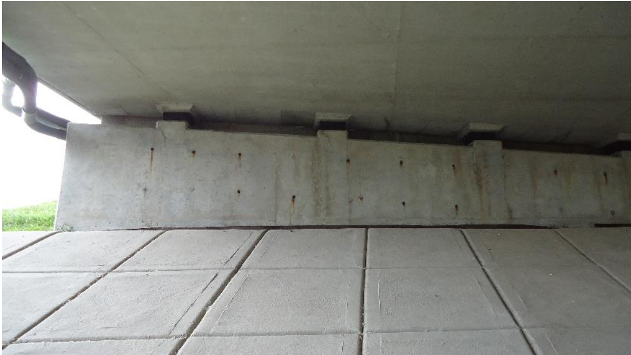
Photograph 3: Looking at the west abutment. Surficial cracks were observed on the wall (July 31, 2014).
