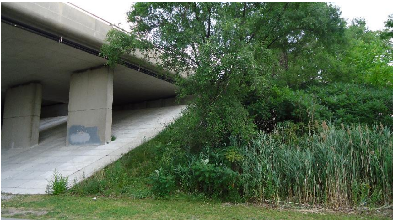
Photograph 8: Looking at the adjacent east south slope. The slope was heavily vegetated. No erosion effects were observed on the slope face and toe (July 31, 2014).
