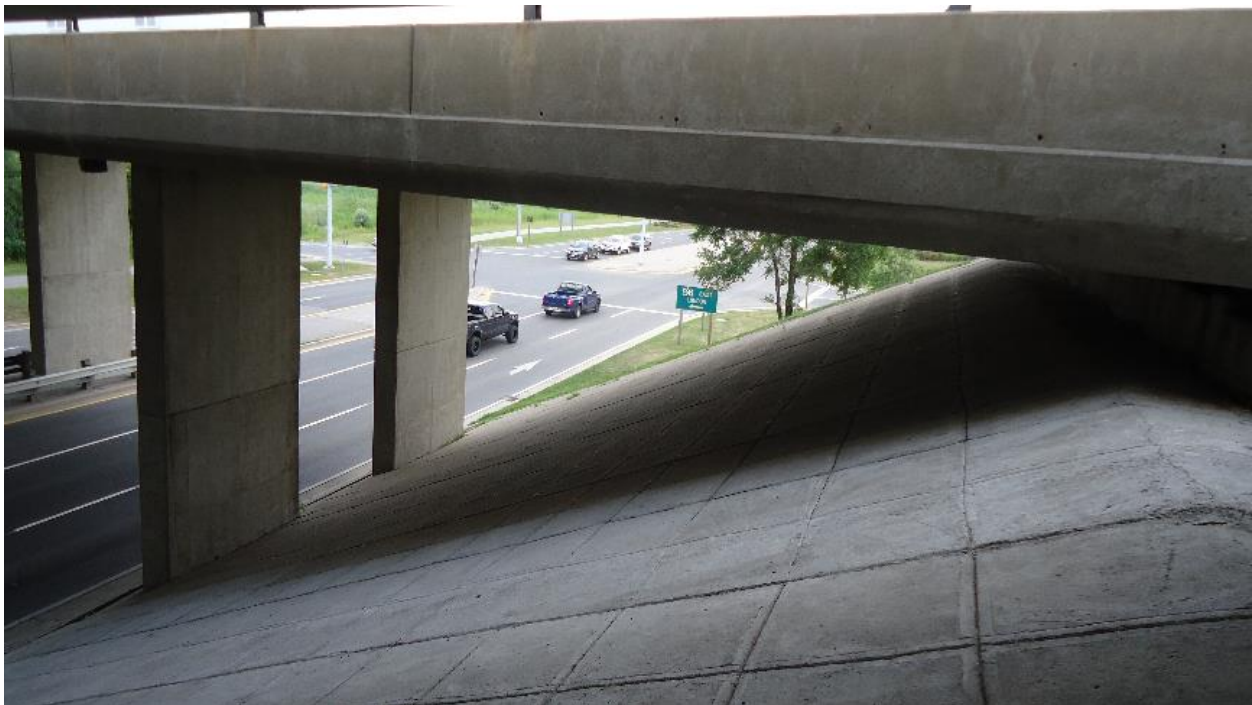
Photograph 2: Looking southeast towards the west front slope which was covered with concrete panels. No obvious major cracks or settlement effects were observed on the concrete paved slope (July 31, 2014).
