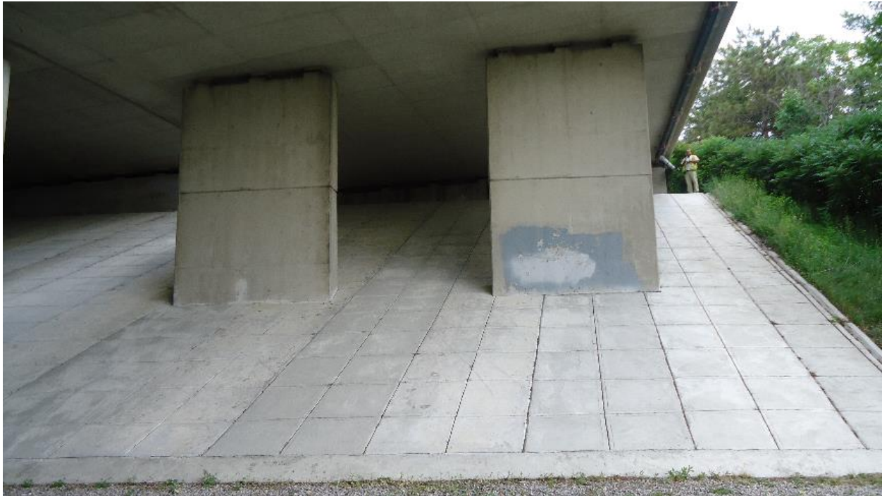
Photograph 7: Looking to the east pier and abutment. The front slope covered with concrete panels. Some rehabilitation work was completed on the piers (July 31, 2014).
