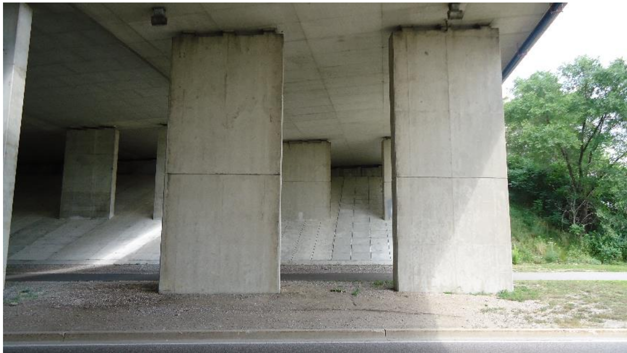
Photograph 6: Looking east at the center pier. No erosion effects were observed around the piers. Surficial crack were observed on the piers (July 31, 2014).
