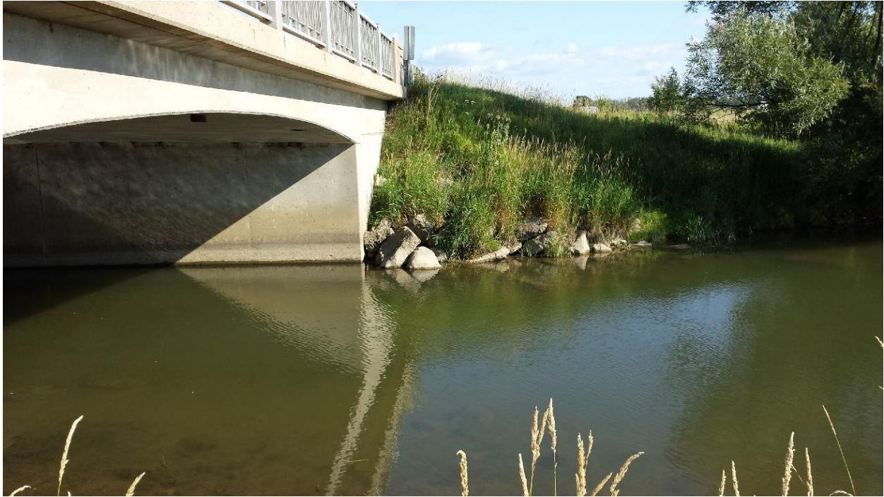
Photograph 6: Looking south at the west slope adjacent to the south abutment wall. Rocks were placed at the toe and face of the slope to prevent erosion and scouring. (July 24, 2014)
