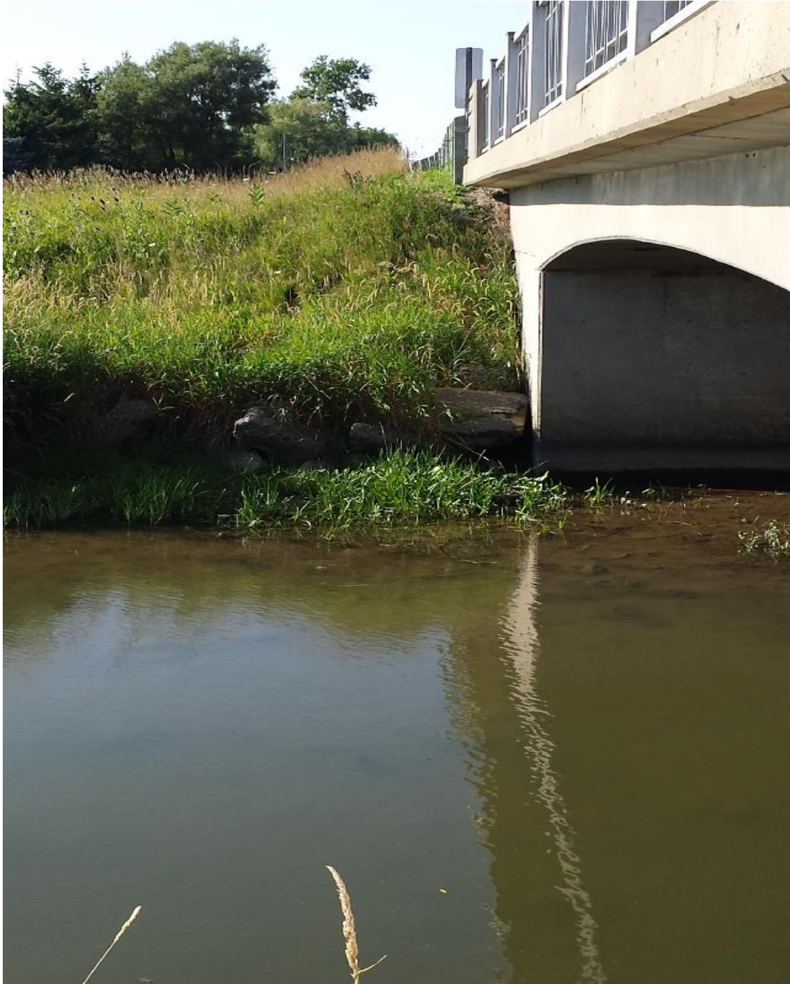
Photograph 3: Looking north at the adjacent west slope of the north abutment. The slope was covered by bushes. Rocks were observed at the toe of the slope to prevent further scouring. (July 24, 2014)
