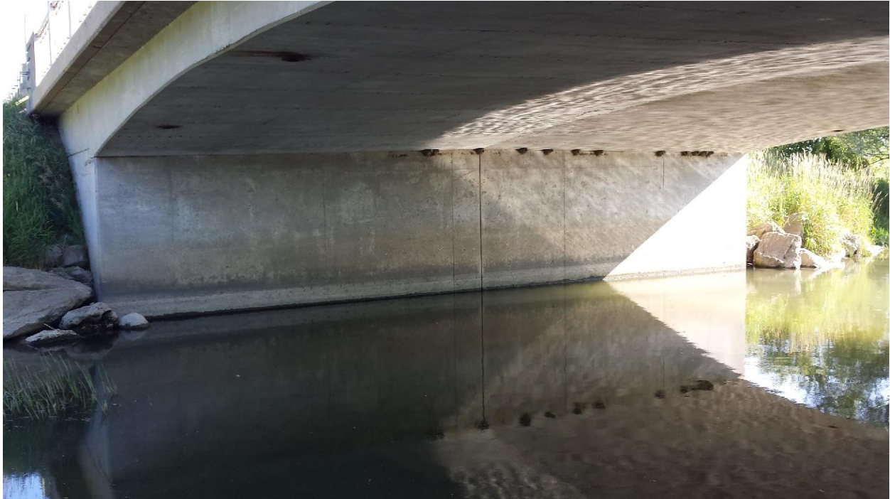
Photograph 4: Looking at the south abutment wall from the northeast corner of the bridge site. No obvious cracks were observed except for some surface cracks. Scouring effect below the water could not be established. (July 24, 2014)
