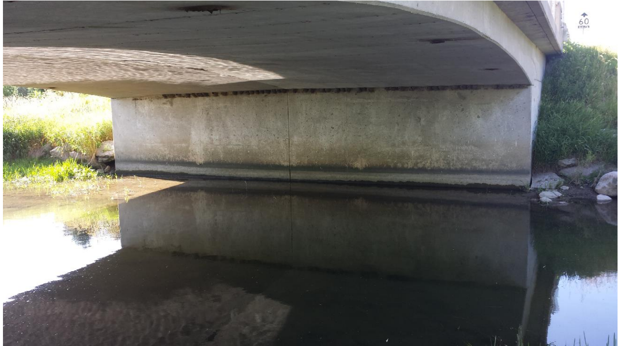
Photograph 1: Looking at the north abutment from the southeast corner of the bridge site. No obvious cracks were observed on concrete. Scouring effect below the water could not be established. (July 24, 2014)
