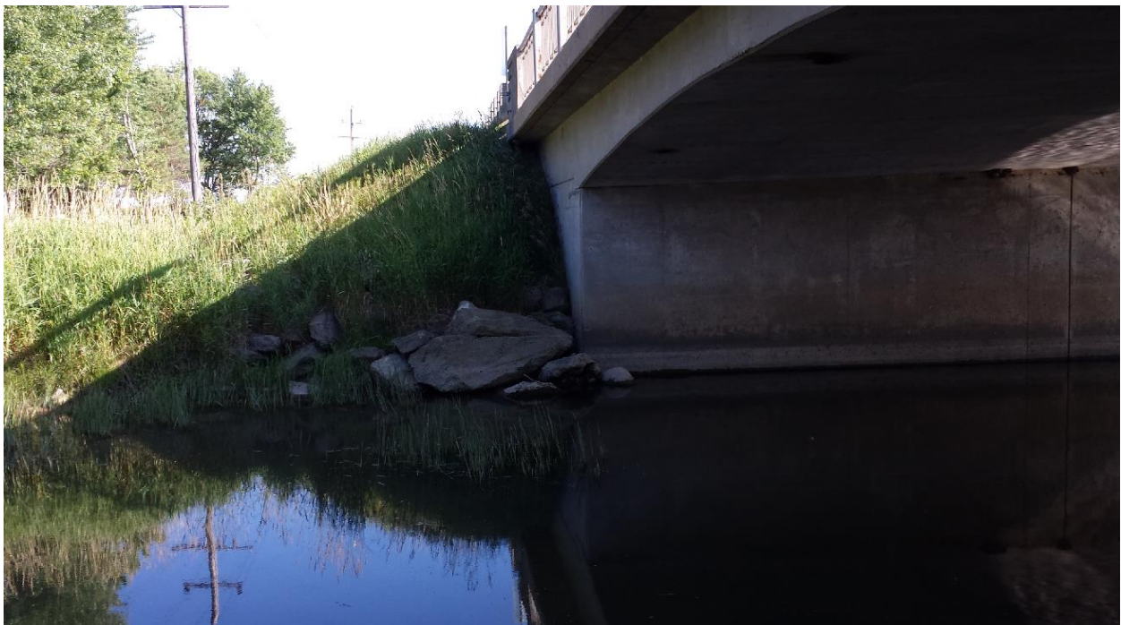
Photograph 5: Looking south at the east slope adjacent to the south abutment. Rocks were placed at the toe and face of the slope to prevent erosion and scour. (July 24, 2014)
