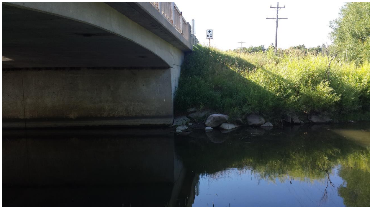
Photograph 2: Looking north at the east adjacent slope. The slope was covered with grass and bushes. Rock pieces were observed at the slope toe to protect from scouring effects. (July 24, 2014)
