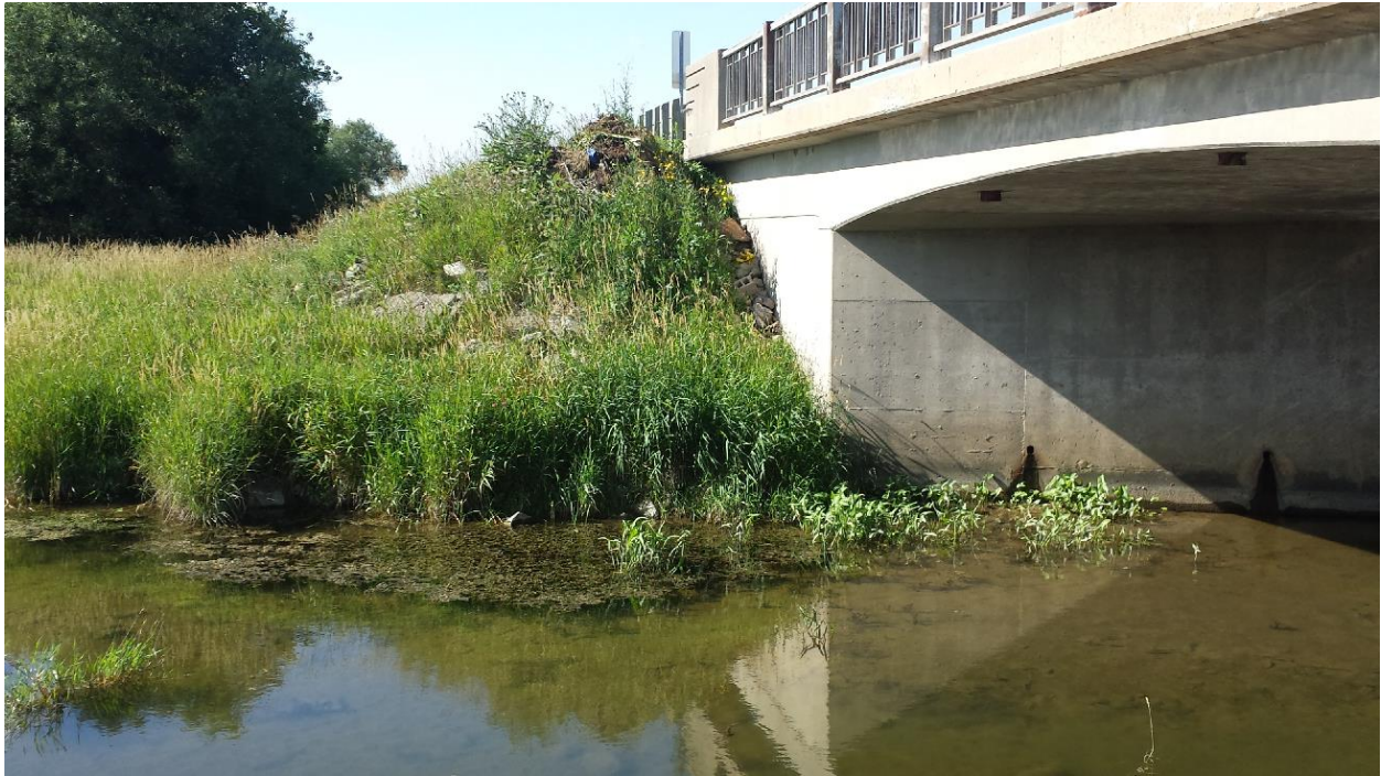
Photograph 3: Looking north at the west slope adjacent to the north abutment. The slope face was vegetated. However, previous construction debris was observed on the slope face. (July 24, 2014)
