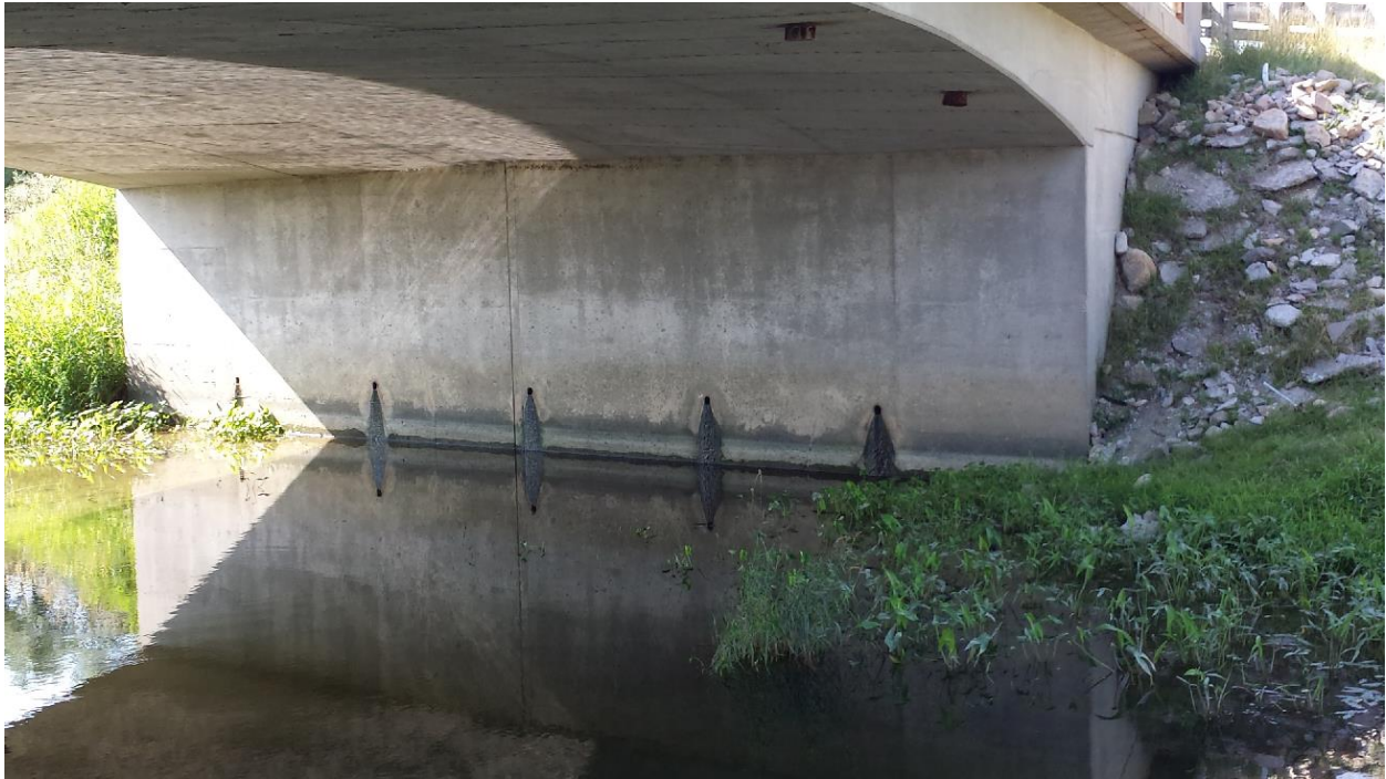
Photograph 1: Looking north at the north abutment. No obvious cracks were observed on abutment wall except some surficial cracks. Weep holes observed in the abutment wall were open and wet. (July 24, 2014)
