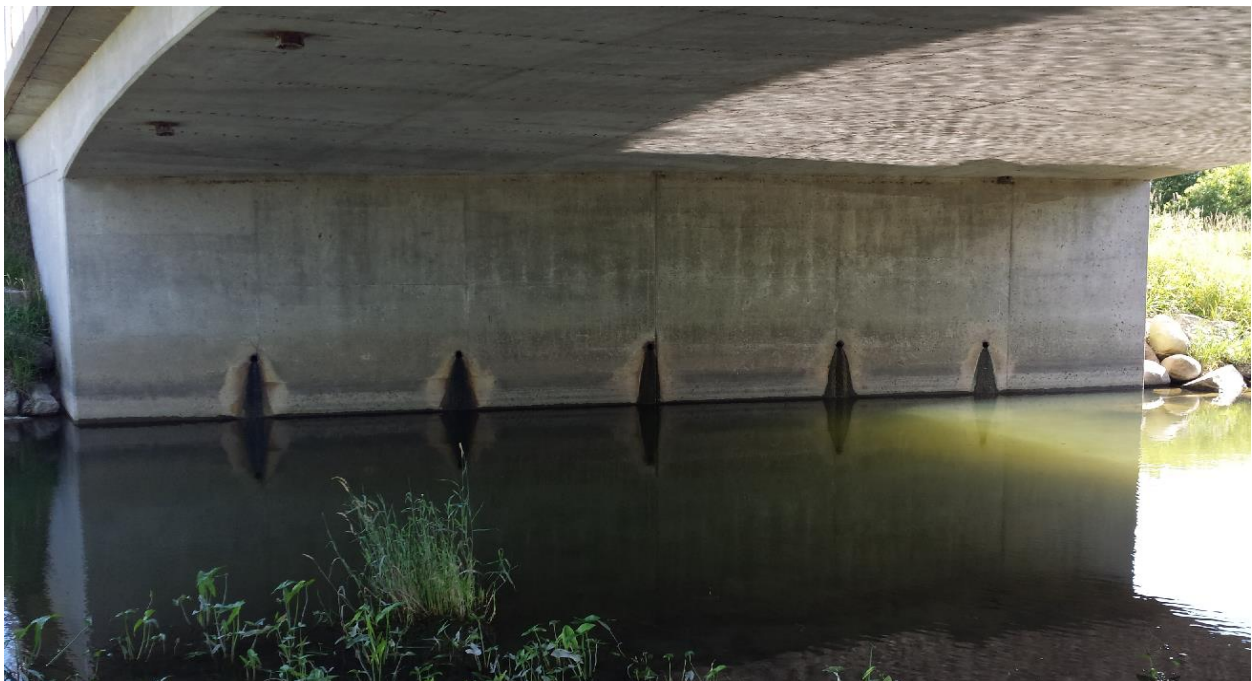
Photograph 4: Looking at the south abutment from the northeast corner of the bridge. No obvious cracks were observed on the abutment wall, except some surficial cracks. Weep holes in the abutment wall were open and wet. (July 24, 2014)
