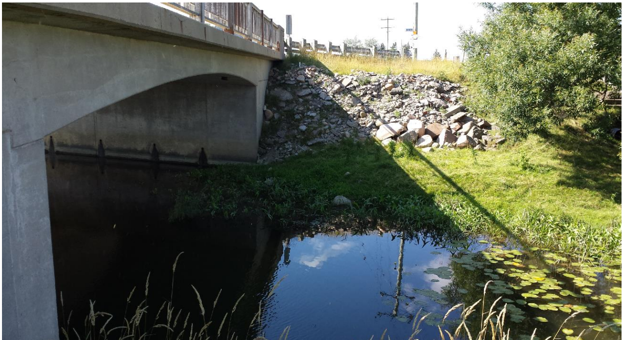
Photograph 2: Looking north at the east slope adjacent to the north abutment. Rip-rap protection was observed on the slope face to prevent further erosion of the exposed earth. (July 24, 2014)
