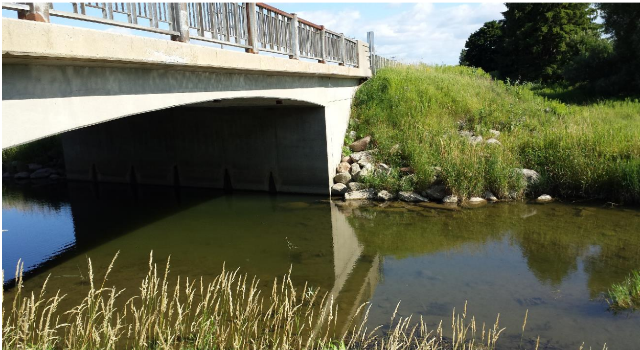
Photograph 6: Looking south at the west slope adjacent to the south abutment. The slope face observed was vegetated with rip-rap placed on the face and at the toe of the slope to prevent erosion and scour of the exposed earth. (July 24, 2014)
