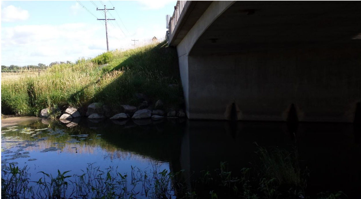
Photograph 5: Looking south at the east slope adjacent to the south abutment. The slope face was vegetated. Rip-rap was observed at the toe of the slope. (July 24, 2014)
