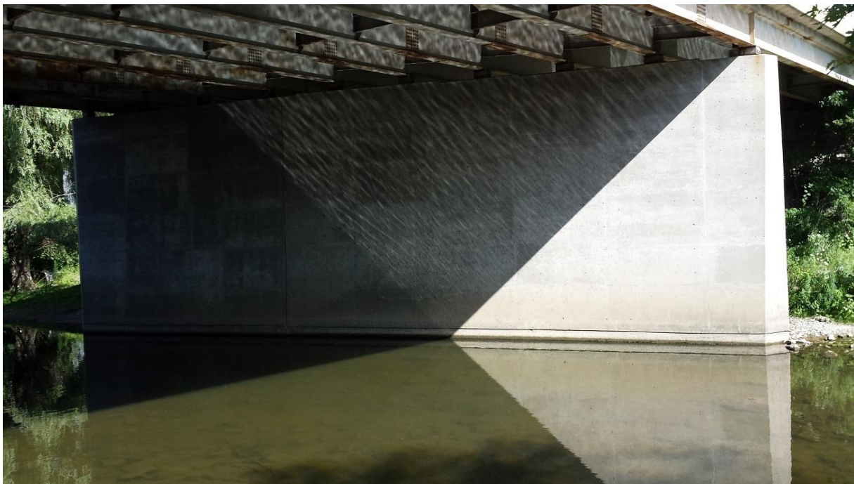
Photograph 10: Looking south at the south pier wall from the northwest corner. No obvious cracks were observed on the concrete pier. Scouring effect below the water could not be established during the site reconnaissance. (July 24, 2014)
