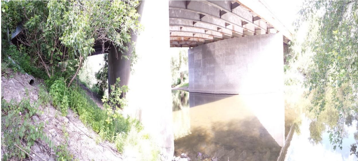
Photograph 7: Looking east at the bridge structure from the northwest corner. Erosion of exposed earth was evident on the slope face and adjacent to the north pier. (July 24, 2014)
