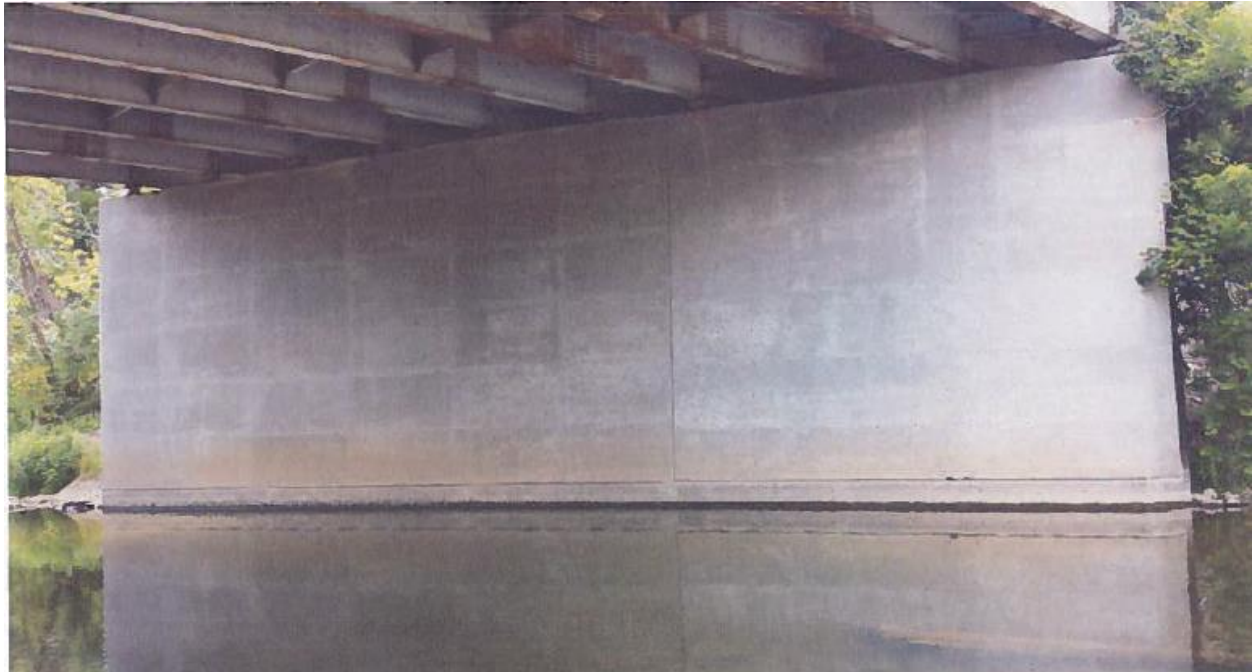
Photograph 3: Looking north at the north pier wall from the southeast corner. No obvious cracks were observed on the concrete pier. Scouring effect below the water could not be established during the site reconnaissance. (July 24, 2014)
