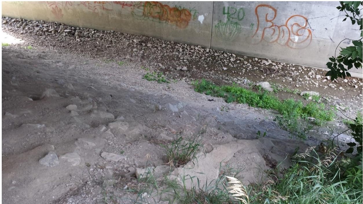
Photograph 5: Looking down at the slope face in front of the south abutment. Effects of erosion were observed on the slope face and the exposed earth in front of the south pier. There were no obvious cracks on the pier wall. (July 24, 2014)
