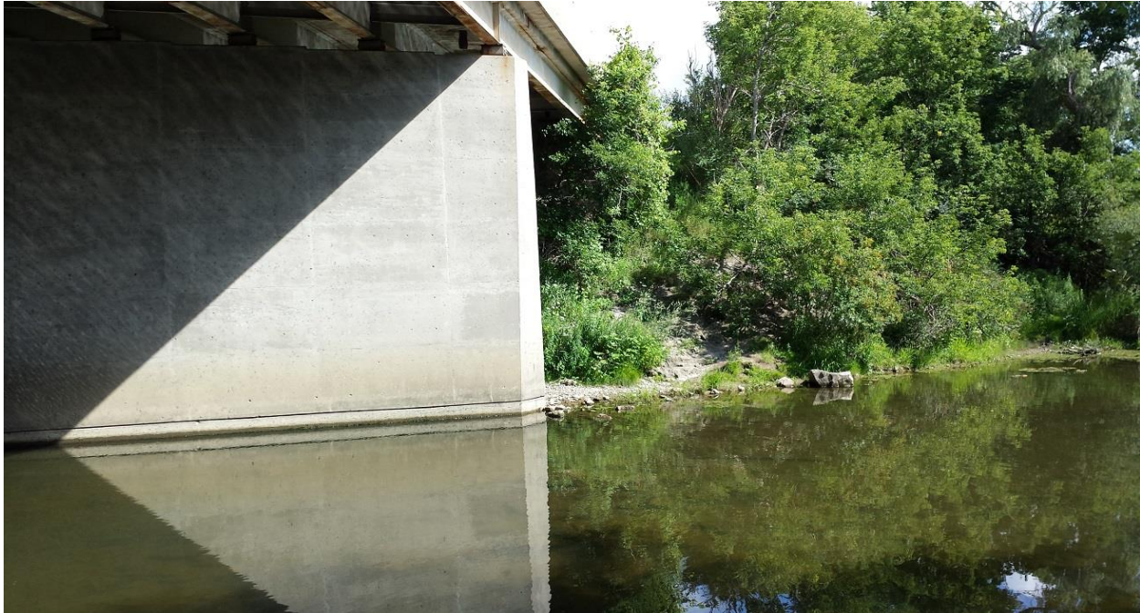
Photograph 9: Looking south from the west side of the bridge. The west slope adjacent to the south abutment was covered with bushes. Erosion of the slope face and scouring of the slope toe adjacent to the south abutment was observed. (July 24, 2014)
