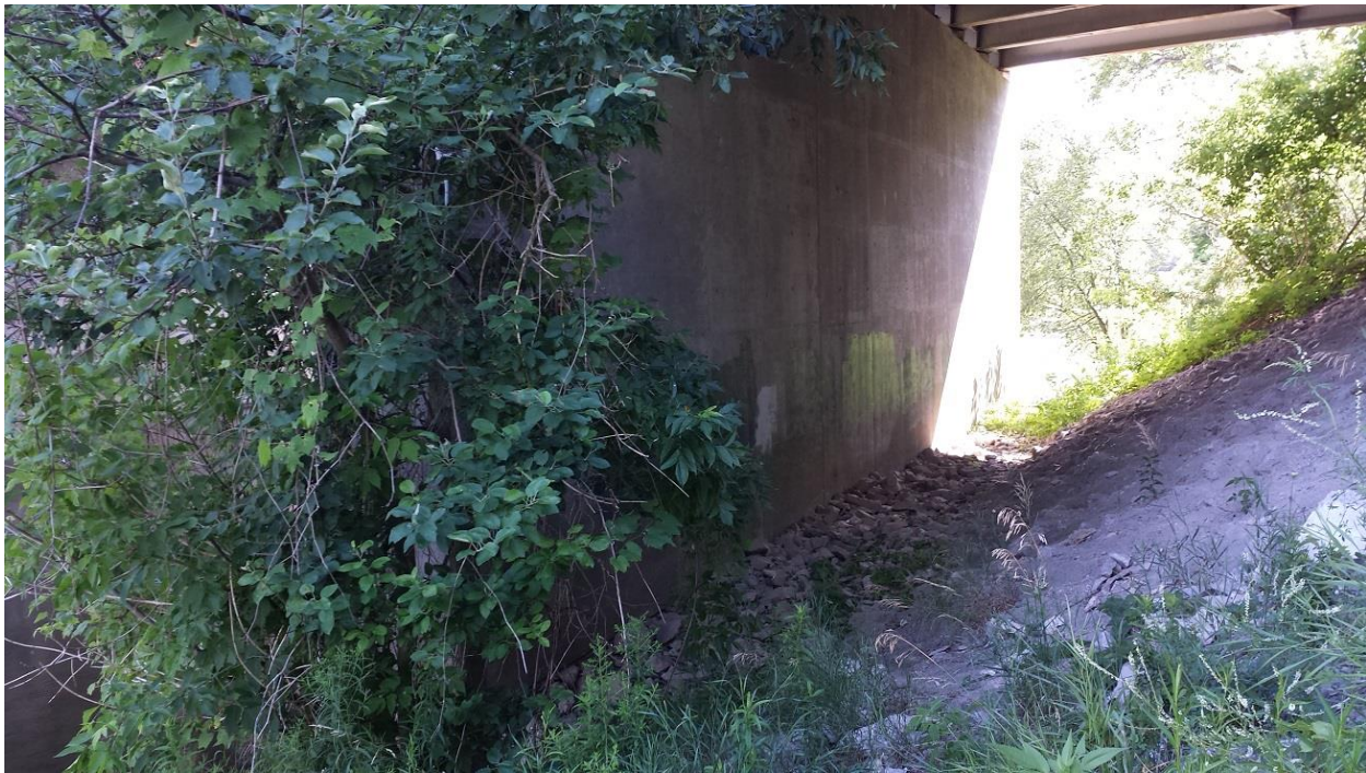
Photograph 11: Looking west at the north pier structure from the northeast corner. Rip-rap stones gathered at the bottom of the slope in front of the pier. No obvious cracks were observed on the pier. (July 24, 2014)
