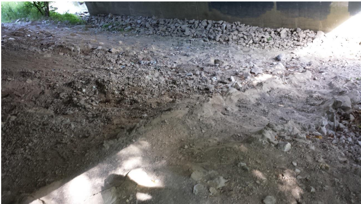
Photograph 8: Looking down at the slope face in front of the north abutment. Effects of erosion were observed on the slope face and the exposed earth in front of the north pier. The rip-rap stones gathered at the bottom of the slope probably due to erosion activity of the slope face. There were no obvious cracks on the pier wall. (July 24, 2014)
