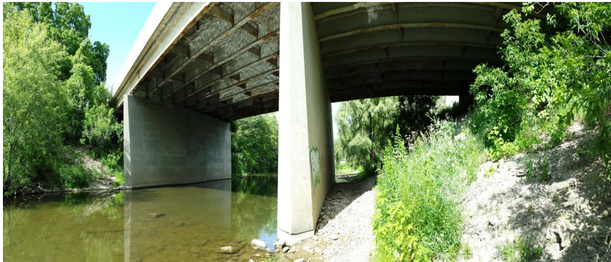
Photograph 6: Looking east at the bridge structure from the southwest corner. Erosion of exposed earth was evident on the slope face and adjacent to the south pier. (July 24, 2014)
