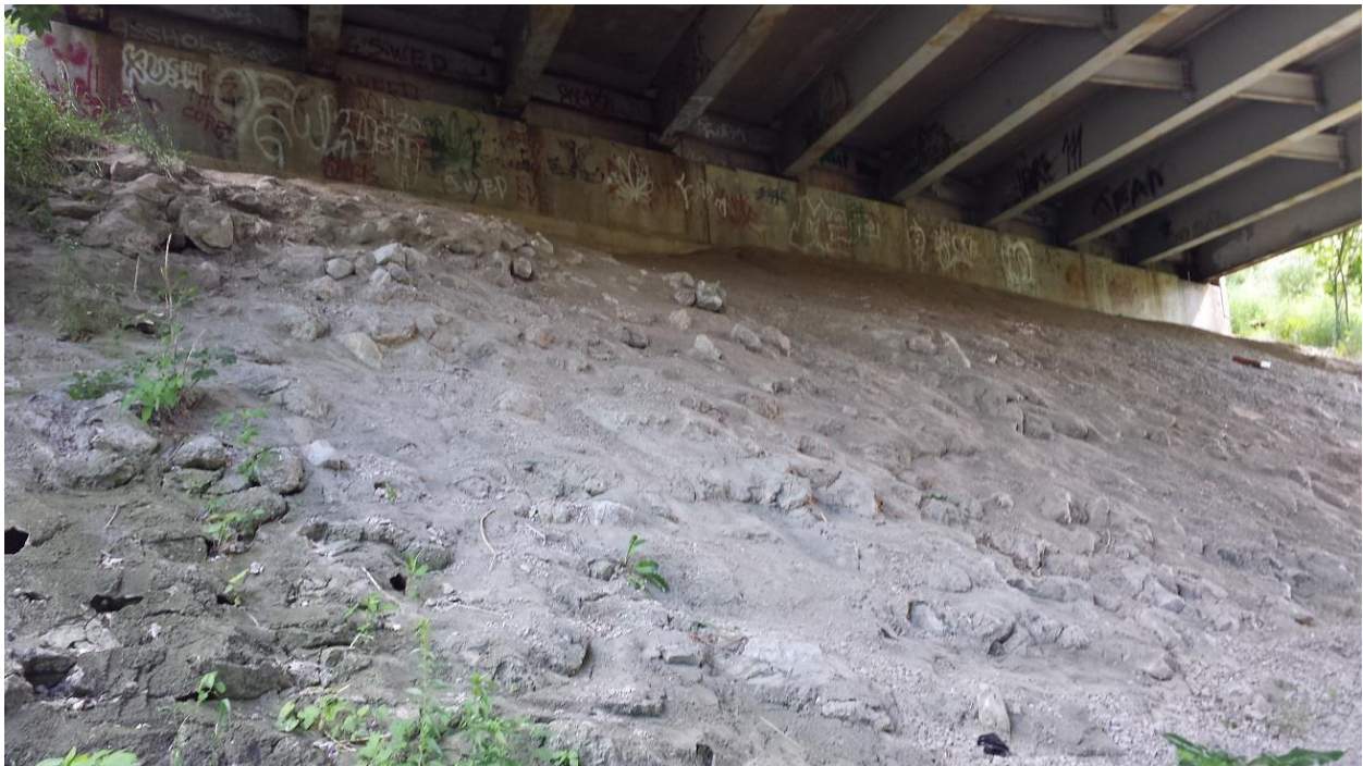
Photograph 4: Looking south at the slope face in front of the south abutment. Effects of erosion were observed on the slope face. (July 24, 2014)
