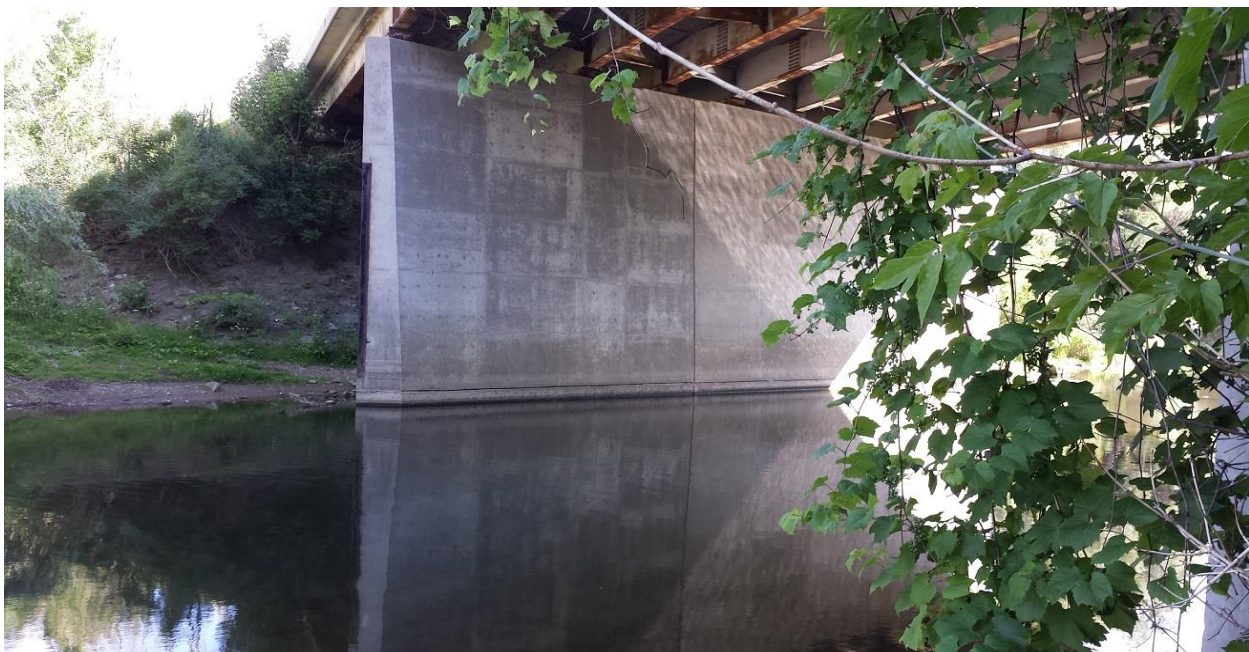
Photograph 12: Looking south from the east side of the bridge. The east slope adjacent to the south abutment was greatly affected by erosion activity. (July 24, 2014)
