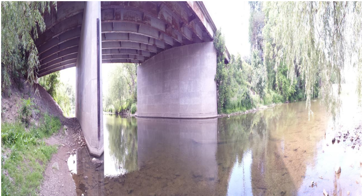
Photograph 1: Looking west at the bridge structure from the southeast corner. Slight erosion was observed on the slope face and the exposed earth adjacent to the south pier. (July 24, 2014)
