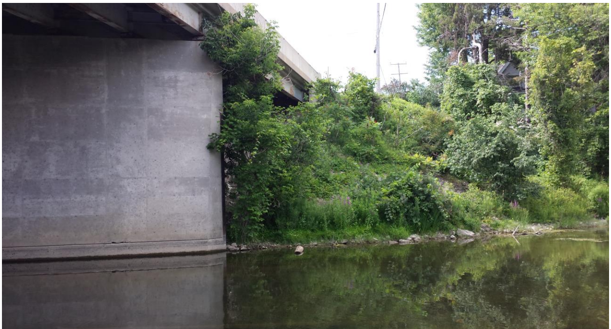
Photograph 2: Looking north from the east side of the bridge. The northeast slope was covered with bushes. Slight erosion of the slope face and scouring of the slope toe adjacent to the abutment was observed. (July 24, 2014)
