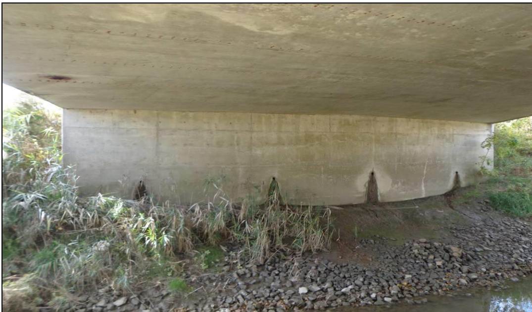
Photograph 4: Looking west at the west abutment wall from the east abutment. Weep holes in the abutment wall were observed to be open and wet. Scouring of the exposed earth was observed due to probable numerous fluctuated cycles of the water level over time. In addition, adequate rip-rap protection of the slope face was not observed and may need to be rehabilitated to protect the exposed ground from scouring effect. (October 20, 2013)
