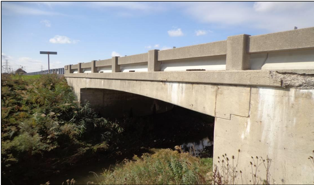
Photograph 1: Looking west at the adjacent south slope of the west abutment from the south slope of the east side of the bridge. The slope was heavily vegetated. No erosion or scouring was observed. (October 20, 2013).
