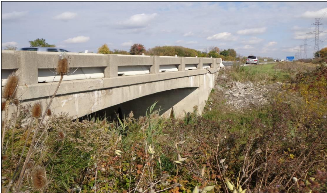
Photograph 3: Looking west at the south slope adjacent to the east abutment. A pile of debris was observed on the slope face. No erosion and scouring observed. (October 20, 2013)
