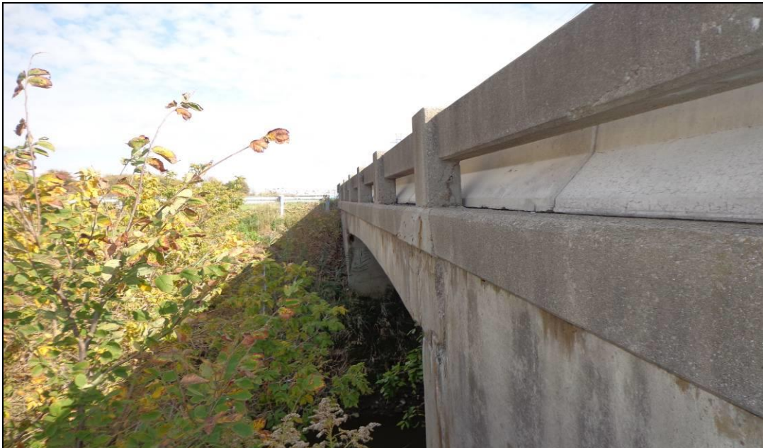
Photograph 2: Looking east at the north slope adjacent to the east abutment. Slope face was densely vegetated. No erosion or scouring was observed. (October 20, 2013)
