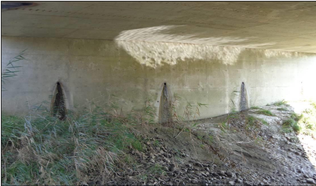
Photograph 5: Looking east from the north slope of the west side of the bridge towards the east abutment wall. Weep holes observed in the abutment wall were open and wet. Scouring of the exposed earth was observed most likely due to numerous fluctuated cycles of the water level over time. adequate rip-rap protection of the slope face was not observed and may need to rehabilitated to protect the exposed ground from scouring effect. (October 20, 2013)
