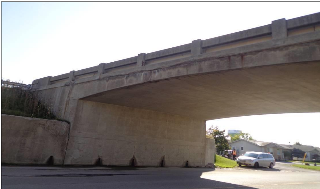
Photograph 2: Looking at the east abutment of the structure from northwest corner of the structure. The north and south slopes adjacent to the east abutment were vegetated with no signs of erosion. The slopes were retained with retaining wall structures. Weep holes were visible coming out the abutment and retaining walls. (October 20, 2013)
