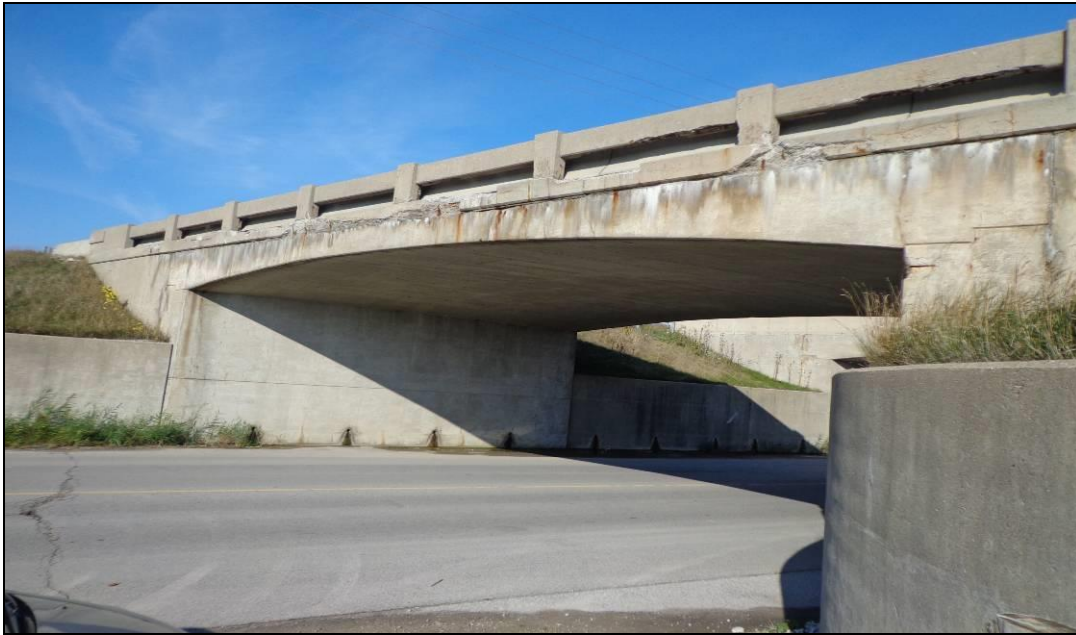
Photograph 3: Looking northwest at the west abutment wall of the structure from the southeast corner of the structure. The north and south slopes adjacent to the west abutment were vegetated with no signs of erosion. The slopes were retained with retaining wall structures. Weep holes were visible coming out the abutment and retaining walls. (October 20, 2013)
