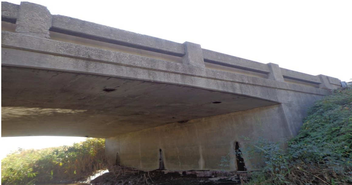
Photograph 4: Looking at the east abutment of the structure. The piling sheets driven were visible. The adjacent north slope of the abutment was vegetated and erosion of the slope face was not observed. (October 20, 2013)
