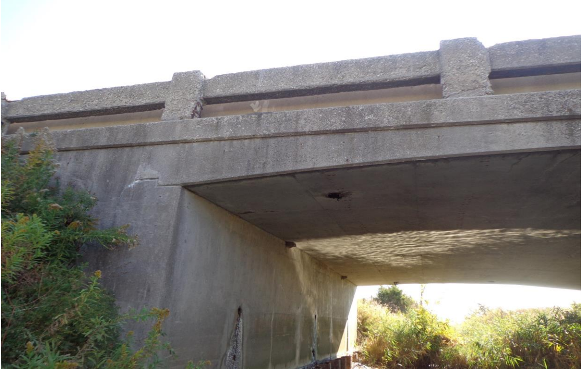
Photograph 5: Looking at the west abutment of the structure. The piling sheets driven were visible. The adjacent north slope of the abutment was vegetated and erosion of the slope face was not observed. (October 20, 2013)
