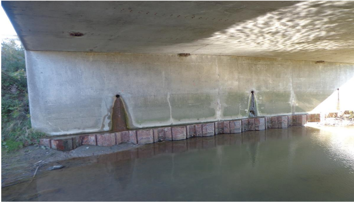
Photograph 3: Looking at the west abutment of the structure. The piling sheets driven were visible. The weep holes observed were open and wet. The exposed earth was affected by scouring. (October 20, 2013)
