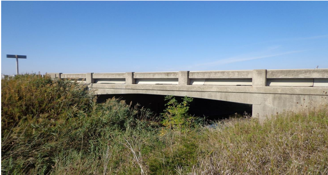
Photograph 1: Looking northwest at the McDougall Drain Bridge EBL from south side of the bridge. The two adjacent slopes flanking the drain on the south side of the bridge were heavily vegetated. No erosion of the slope faces was observed. (October 20, 2013)
