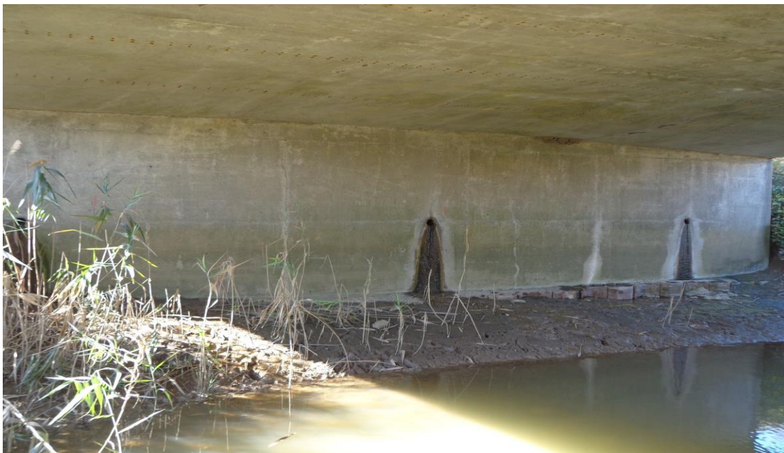
Photograph 2: Looking at the east abutment of the structure. The piling sheets driven were visible. The weep holes observed were open and wet. The exposed earth was affected by scouring. (October 20, 2013)
