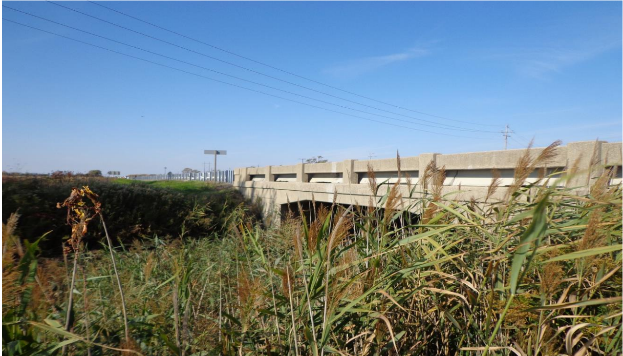
Photograph 1: Looking at the Little Baptiste Creek Bridge EBL structure from the southeast corner of the bridge. Vegetated slopes on either side of the banks were observed. Erosion of the slope faces was not observed. (October 20, 2013)
