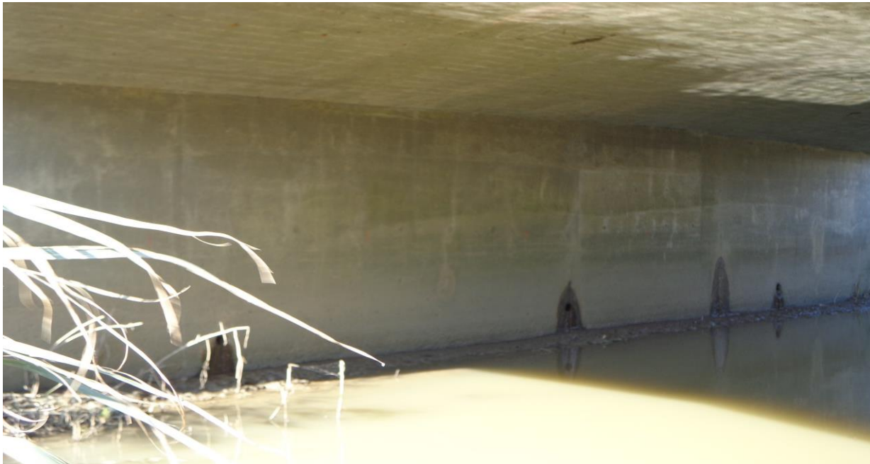
Photograph 3: Looking at the west abutment wall from the southeast corner of the structure. Scouring of the exposed earth was observed. Weep holes in the wall were open and wet. (October 20, 2013)
