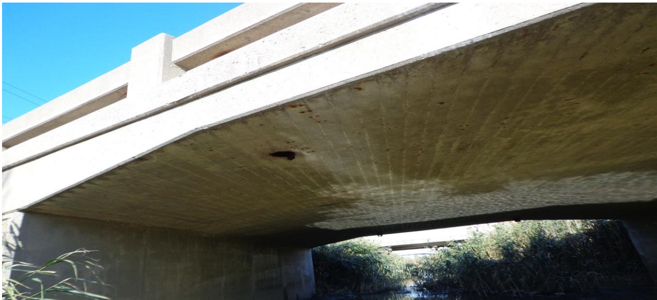
Photograph 2: Looking at the Little Baptiste Creek Bridge EBL structure from south of the bridge. The banks were heavily vegetated. No erosion of the slope faces was observed. (October 20, 2013)
