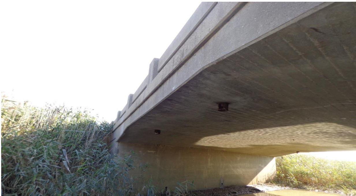
Photograph 4: Looking at the east abutment of the structure from the northwest corner of the structure. Scouring of the exposed earth in front of the abutment wall was observed. Weep holes in the wall were open. (October 20, 2013)
