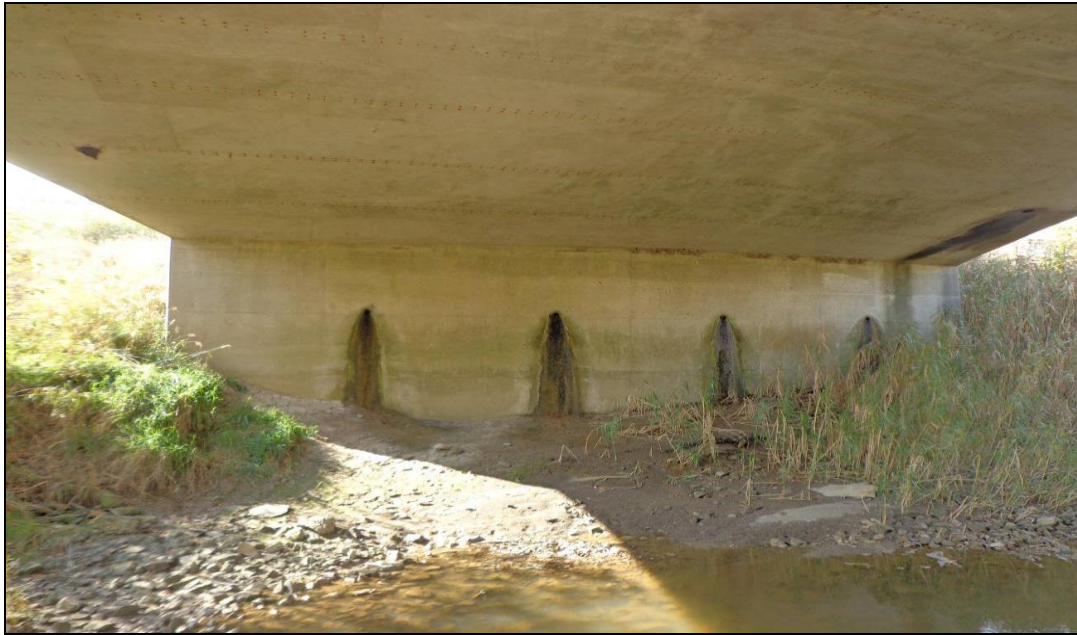
Photograph 3: Looking at the west abutment of the structure. Erosion/scouring effects were observed on the front slope and toe. Rock protection of the earth surface was minimum and scattered. Adjacent slopes of the abutment were vegetated. Weep holes in the abutment wall were open and wet. (October 20, 2013)
