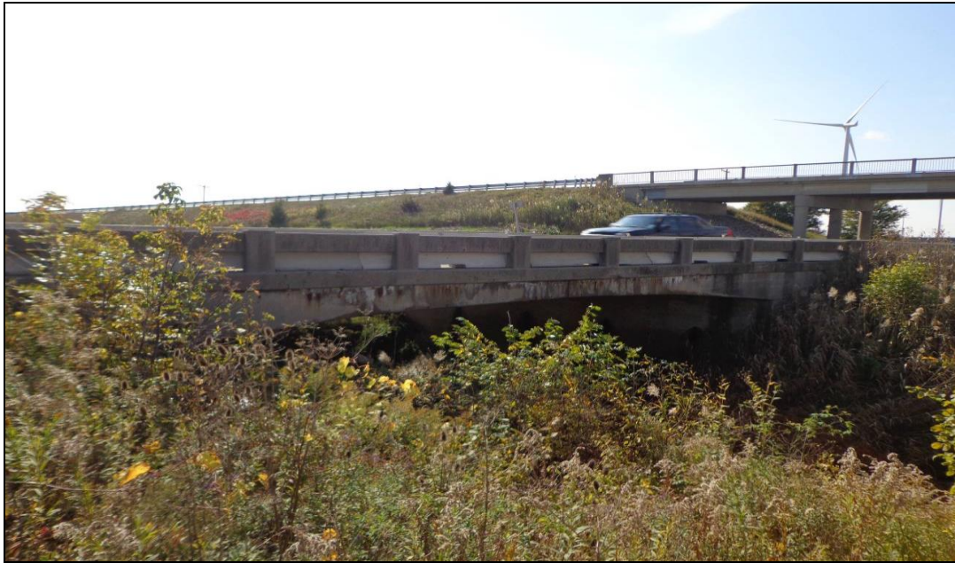
Photograph 1: Looking east at the Government Drain Bridge No. 3 EBL structure. The adjacent slopes of the abutments are heavily vegetated. No erosion of the slope face was observed. Scouring effects of the slope toes were not observed. (October 20, 2013)
