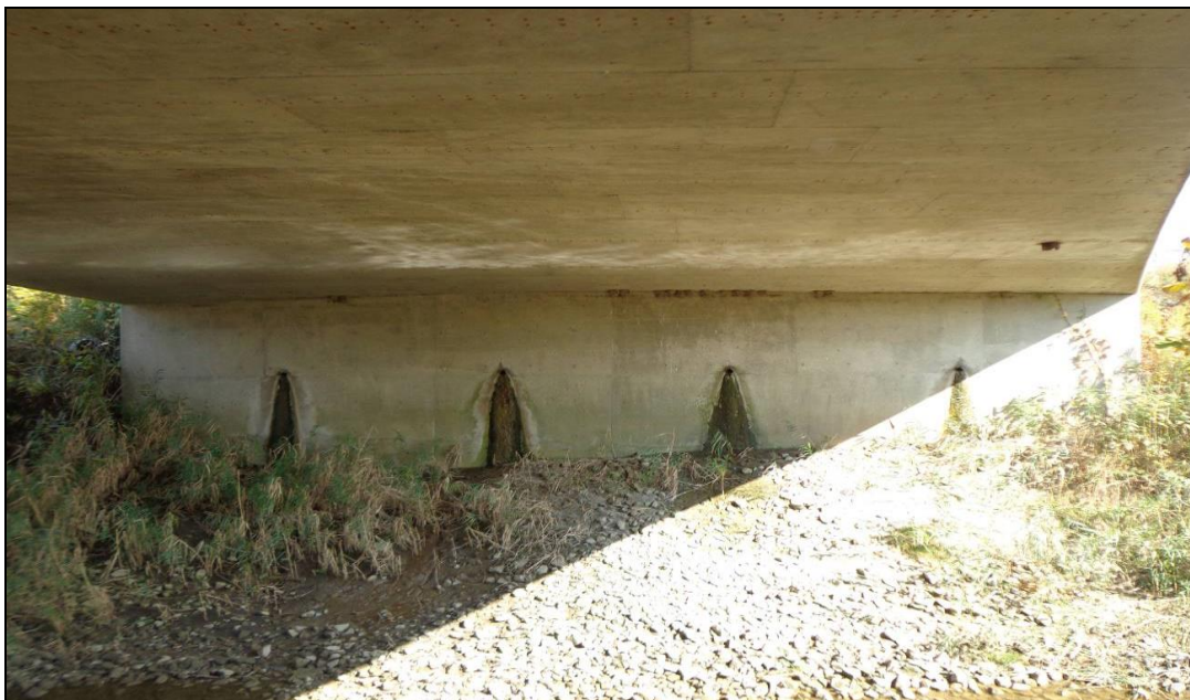
Photograph 2: Looking at the east abutment of the structure. Front slope partially covered with rip-rap. Slight erosion of the slope face or scouring of the toe of the exposed earth was observed on the front slope. Adjacent slopes of the abutment were vegetated. Weep holes in the abutment wall were open and wet. (October 20, 2013)
