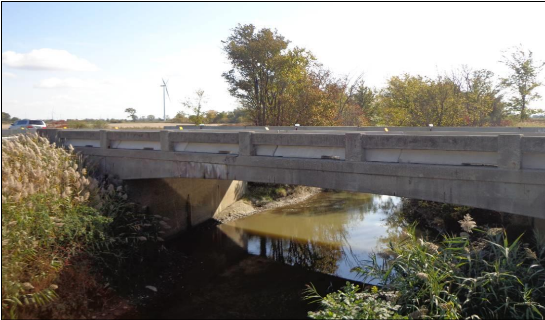
Photograph 1: Looking south at the Government Drain Bridge #2 EBL structure from the median of Highway 401. Both adjacent slopes were observed to be densely vegetated. Erosion of the slope faces was not observed. (October 20, 2013)
