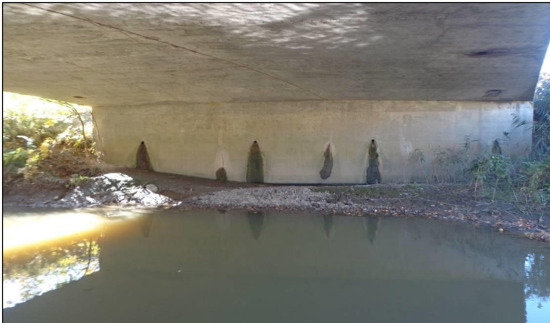
Photograph 3: Looking at the west abutment wall of the bridge structure from the east abutment wall. Scouring/erosion of the exposed earth were observed. Weep holes in the abutment wall were open and wet. (October 20, 2013)
