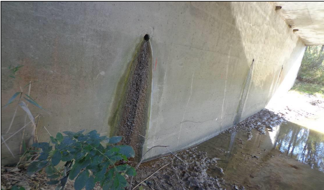
Photograph 2: Looking south at the east abutment wall of the bridge structure. Scouring of the exposed earth was observed. Weep holes in the abutment wall were open and wet. (October 20, 2013)
