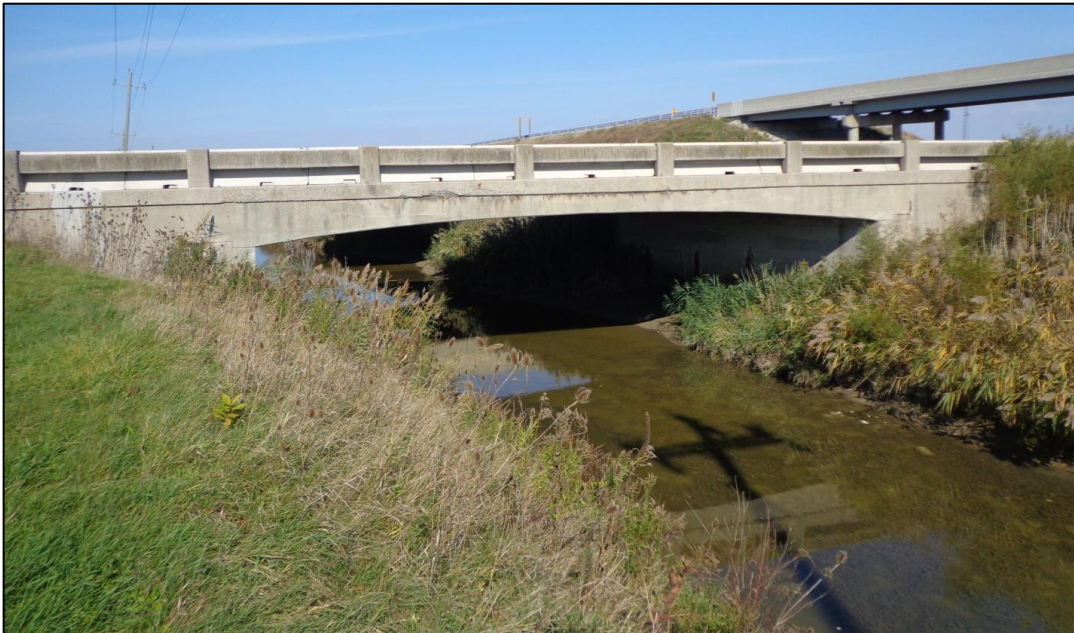
Photograph 1: Looking north at the Government Drain Bridge #1 EBL Structure from the south bank. The north and south slopes adjacent to the structure were densely vegetated. No scouring and erosion were observed. (October 20, 2013)
