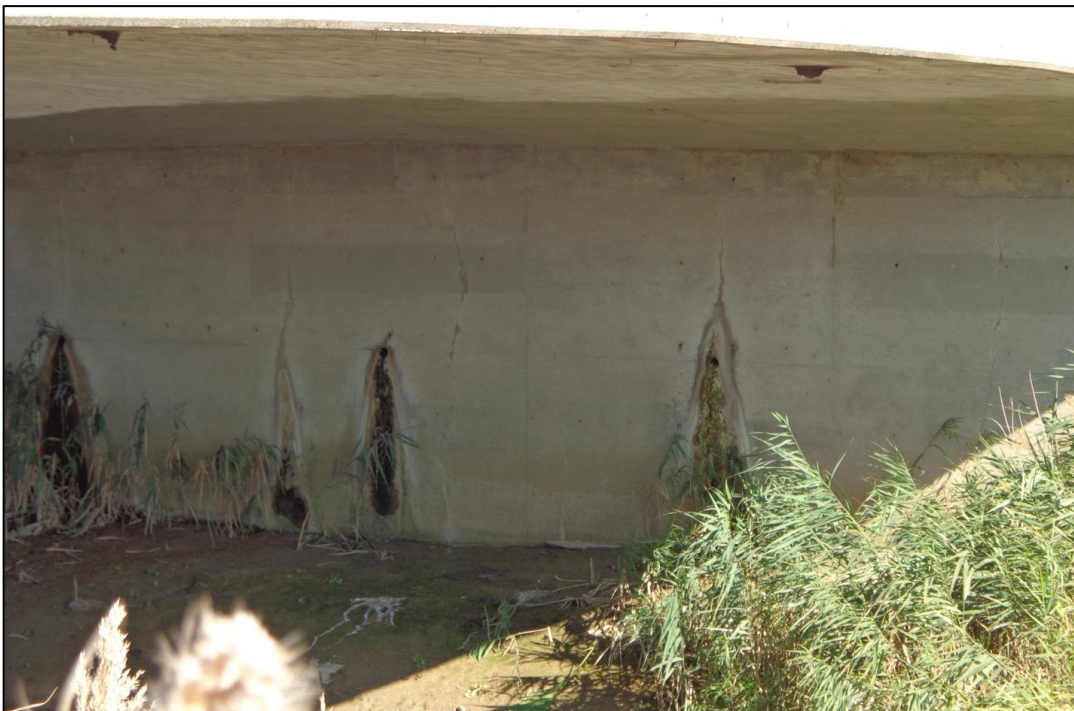
Photograph 2: Looking at east abutment of the structure from the adjacent south slope of the west abutment. Concrete surface deterioration including concrete spalls and cracks were observed. It was noticed that very few vegetation was growing in front of the abutment. Slight scouring effect of the exposed earth was observed at the abutment wall. No rock protection was observed. (October 20, 2013)
