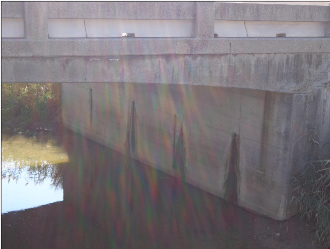
Photograph 3: Looking at west abutment of the structure from the adjacent north slope of the east abutment. Slight scouring effect was observed at the abutment wall location. No rock protection was observed. Water was at about 0.1 m deep close to the abutment wall. (October 20, 2013)
