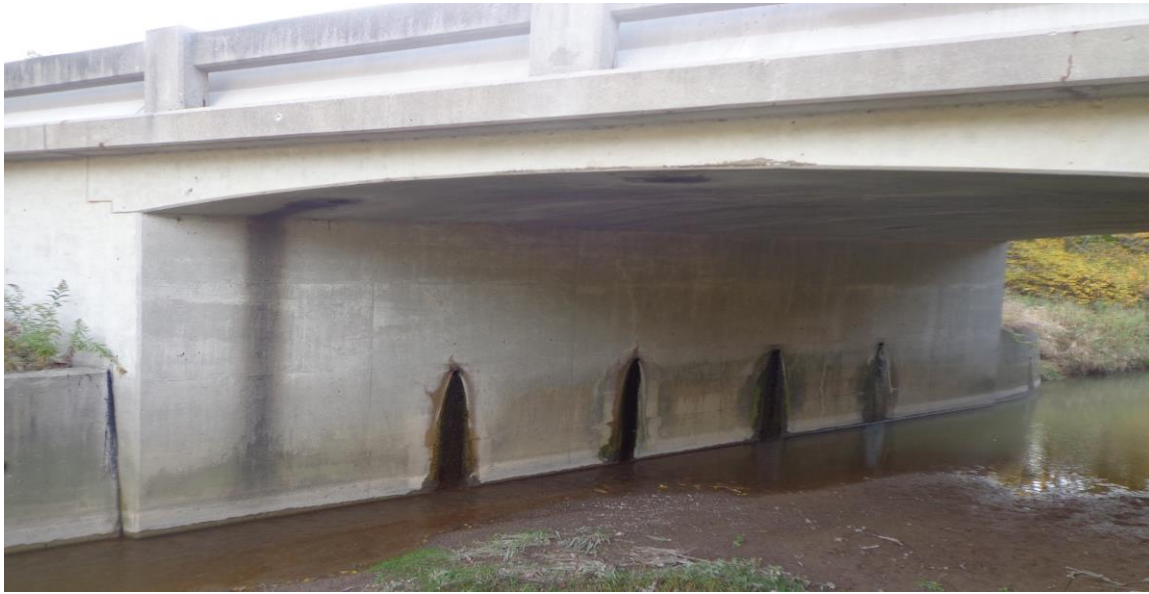
Photograph 3: Viewing east from the west side of the Fleming Creek Bridge EBL structure at the east abutment wall. Surficial cracks were observed on the abutment wall. Scouring effect of the exposed ground was evident. The weep holes in the abutment and retaining walls were open and wet. (October 20, 2013)
