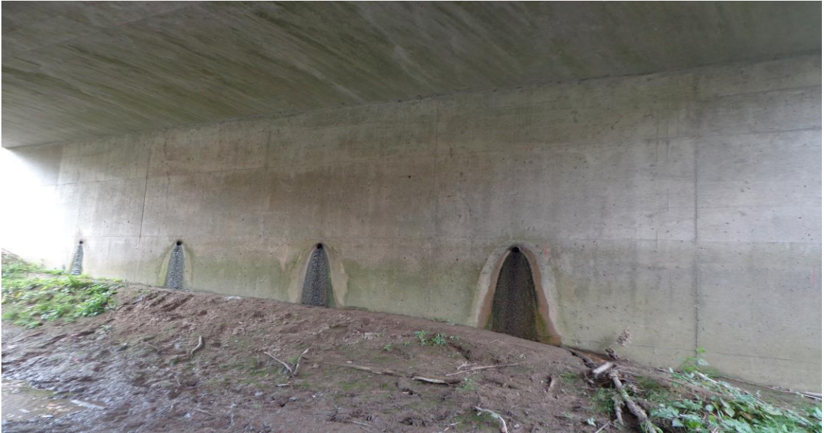
Photograph 5: Viewing west from the east side of the Fleming Creek Bridge EBL structure at the west abutment wall. Slight scouring of the exposed ground was evident. The weep holes in the abutment and retaining walls were open and wet. (October 20, 2013)
