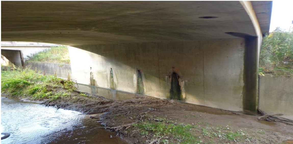
Photograph 4: Viewing west from the east side of the Fleming Creek Bridge WBL structure at the west abutment wall. Surficial cracks were observed on the abutment wall. Scouring of the exposed ground was evident. The weep holes in the abutment and retaining walls were open and wet. (October 20, 2013)
