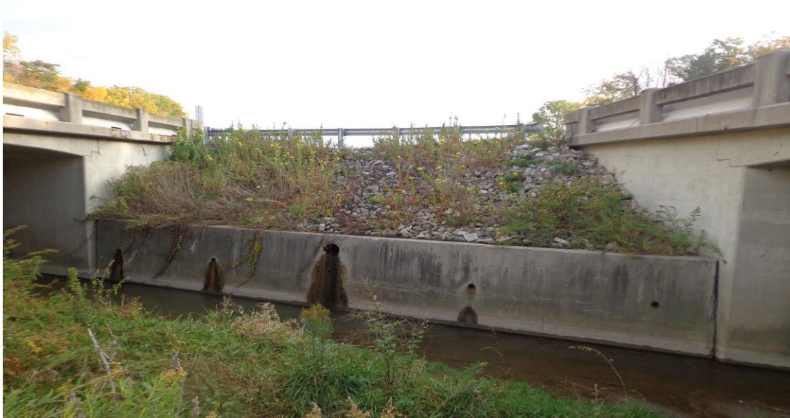
Photograph 2: Viewing east from the west side of the Fleming Creek Bridge WBL structure at the east median retaining wall structure. Partial vegetation and some rock protection on the slope ground were observed. The weep holes in the retaining walls were open and wet. (October 20, 2013)
