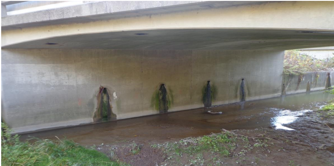
Photograph 1: Viewing east from the west side of the Fleming Creek Bridge WBL structure at the east abutment wall. Scouring effect of the exposed ground was evident. The weep holes in the abutment and retaining walls were open and wet. (October 20, 2013)
