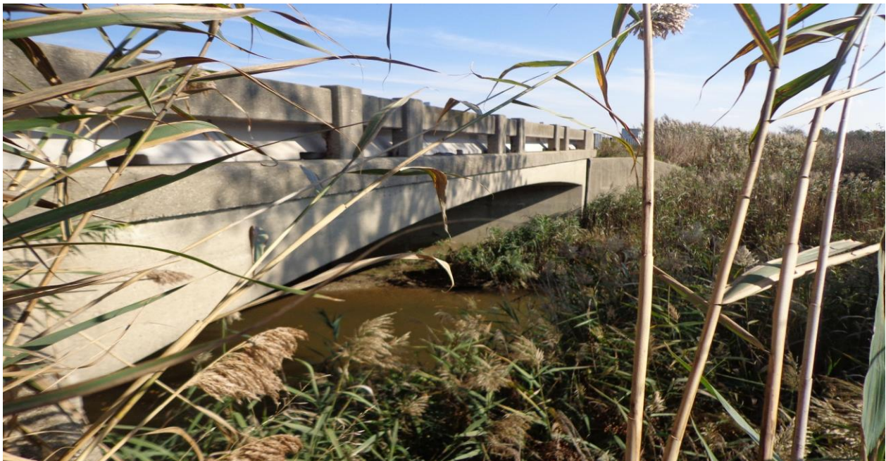
Photograph 2: Looking at east abutment and retaining walls of the structure. The adjacent slopes were heavily vegetated. Scouring of the exposed earth in front of the abutment was observed. (October 20, 2013)
