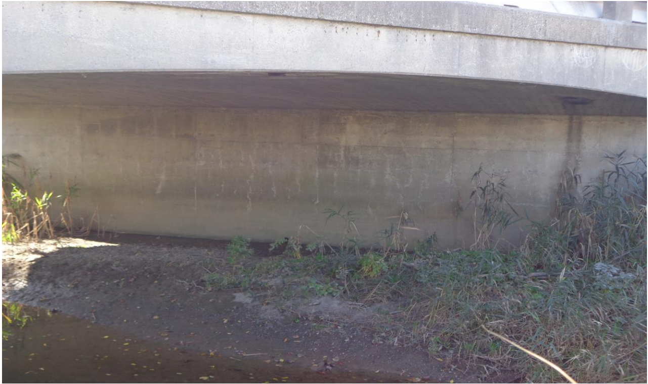
Photograph 3: Looking at west abutment of the structure. Slight scouring of the exposed earth was observed. The weep holes in the wall were open and dry. Water was at about 0.3 m depth at the abutment location.
