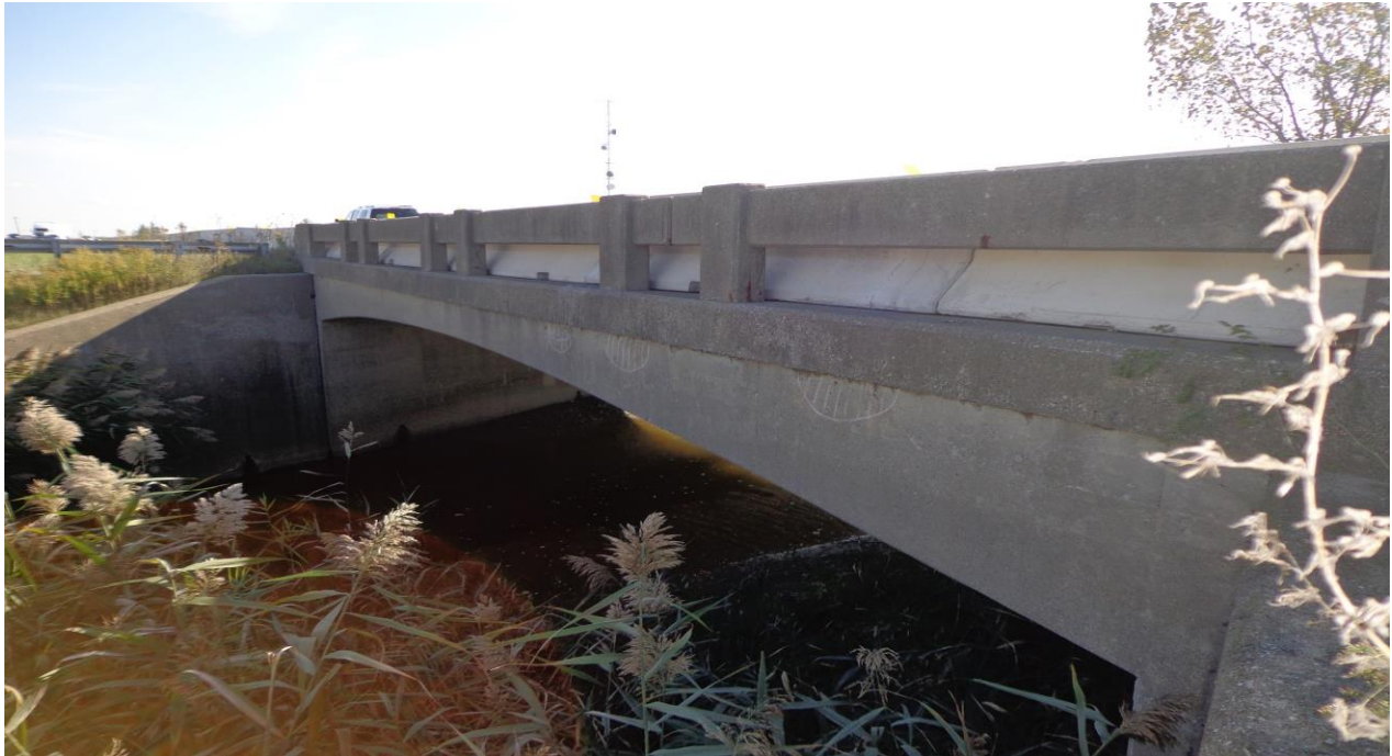
Photograph 1: Looking east at the east abutment and retaining walls from the west side of the Baptiste Creek Bridge EBL. Scouring of the exposed earth in front of the abutment wall was observed. The weep holes in the walls were open and wet. (October 20, 2013)
