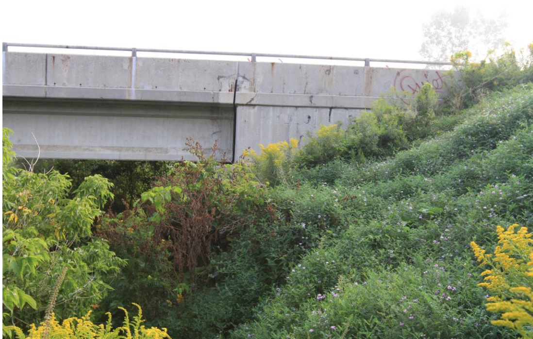
Photograph 2: Westbound Lane, West Abutment. Abutment side slopes are grass covered and no obvious signs of erosion observed on abutment side slopes (September 2, 2015).
