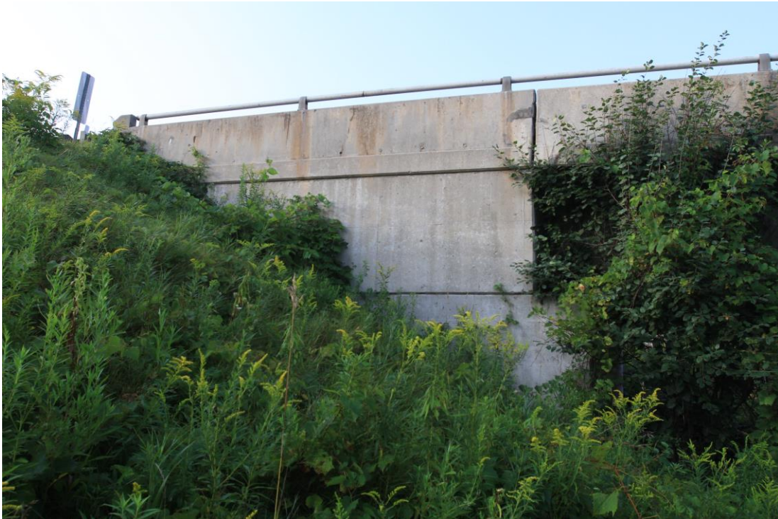
Photograph 1: Westbound Lane, East Abutment and North Wingwall. Abutment slopes are grass covered and no obvious signs of erosion observed on slope (September 2, 2015).
