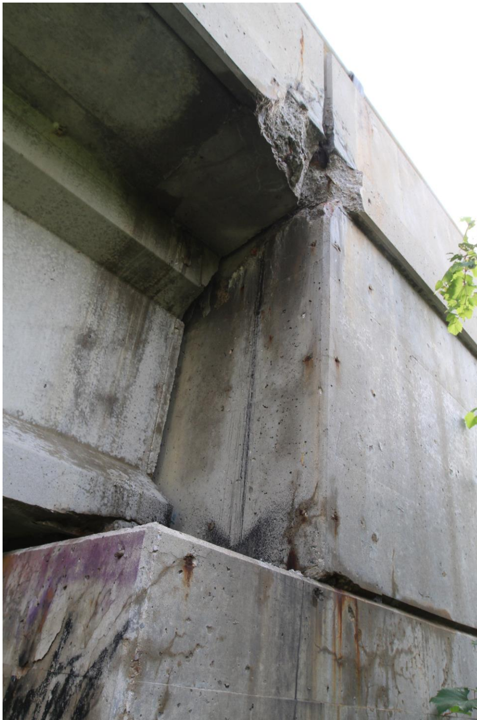
Photograph 6: Eastbound Lane, East Abutment and South Wingwall. Spalling of Bridge Deck Concrete observed (September 2, 2015).
