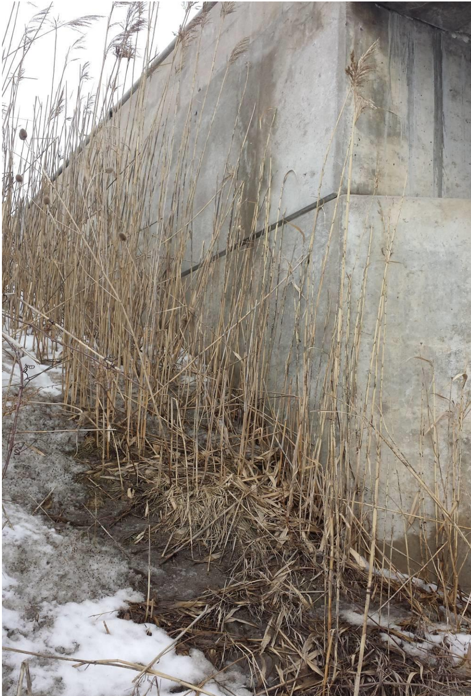
Photograph 4: Looking northwest at the south wingwall of the west abutment of the WBL structure. Slope covered with ice and snow. Surficial cracks were observed on the wall. (February 19, 2014)
