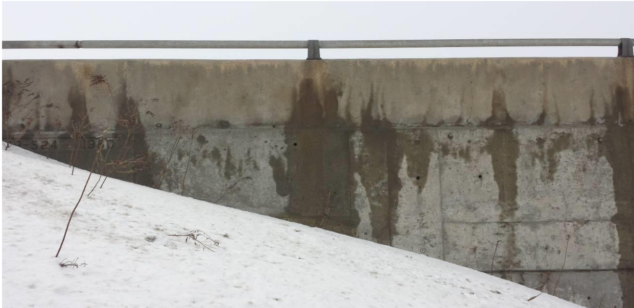
Photograph 1: Viewing south at the north wingwall of the east abutment of the WBL structure. Slope covered with snow and thus, no erosion or scour was observed on slope. No obvious major cracks were observed on the wall. (February 19, 2014)
