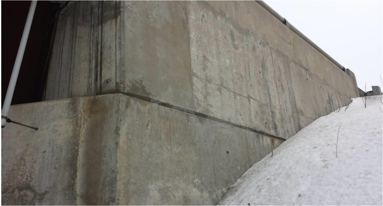
Photograph 3: Viewing north at the south wingwall of east abutment of WBL structure. Slope covered with snow and thus, no erosion was observed on the slope. Surficial cracks were observed on the wall. (February 19, 2014)
