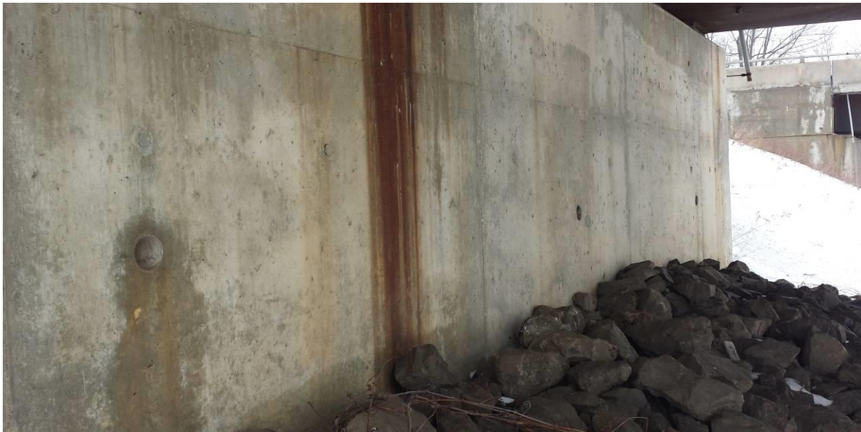
Photograph 2: Looking at the east abutment wall of the WBL structure. The front slope of the abutment wall was covered with rock protection in non-uniform distribution. Surficial cracks observed on abutment wall. Weeping holes observed in the abutment wall. (February 19, 2014)
