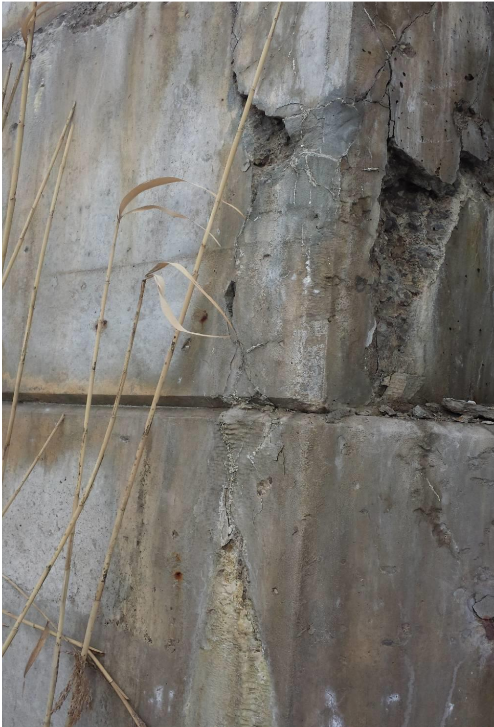
Photograph 13: Looking at the southwest corner of the west abutment of the EBL structure. Major concrete spalling with concrete deterioration was observed. (February 19, 2014)
