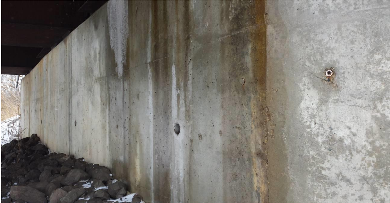
Photograph 10: Viewing south at the west abutment wall of the EBL structure. Concrete spalling was observed on the wall with minor cracks. The front slope of the abutment wall was covered with rock protection in non-uniform distribution. (February 19, 2014)
