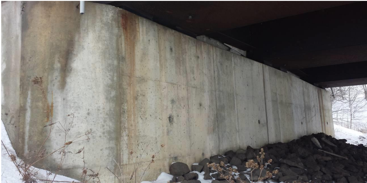
Photograph 7: Looking at the east abutment wall of the EBL structure. The front slope of the abutment wall was covered with stones in non-uniform distribution. Surficial cracks observed on abutment wall. Weeping hole observed in abutment wall. (February 19, 2014)
