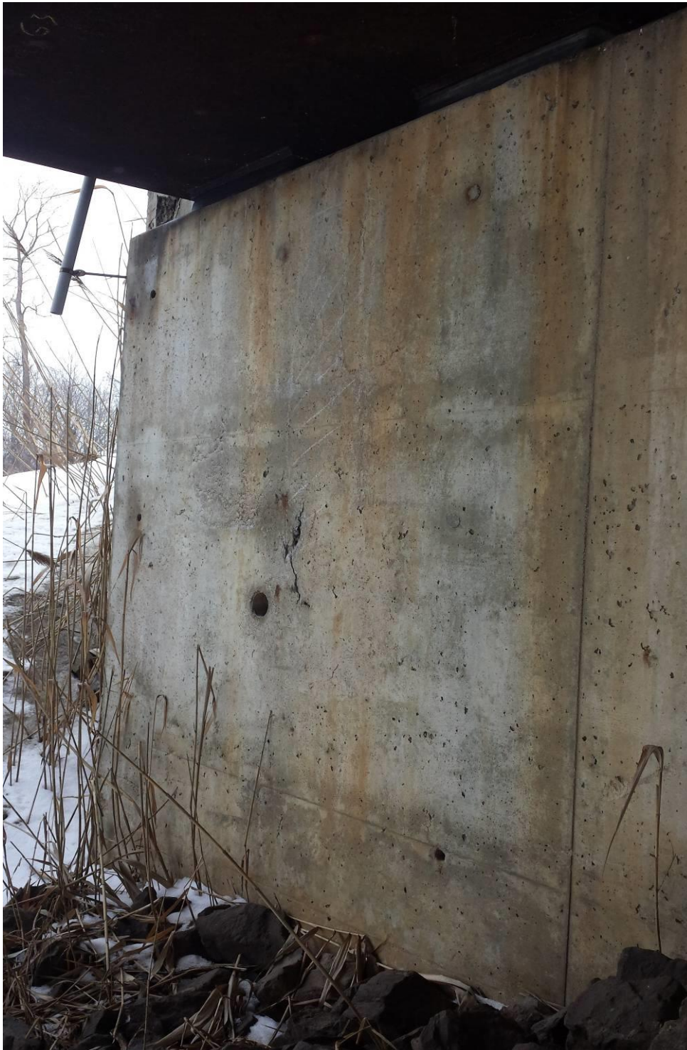
Photograph 11: Viewing the south end of the west abutment wall of the EBL structure. Concrete spalling with associated pop outs were observed on the abutment wall. (February 19, 2014)
