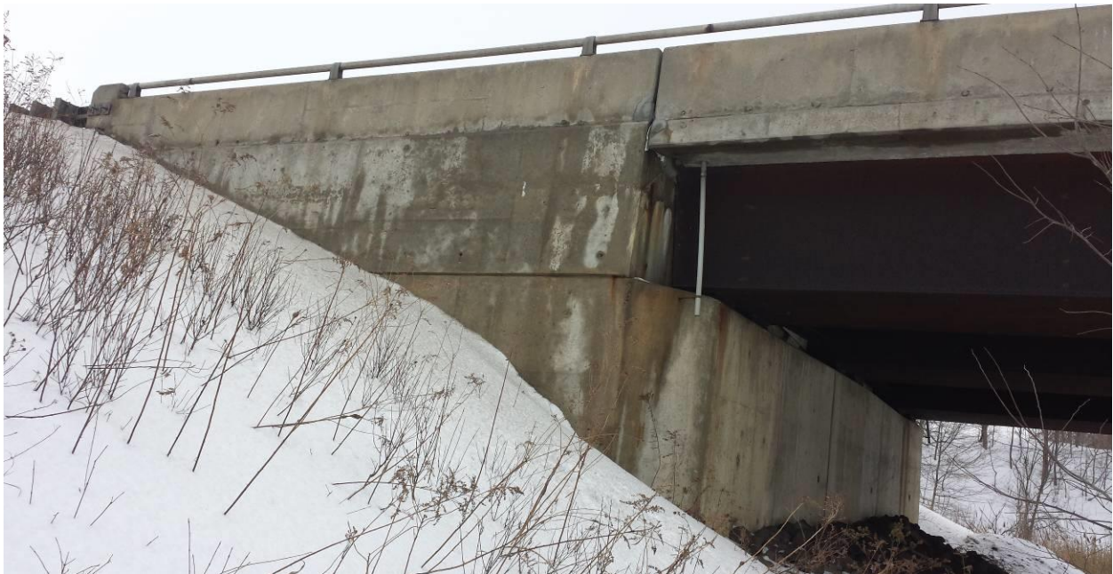
Photograph 6: Viewing south at the north wingwall of east abutment of EBL structure. Minor concrete scaling was observed on wingwall. No erosion was observed on slope. No obvious major cracks were observed, except for map cracks. Minor spalling was observed on the wall. (February 19, 2014)
