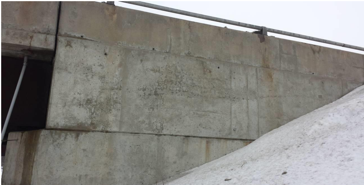
Photograph 8: Viewing north at the south wingwall of the east abutment of the EBL structure. Minor concrete scaling was observed on the wingwall. No erosion was observed on slope due to snow covering. Surficial cracks and slight spalling were observed on the wall. (February 19, 2014)
