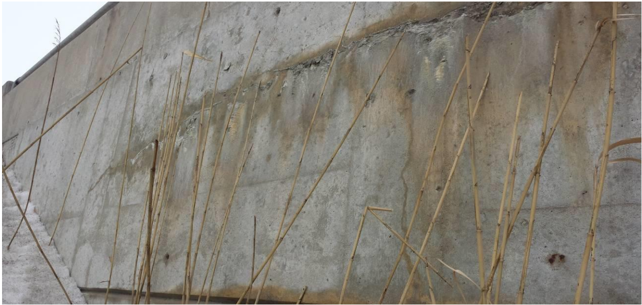
Photograph 12: Viewing northwest at the south wingwall of the west abutment of the EBL structure. A major horizontal crack was observed on the wingwall with concrete spalling. (February 19, 2014)
