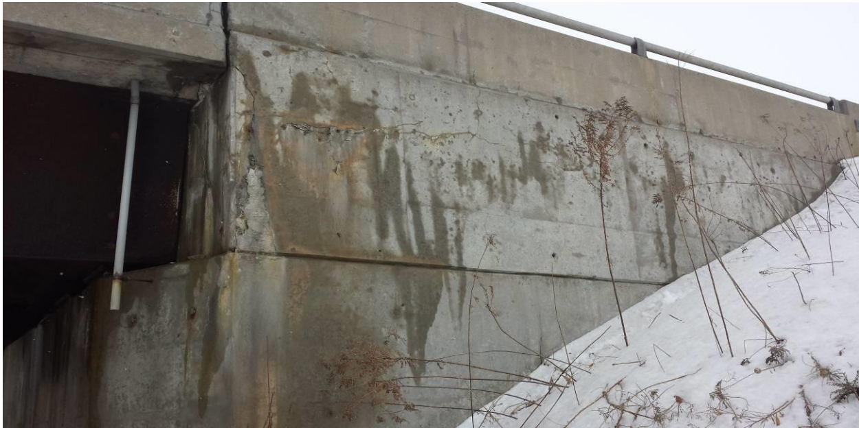
Photograph 9: Viewing south at the north wingwall of the west abutment of the EBL structure. A major horizontal crack with concrete spalling was observed on the wingwall. The slope was covered with snow and thus, no erosion was observed of the slope. (February 19, 2014)
