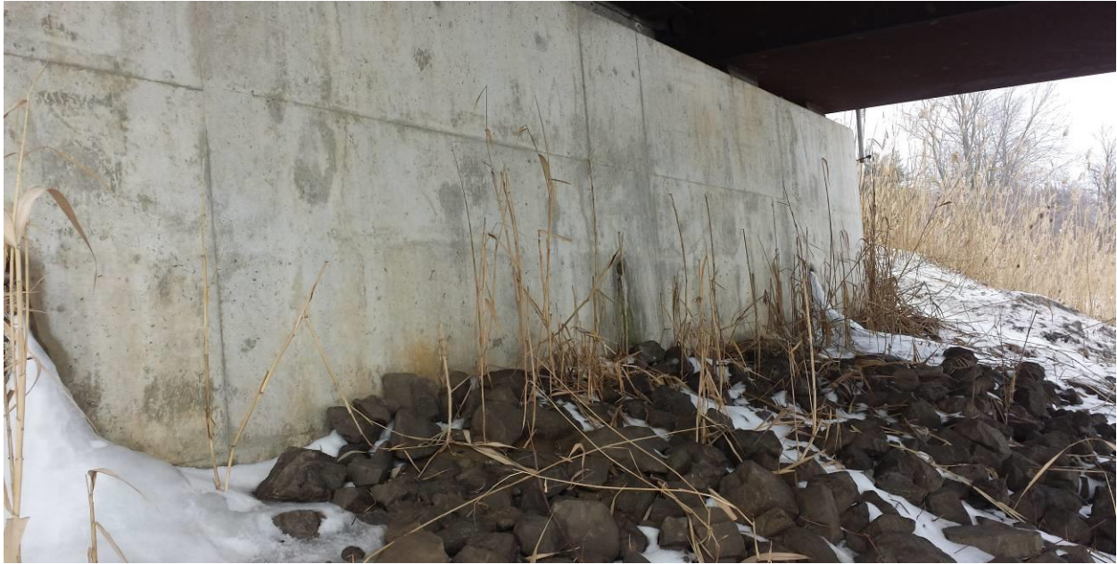
Photograph 5: Looking at the west abutment wall of the WBL structure. The front slope of the abutment wall was covered with rock protection in non-uniform distribution. Surficial cracks were observed on the abutment wall. Weeping holes were observed in the abutment wall. (February 19, 2014)
