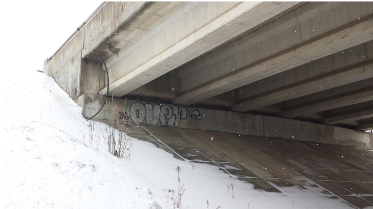
Photograph 9: Looking at north wingwall of the east abutment of WBL structures; no obvious major cracks observed except for surficial cracks. Adjacent slope covered with snow and few withered grasses. (February 19, 2014)
