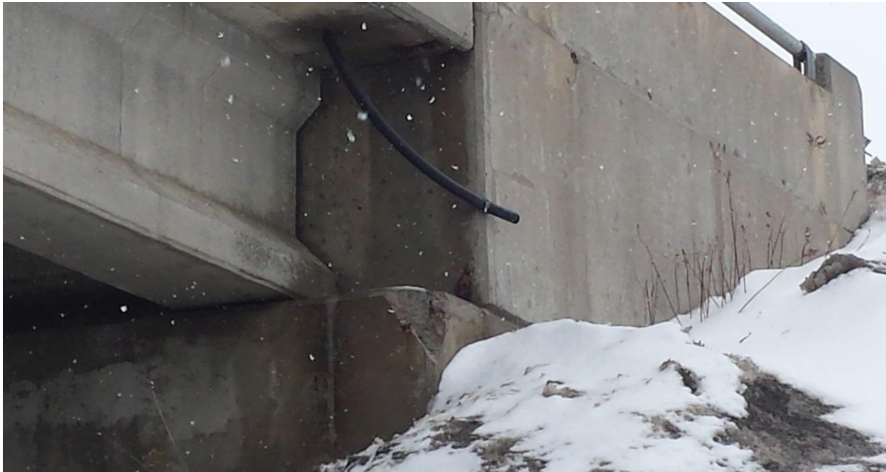
Photograph 12: Looking at south wingwall of the east abutment of EBL structure. Corner concrete damage of the wall was observed. Otherwise no obvious major cracks were observed except for surficial cracks. Adjacent slope covered with snow. (February 19, 2014)
