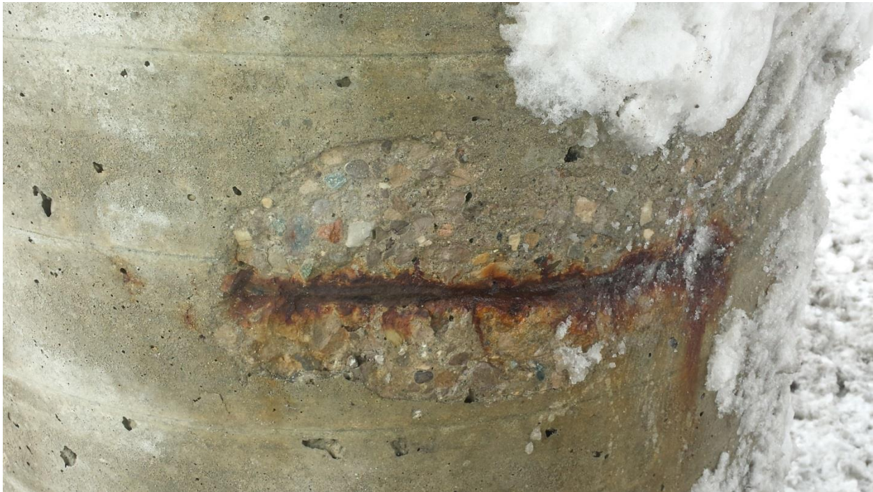
Photograph 14: Concrete deterioration exposed the reinforcement of piers.
