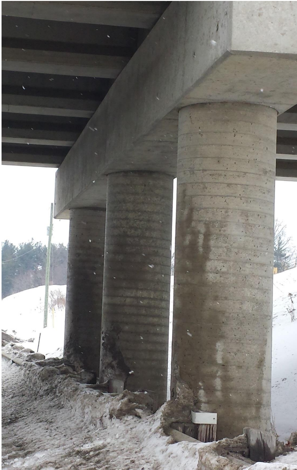
Photograph 13: Looking at the piers of the west abutment of EBL structure. Concrete cracks, spalling and deterioration were observed on the surfaces of the piers. (February 19, 2014)
