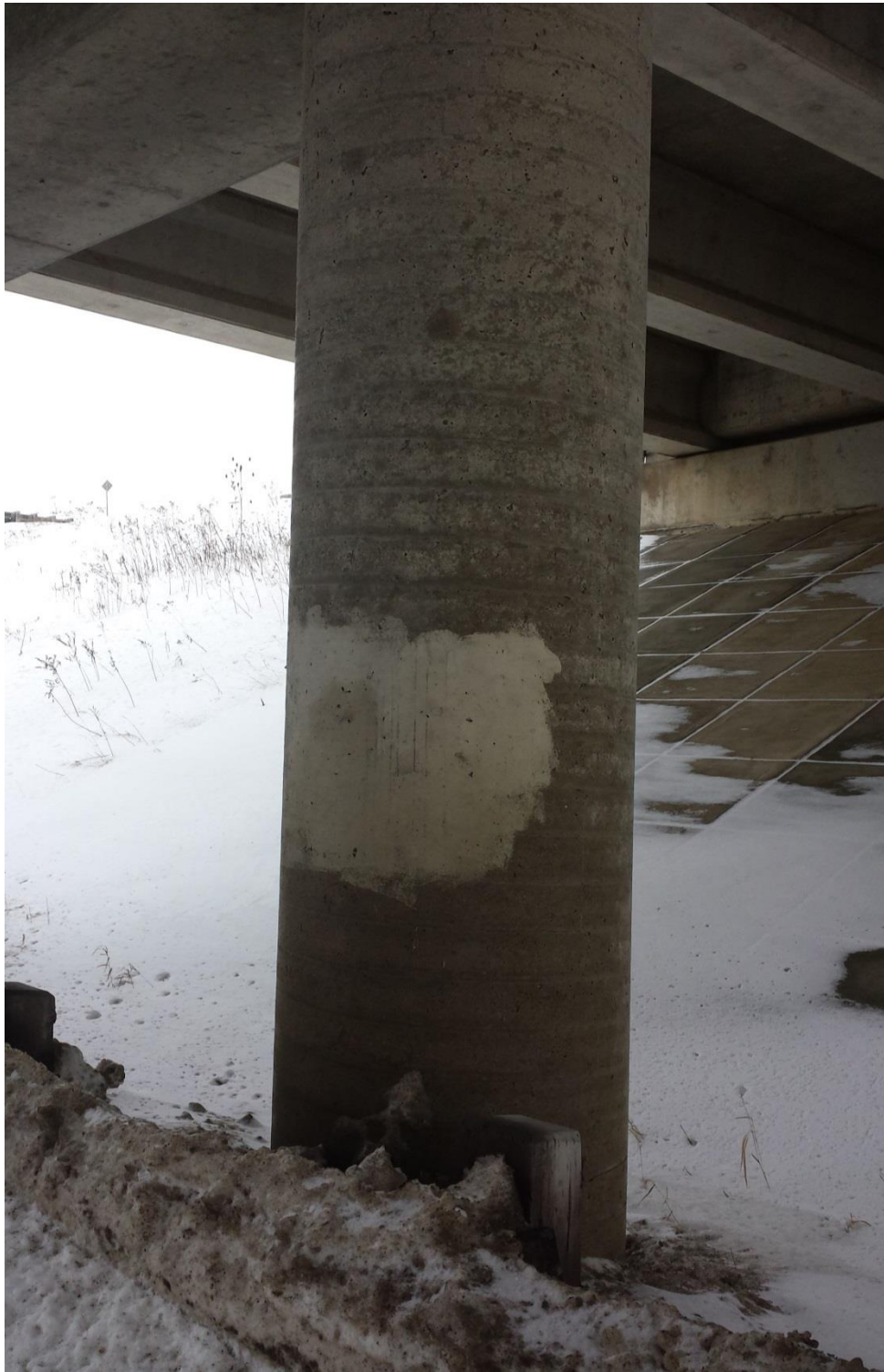
Photograph 16: Looking at a pier of the east abutment of WBL structure. Surface rehabilitation was performed on the pier surface. (February 19, 2014)
