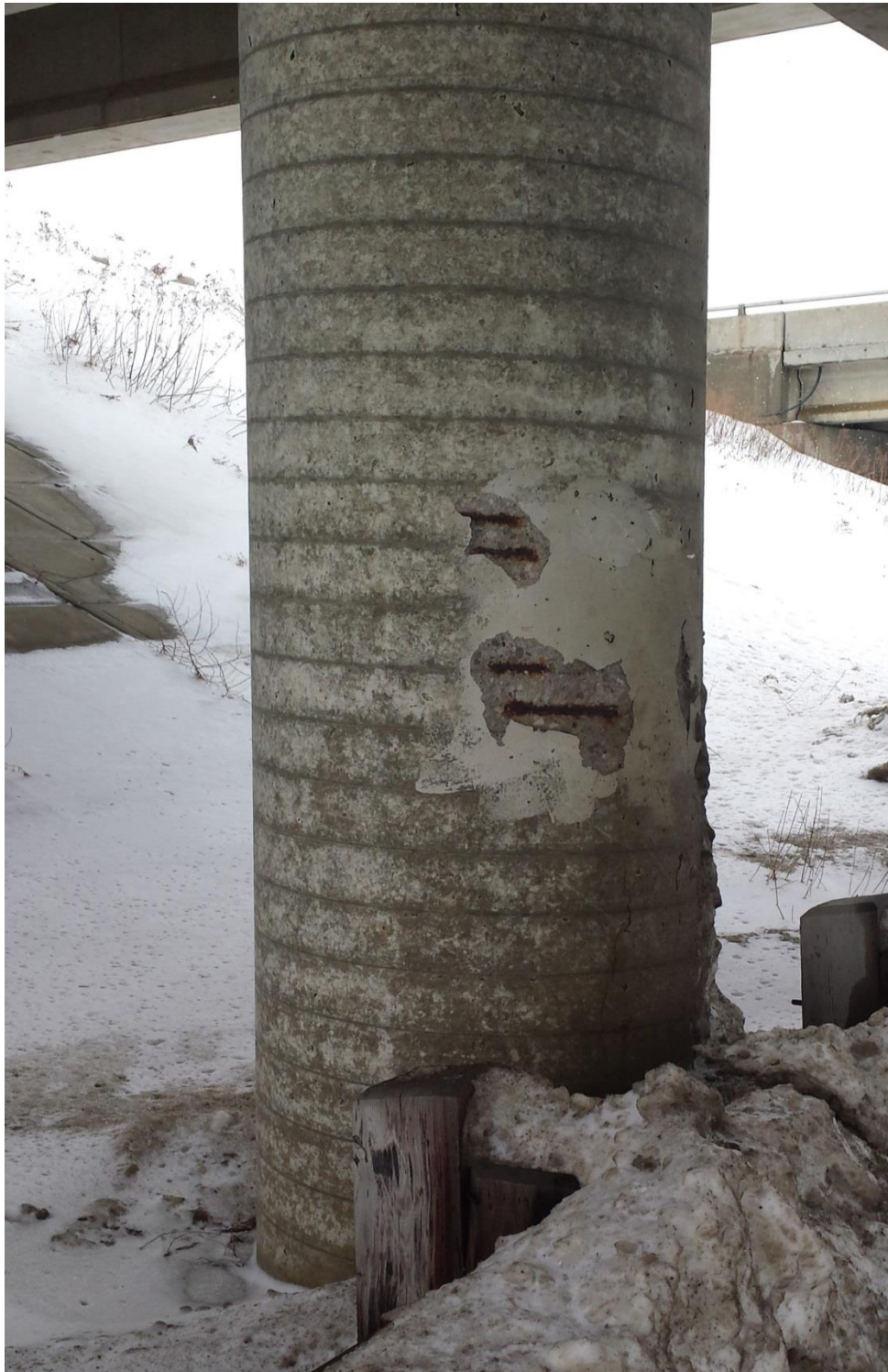
Photograph 15: Looking at a pier of the east abutment of EBL structure. Concrete cracks, spalling and deterioration were observed on the pier surface. Rehabilitation was performed on the pier surface, however, deterioration progressed exposing the rebars. (February 19, 2014)
