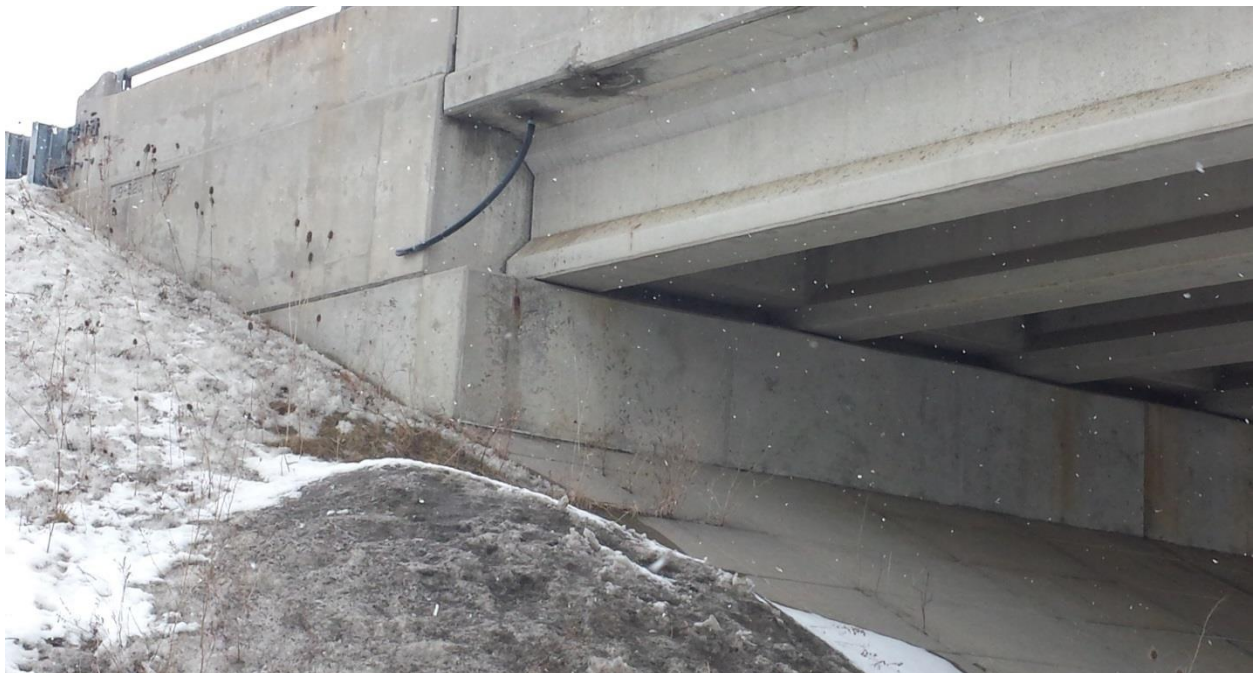
Photograph 2: Looking at south wingwall of the west abutment of EBL structure. No obvious major cracks observed except for surficial longitudinal cracks. No erosion could be observed on adjacent slope due to snow cover. (February 19, 2014)
