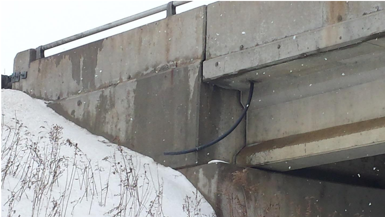
Photograph 11: Looking at north wingwall of the east abutment of EBL structure; no obvious major cracks observed except for surficial cracks. Adjacent slope covered with snow and few withered grasses.
