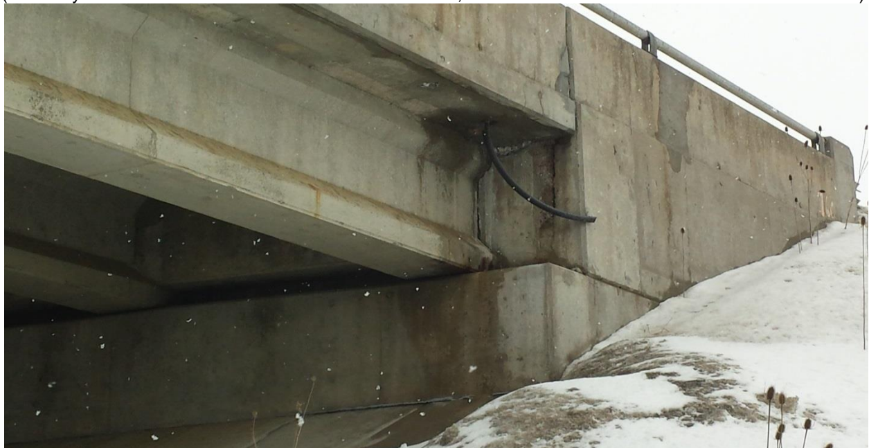
Photograph 10: Looking at south wingwall of the east abutment of WBL structure; no obvious major cracks observed except for surficial cracks. Slope covered with snow. (February 19, 2014)
