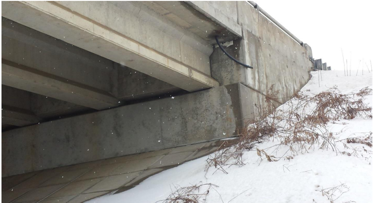
Photograph 5: Looking at north wingwall of the west abutment of EBL structure, no obvious major cracks observed except for surficial cracks. Adjacent slope covered with snow. (February 19, 2014)
