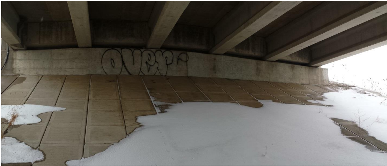
Photograph 7: Looking at west abutment wall of WBL structure. Front slope covered with concrete, no obvious major cracks observed except map cracking. No weeping hole or outlet system observed on abutment. (February 19, 2014)
