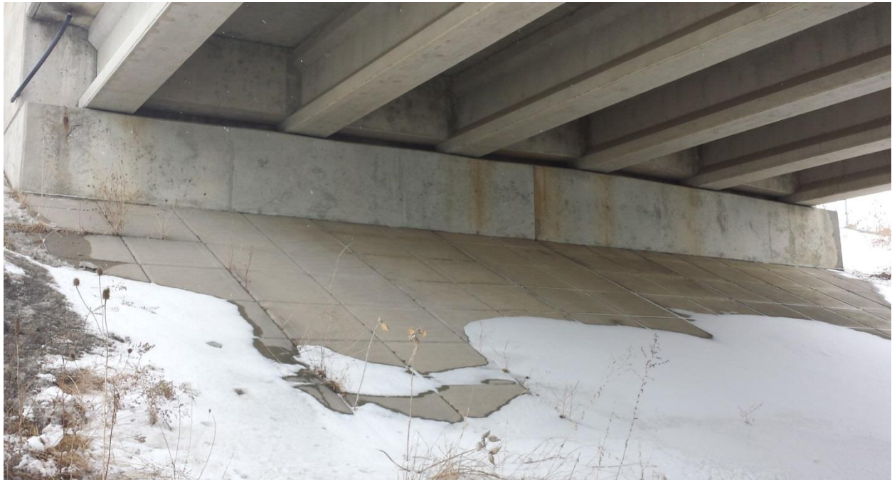
Photograph 3: Looking at west abutment of EBL structure. Front slope covered with concrete, no obvious major cracks observed except surficial cracks on the abutment wall. No weeping hole or outlet system observed out of abutment wall. (February 19, 2014)
