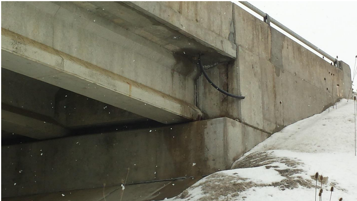
Photograph 8: Looking at north wingwall of the west abutment of WBL structure; no obvious major cracks observed except for surficial cracks. Slope covered with snow and withered grasses.
