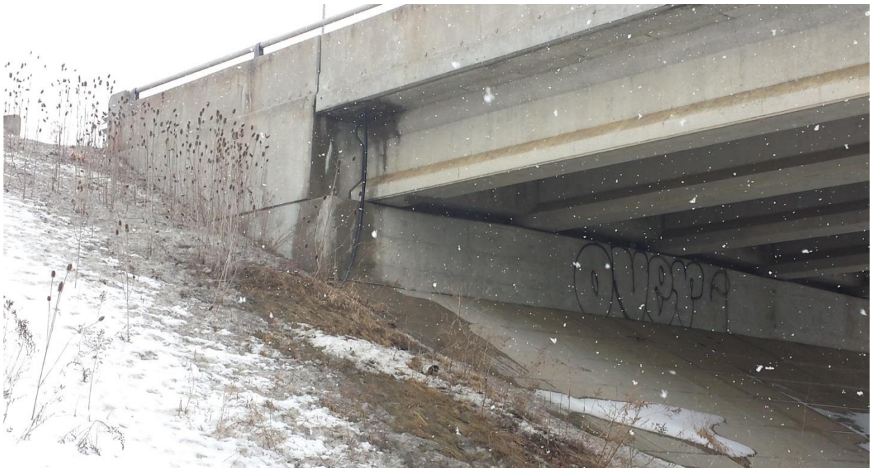
Photograph 6: Looking at south wingwall of the west abutment of WBL structure; no obvious major cracks observed except for surficial cracks. Slight erosion was observed on the exposed slope. (February 19, 2014)
