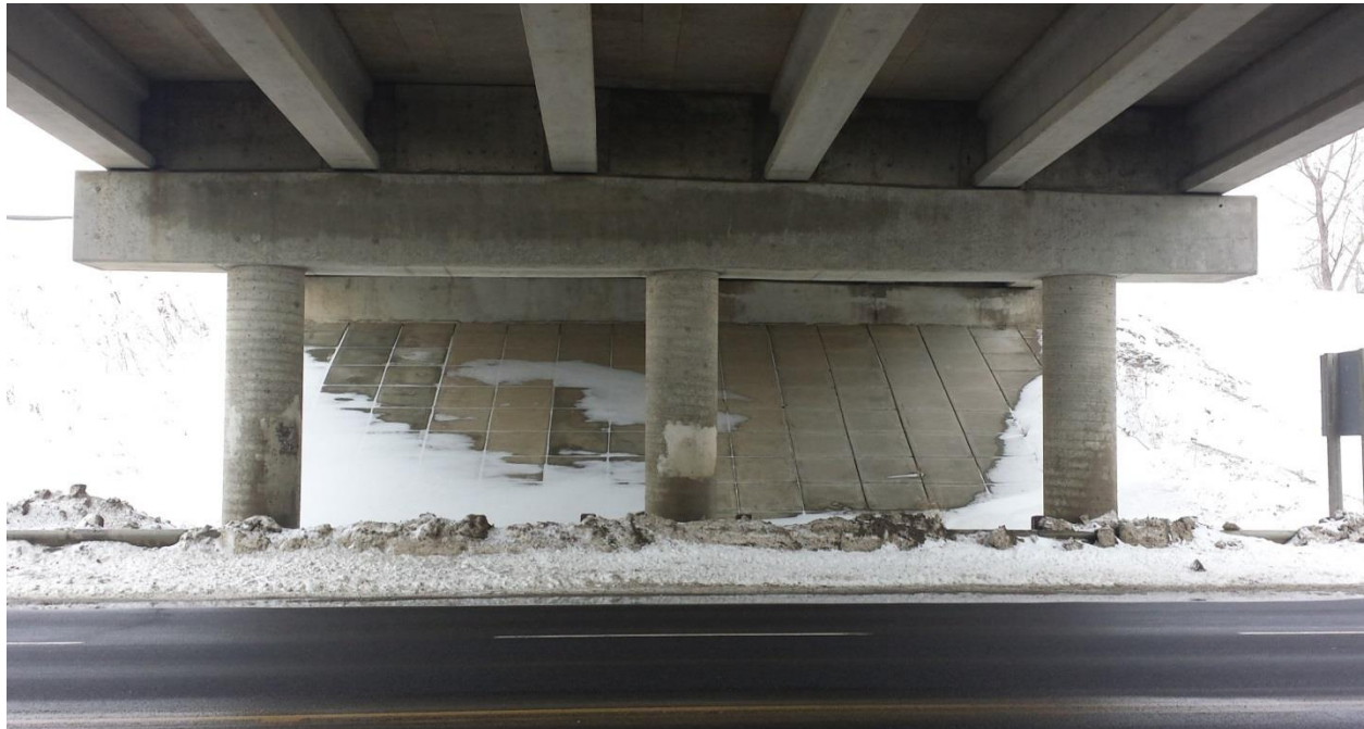
Photograph 4: Looking at east abutment wall and piers of EBL structure. Front slope covered with concrete; no obvious major cracks observed except for surficial cracks. No weeping hole or outlet system observed on abutment wall. Some surface rehabilitation of the piers was performed. (February 19, 2014)
