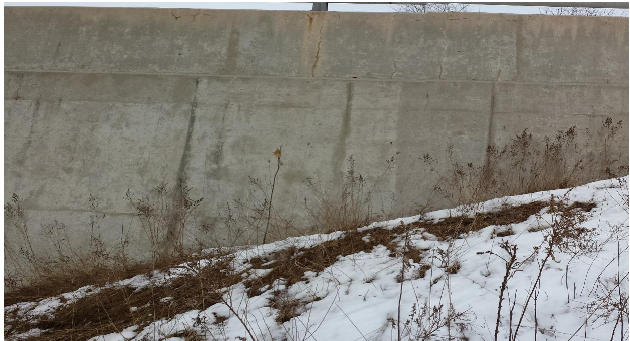
Photograph 4: Looking at the south wingwall of the east abutment wall. Surficial cracks were visible on the wall. No soil erosion was observed of the limited exposed ground surface of the slope face. (February 19, 2014)
