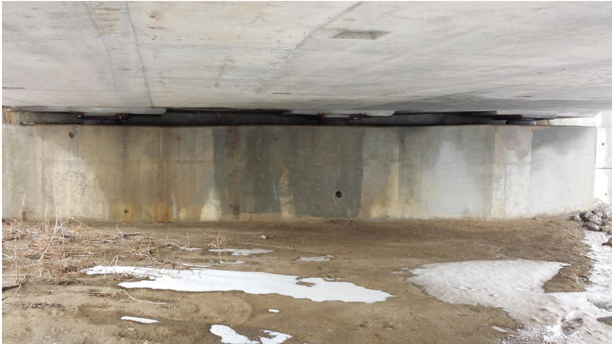
Photograph 8: Looking at the west abutment. Slight erosion of the exposed ground in front of the abutment wall was observed. A weep hole in the wall was observed. (February 19, 2014)
