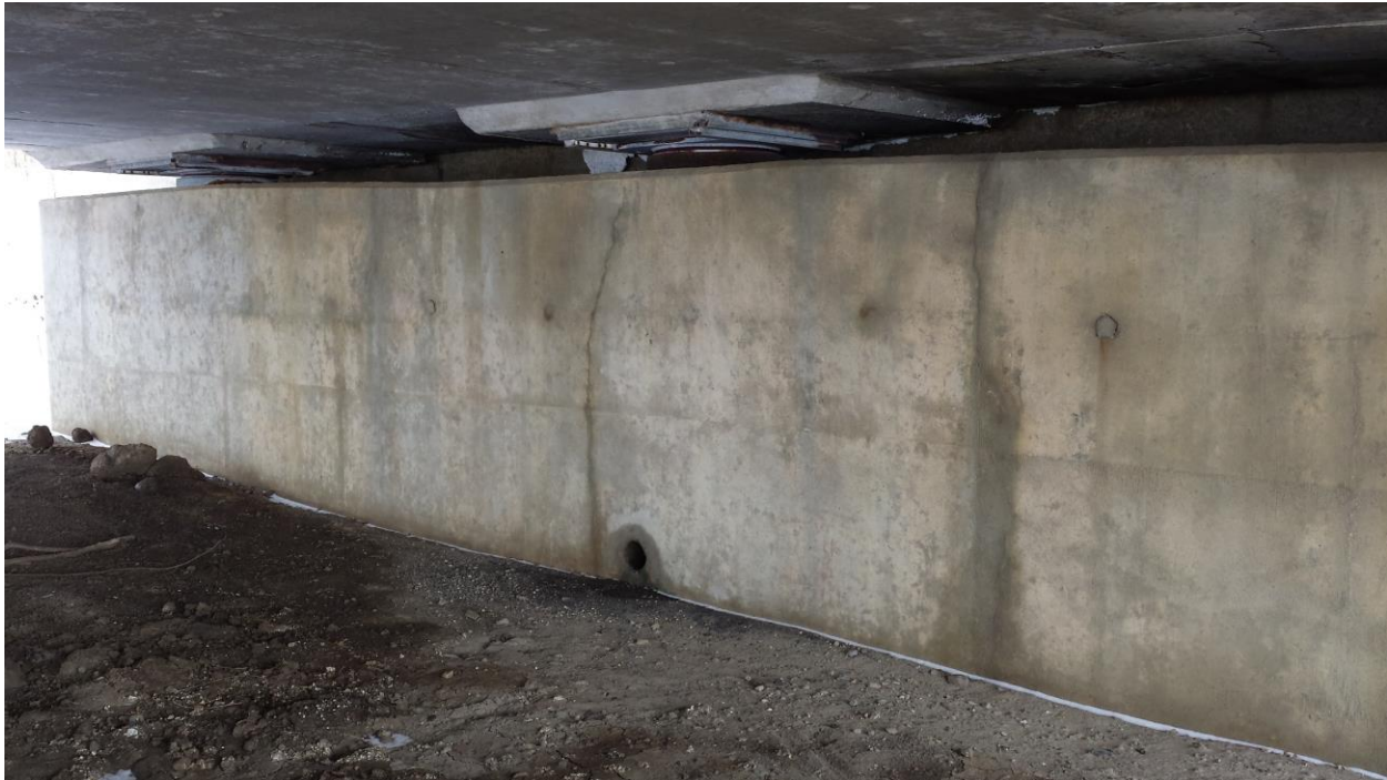
Photograph 3: Looking at the east abutment wall. Slight soil erosion of the exposed ground was visible. Surface cracks were observed on the abutment wall. Also, presence of a weep hole was observed in the wall. (February 19, 2014)
