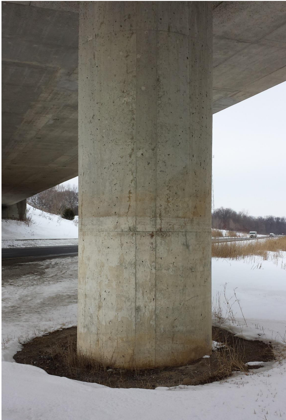
Photograph 6: Looking north at the center pier. Slight surficial soil erosion was observed around the pier. Minor longitudinal surficial cracks are present. (February 19, 2014)
