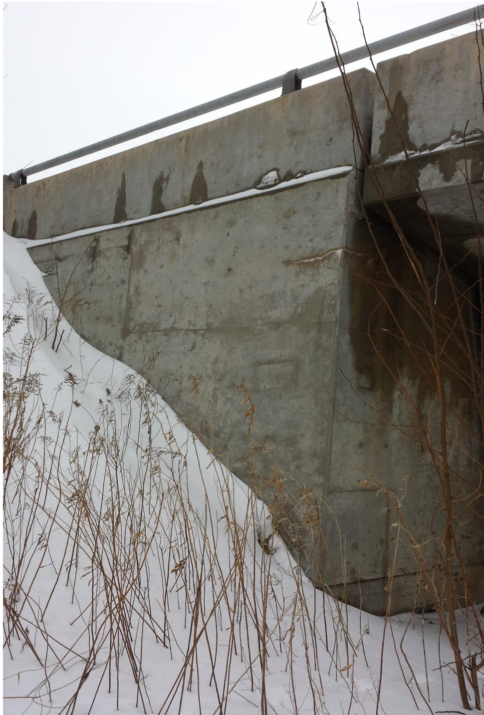
Photograph 5: Looking at the north wingwall of the east abutment. Surficial cracks were present on the wall. The adjacent slope surface was covered with snow. (February 19, 2014)
