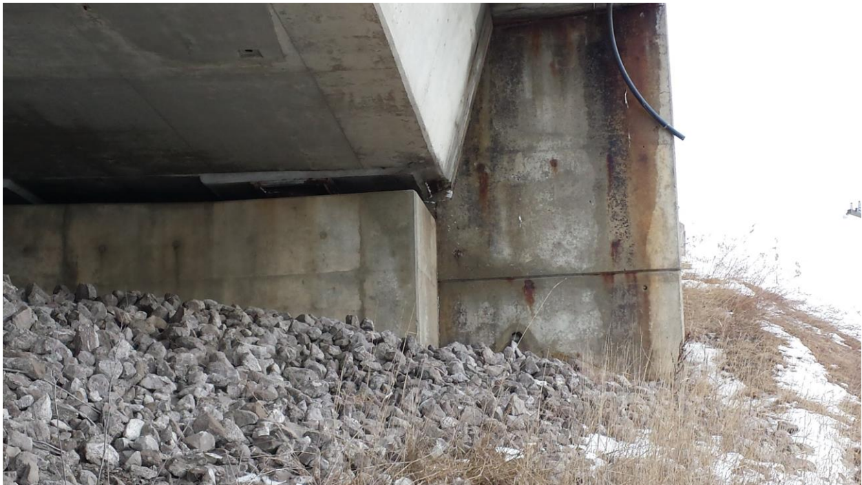
Photograph 2: Looking at the east abutment showing rip-rap stones in front the north wingwall. Weep hole observed in the wingwall (February 19, 2014).
