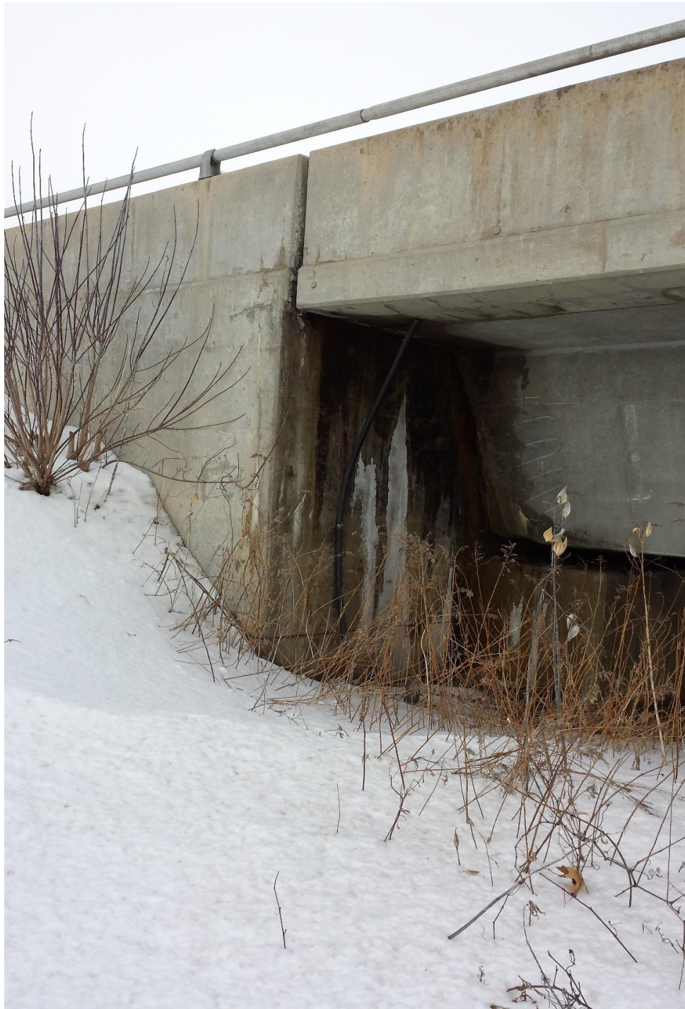
Photograph 9: Looking at the north wing wall of the west abutment. Minor surficial cracks are present on the wall. The ground and the slope surface was covered with snow. (February 19, 2014)
