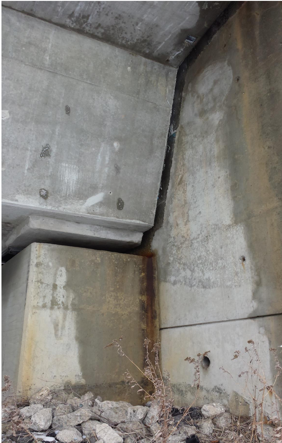
Photograph 7: Looking at the south wingwall of the west abutment showing rip-rap stones in front the wing wall. A weep hole was observed in the wingwall (February 19, 2014)
