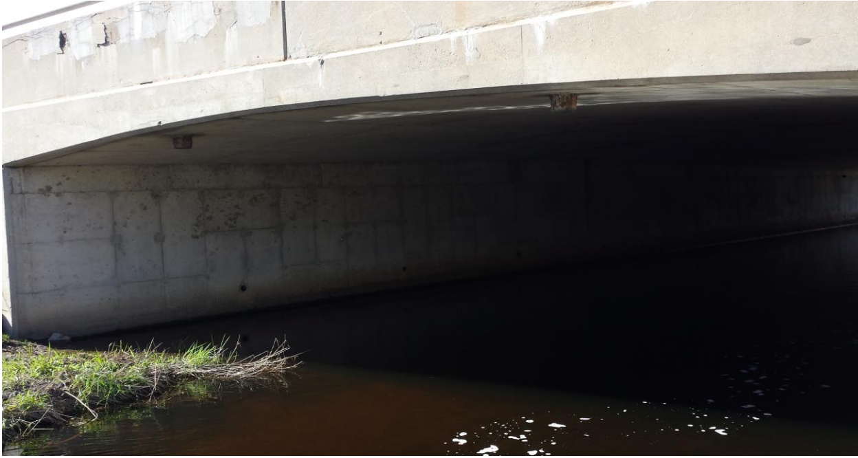
Photograph 5: Looking west from the south slope of the east side of the bridge towards the west abutment wall. Weep holes out of the abutment wall as observed. Scouring below the water could not been observed. (May 10, 2014)
