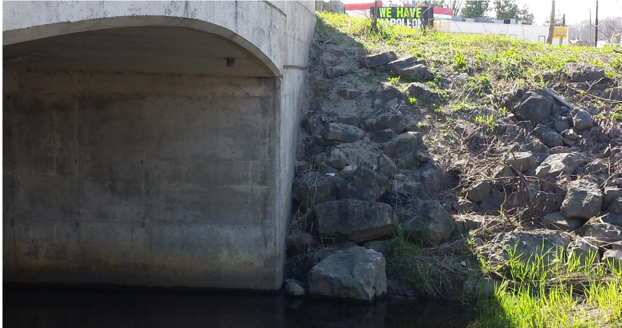
Photograph 3: Looking west at the north slope adjacent to the west abutment. Erosion of the slope face with rocks scattered to mitigate further erosion was observed. Slight scouring of the slope toe was also observed. (May 10, 2014)
