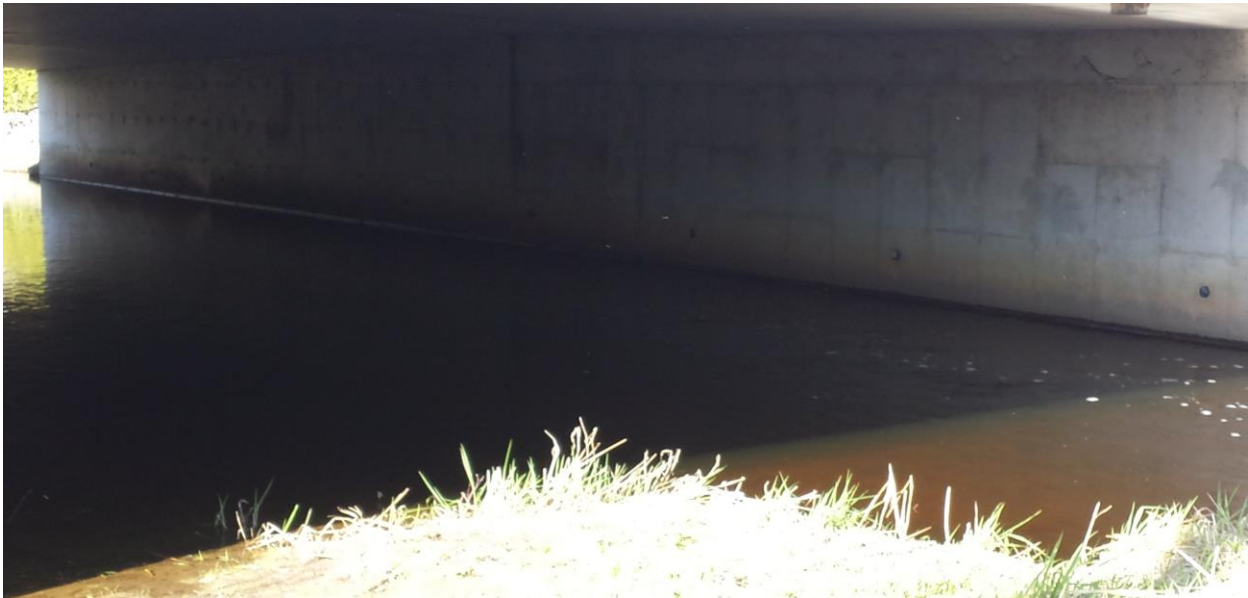
Photograph 6: Looking east from the south slope of the west side of the bridge towards the east abutment wall. Weep holes out of the abutment wall as observed. Scouring below the water could not been observed. (May 10, 2014)
