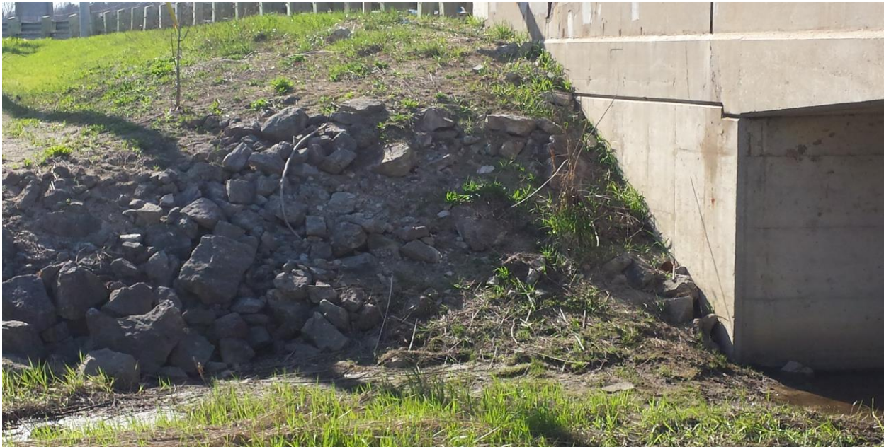
Photograph 1: Looking west at the adjacent south slope of the west abutment from the south slope of the east side of the bridge. Erosion of the slope face and scouring of the slope toe was observed. (May 10, 2014).
