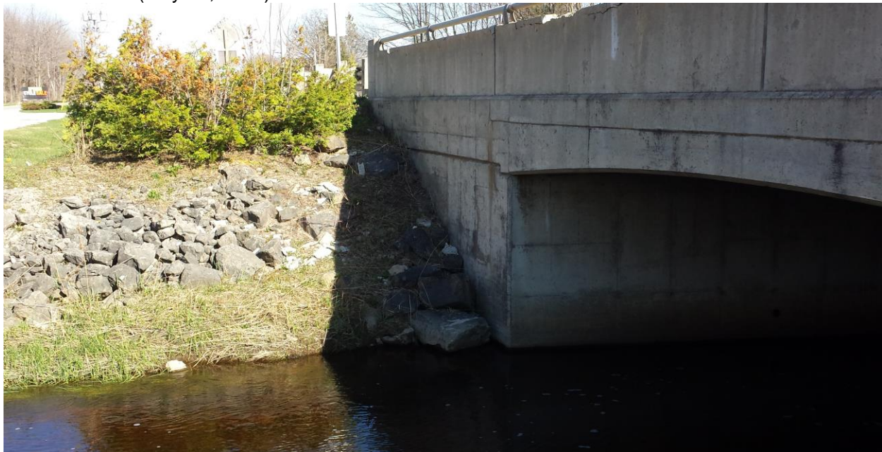
Photograph 4: Looking east at the north slope adjacent to the east abutment. Rocks placed on the slope with slight erosion on the slope face was observed. Further, scouring of the slope toe was also observed. (May 10, 2014)
