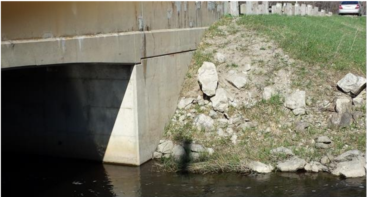
Photograph 2: Looking east at the south slope adjacent to the east abutment. Slight erosion of the slope face with scattered rocks placed were observed. Further, scouring of the slope toe was observed. (May 10, 2014)
