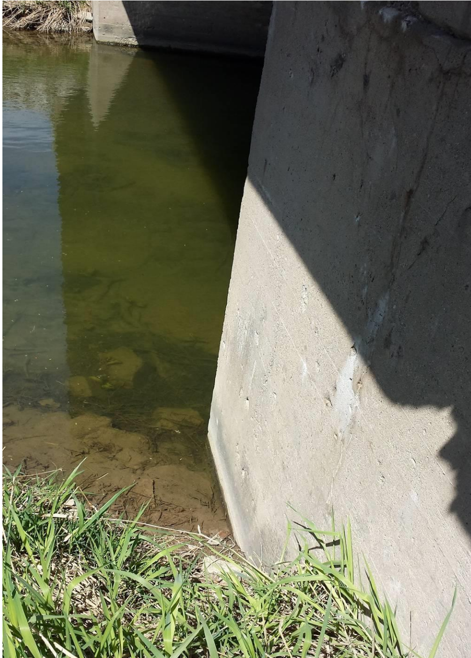
Photograph 4: Looking at the east slope adjacent to the south abutment. Scouring of the slope toe edge was observed. Concrete deterioration on east wingwall of the south abutment was also observed. (May 10, 2014)
