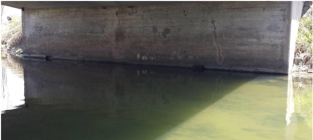
Photograph 6: Looking south from the west slope of the north side of the bridge. Minor surface cracks, wall surface deterioration and a visible crack on the south abutment wall were observed. Concrete spillings off the wall at the water level was also observed. Potential scouring effect could not be verified under the water at the abutment wall. (May 10, 2014)
