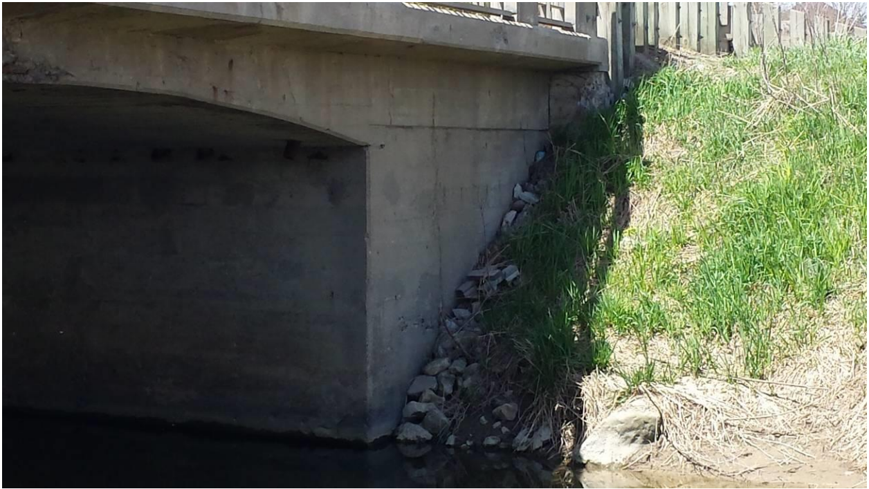
Photograph 1: Looking north at the adjacent east slope of the north abutment from the east slope of the south side of the bridge. Cracks were observed on the wingwall. Slight scouring of the slope toe edge was observed. (May 10, 2014)
