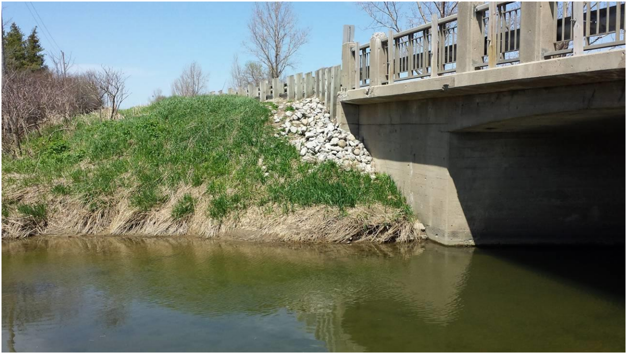
Photograph 7: Looking north at the west slope adjacent to the north abutment. Rock protection placed on the slope to prevent slope surface erosion. (May 10, 2014)
