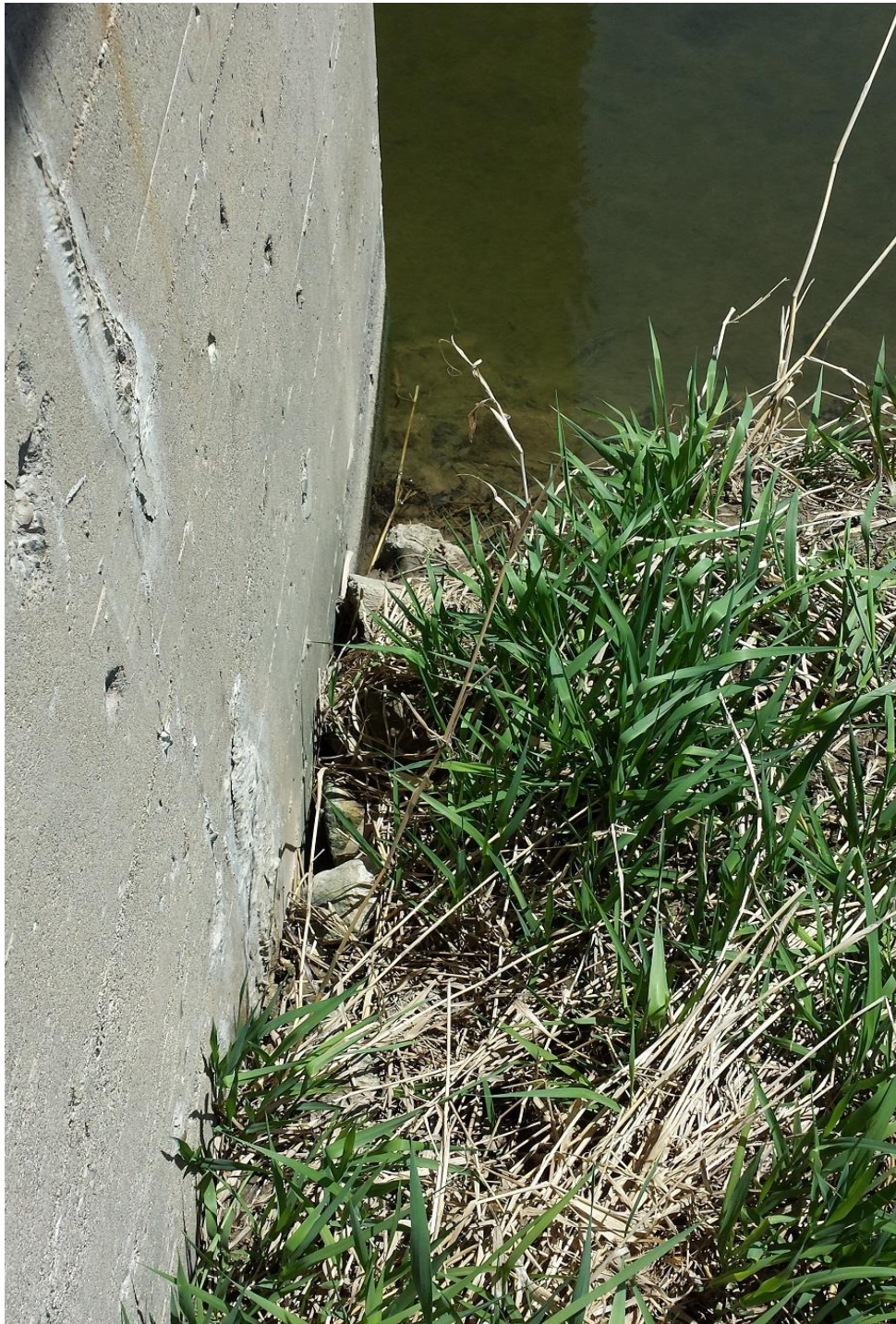
Photograph 3: Looking at the west slope adjacent to the north abutment. Scouring of the slope toe edge was observed. Concrete deterioration on wingwall was also observed. (May 10, 2014)
