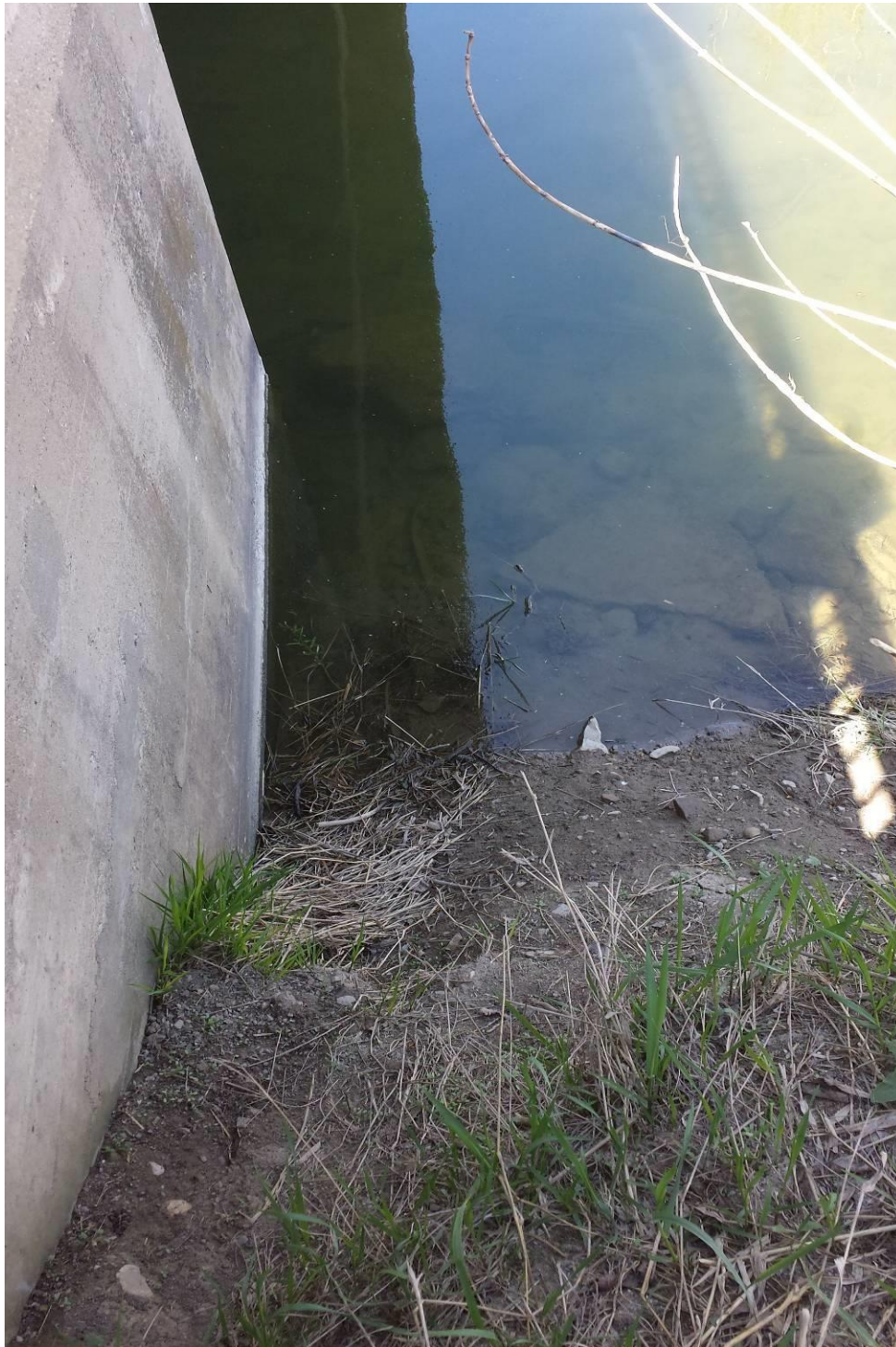
Photograph 2: Looking at the east slope adjacent to the south abutment. Scouring of the slope toe edge and erosion of the slope surface were observed. (May 10, 2014)
