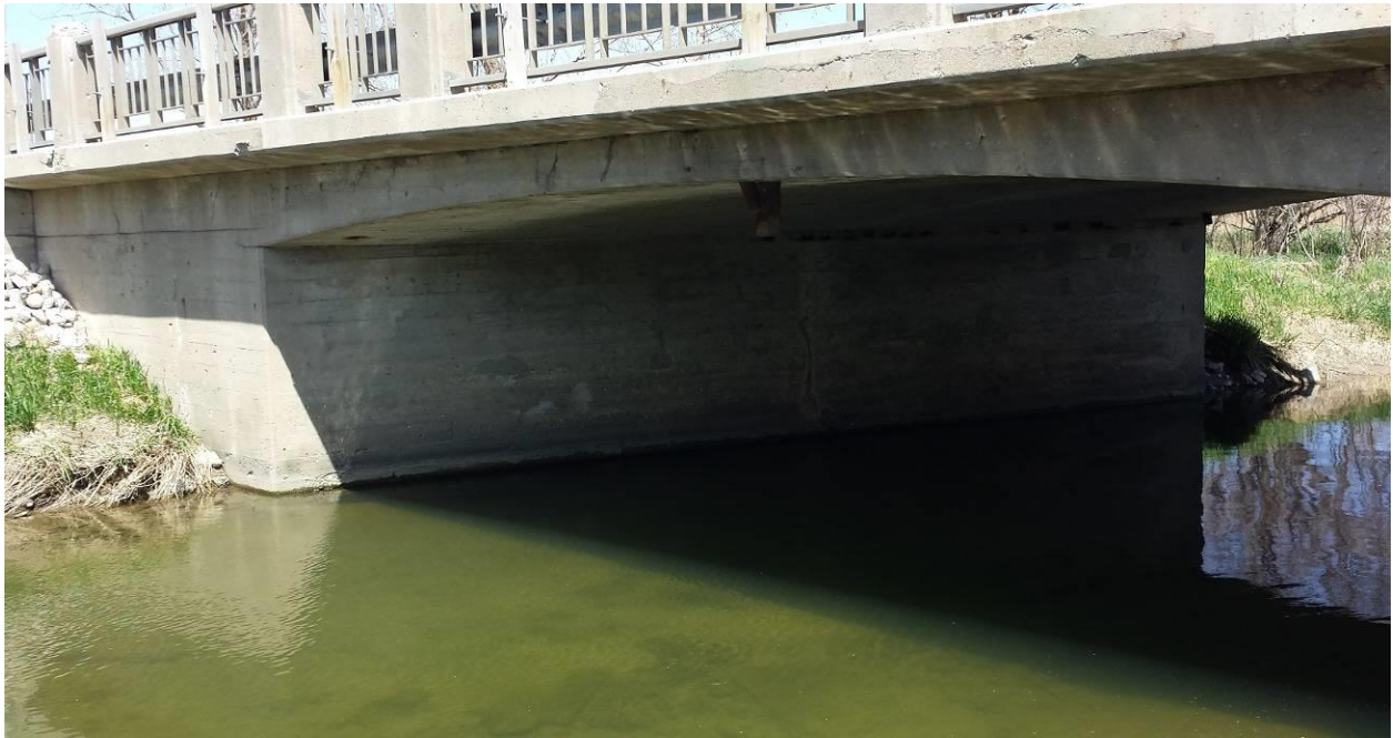
Photograph 5: Looking north from the west slope of the south side of the bridge. Minor surface cracks, wall surface deterioration and a visible crack on the north abutment wall were observed. Potential scouring effect could not be verified under the water at the abutment wall. (May 10, 2014)
