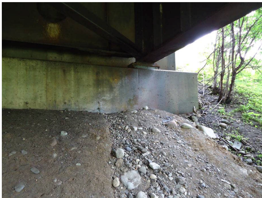
PHOTOGRAPH 18: Erosion on front slope of west abutment of EBL. (June 11, 2013)
