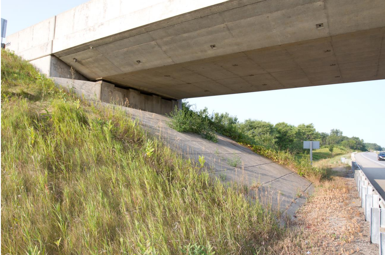
Photograph 1: Looking at the south abutment of the Maple Road Underpass Structure. Vertical cracks were observed on the abutment wall. Weep holes were not observed in the abutment wall. Sealant between the concrete panels appeared degraded at locations where grasses and shrubs are growing. The toe of the front slope was covered partially with gravel (August 28, 2015).
