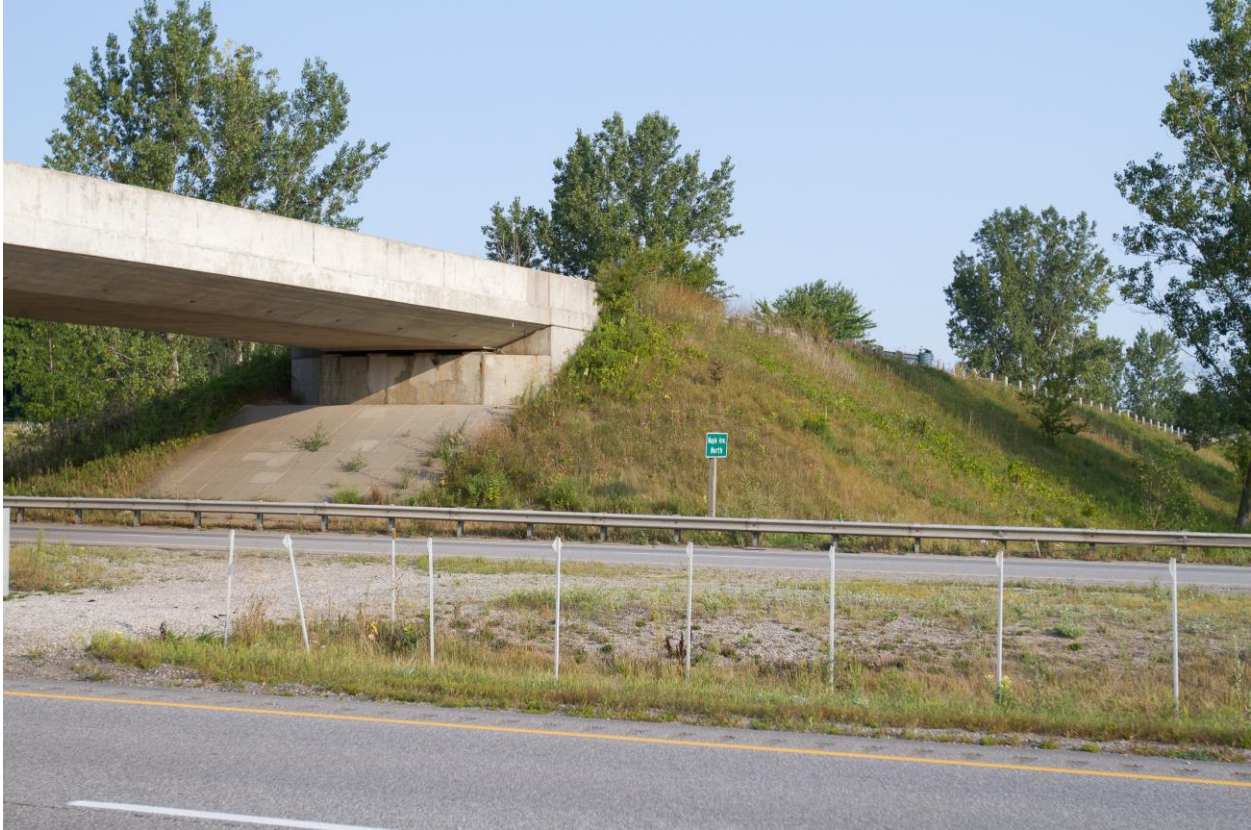
Photograph 7: Looking at the east wingwall and the adjacent slope of the north abutment of the Maple Road Underpass Structure. Minor cracks were observed on the wingwall. The slope is vegetated and effect of erosion on the slope face was not observed (August 28, 2015).
