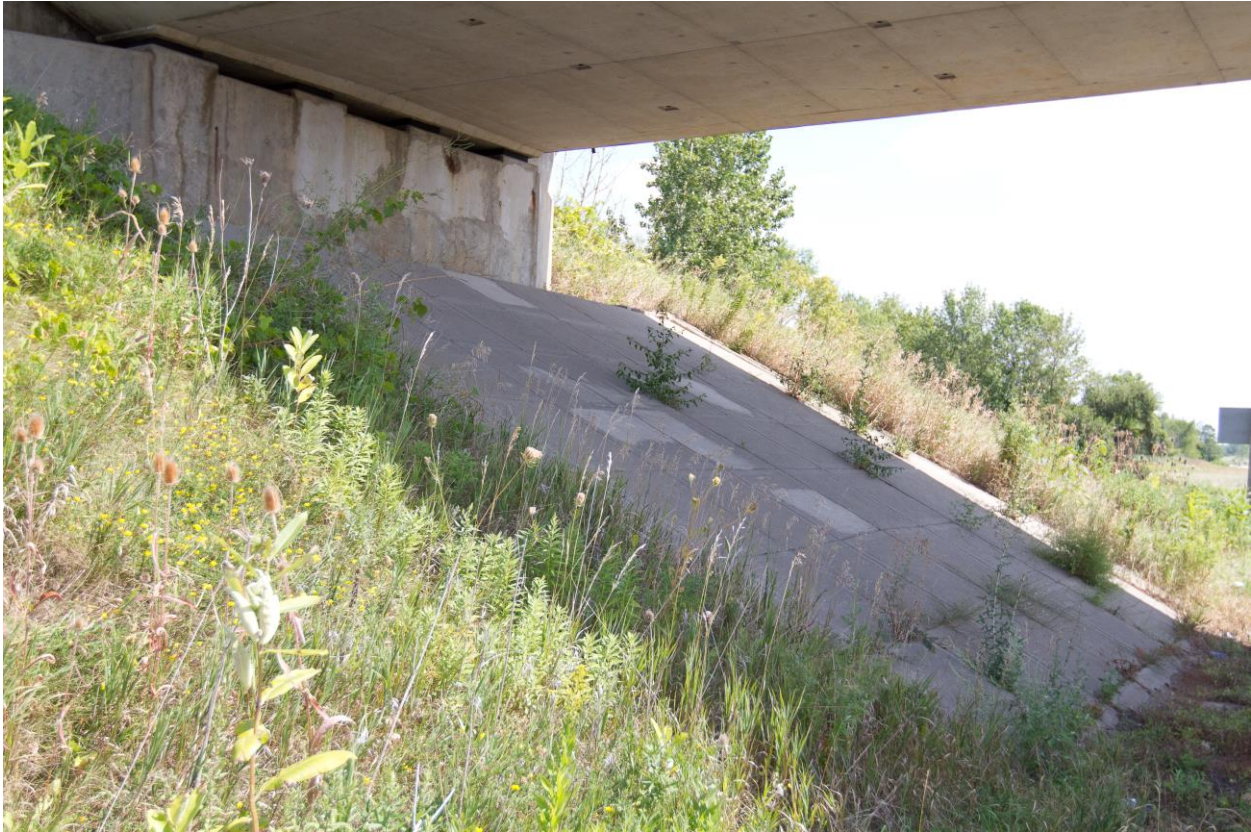
Photograph 2: Looking at the north abutment of the Maple Road Underpass Structure. Random cracks were observed on the abutment wall. Weep holes were not observed in the abutment wall. Sealant between the concrete panels appeared degraded at locations where grasses and shrubs are growing. Few of the concrete panels appeared to have been rehabilitated. The toe of the front slope was vegetated with localized erosion of soil at ground surface (August 28, 2015).
