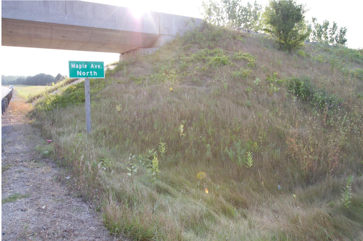
Photograph 5: Looking at the west wingwall and the adjacent slope of the south abutment of the Maple Road Underpass Structure. Surficial cracks were observed on the wingwall. The slope is vegetated and effect of erosion on the slope face was not observed (August 28, 2015).
