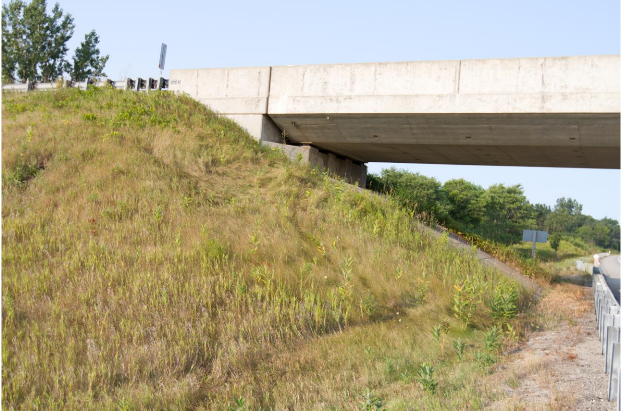
Photograph 4: Looking at the east wingwall and the adjacent slope of the south abutment of the Maple Road Underpass Structure. Surficial cracks were observed on the wingwall. The slope is vegetated and effect of erosion on the slope face was not observed (August 28, 2015).
