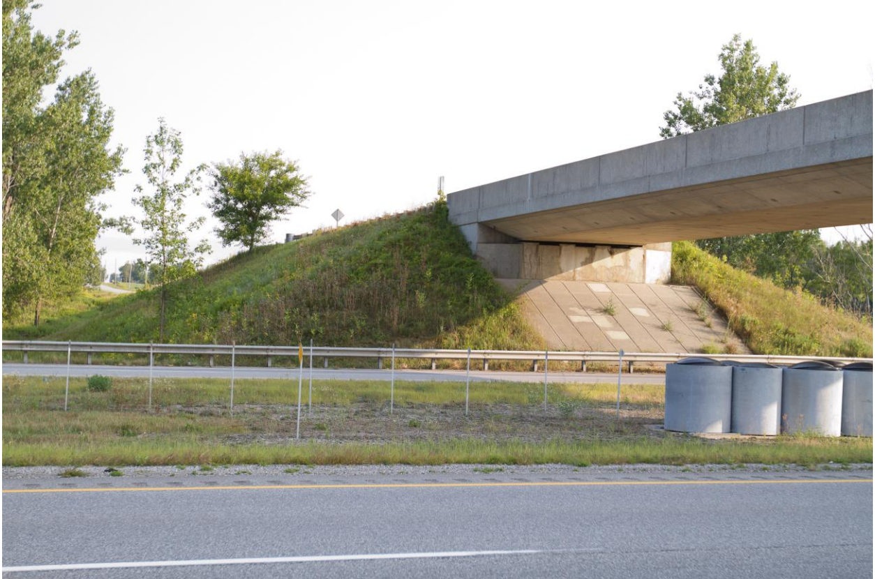
Photograph 6: Looking at the west wingwall and the adjacent slope of the north abutment of the Maple Road Underpass Structure. Surficial cracks were observed on the wingwall. The slope is vegetated and effect of erosion on the slope face was not observed (August 28, 2015).
