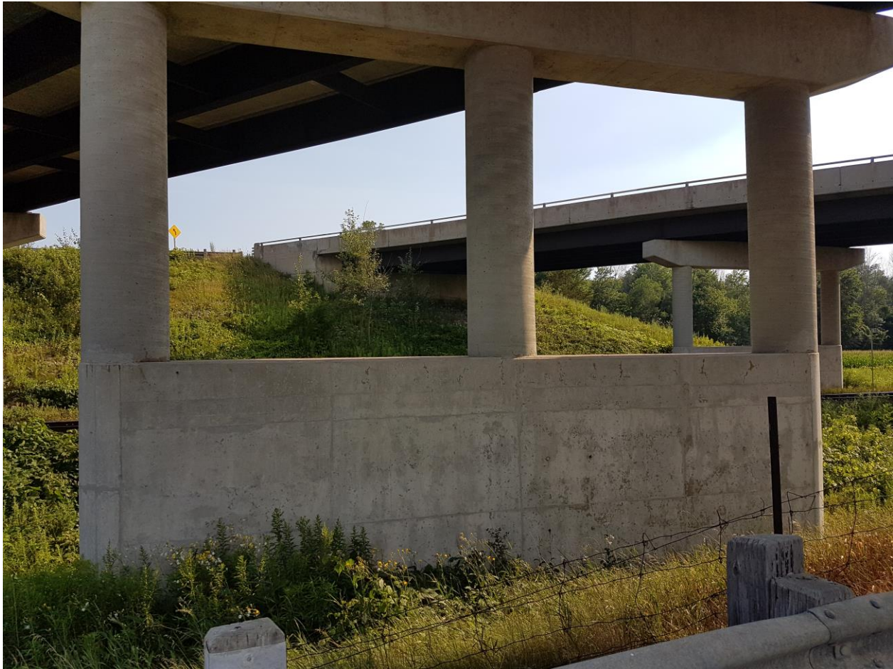
Photograph 15: Looking at the Pier No. 2 with the crash wall of the CNR WBL structure from the service road. Surficial cracks were observed on the pier and the crash wall. The ground around the crash wall was vegetated and effect of erosion was not observed (July 27, 2016).
