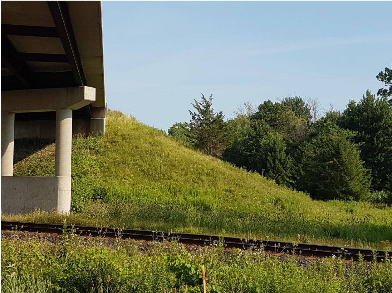
Photograph 9: Looking at the east abutment, the Pier No. 3, the south slope adjacent to east abutment of the CNR EBL structure and single CNR track from the service road. The adjacent slope is vegetated and effect of erosion on the slope face was not observed (July 27, 2016).
