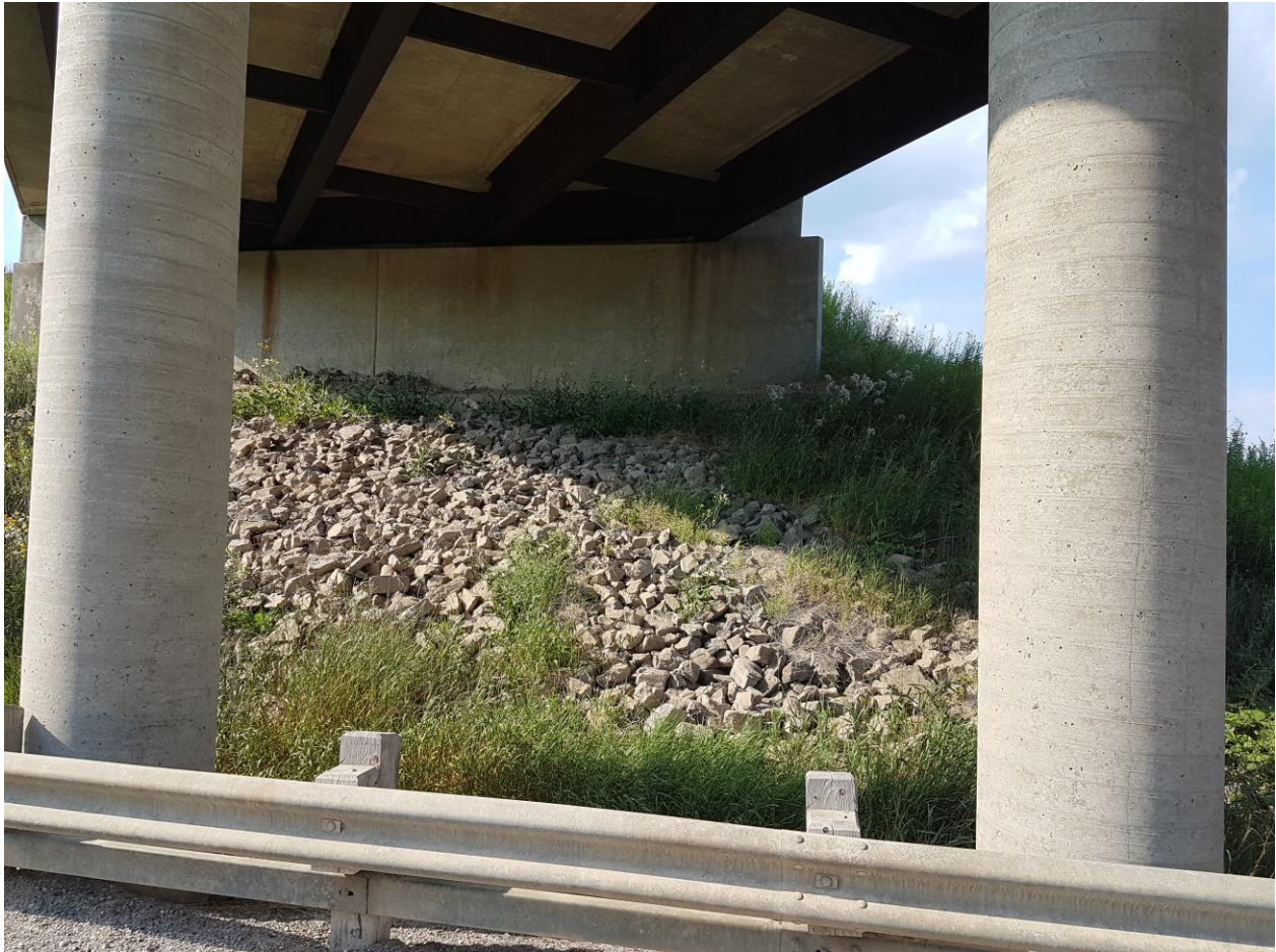
Photograph 14: Looking at the west abutment and the Pier No. 1 of the CNR WBL structure from the service road. Crushed rock protection was covering the front slope of the abutment. Surficial cracks were observed on the pier (July 27, 2016).
