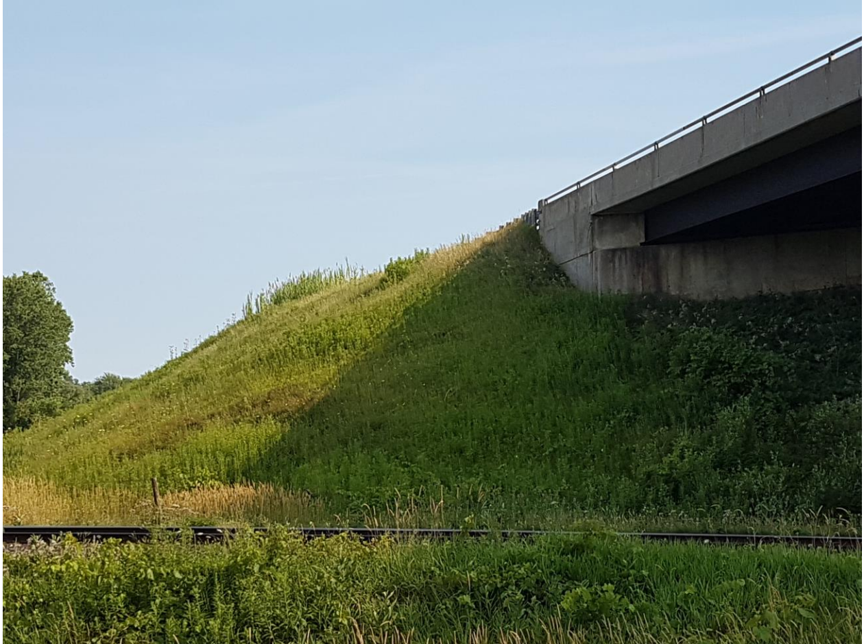
Photograph 19: Looking at the north wing wall and the adjacent slope of east abutment of the CNR WBL structure and single CNR track from the service road. Surficial cracks were observed on the wing wall. The slope is vegetated and effect of erosion on the slope face was not observed (July 27, 2016).
