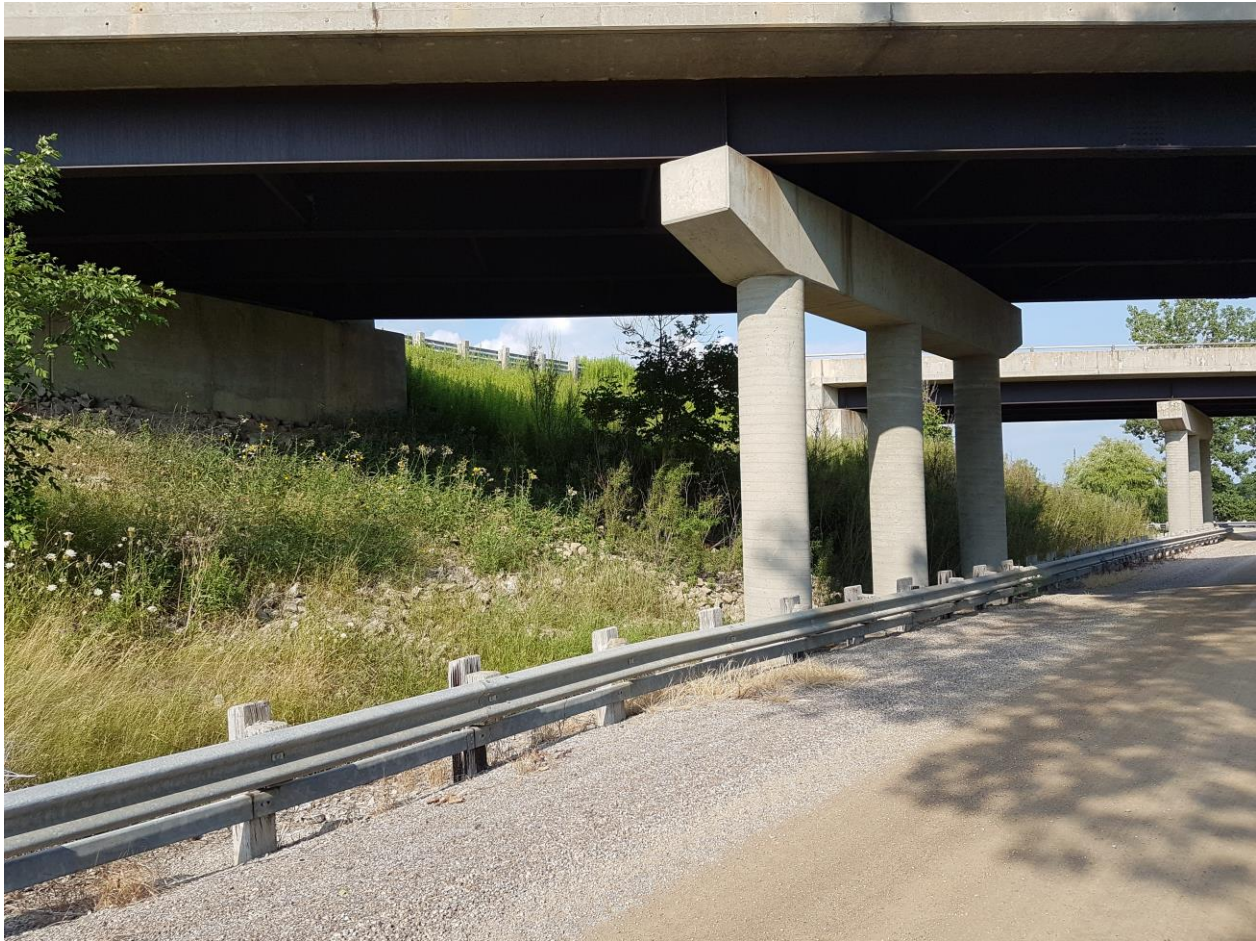
Photograph 4: Looking at the west abutment and the Pier No. 1 of the CNR EBL structure from the service road. Crushed rock protection of the front slope of the abutment was observed. Surficial cracks were observed on the piers (July 27, 2016).
