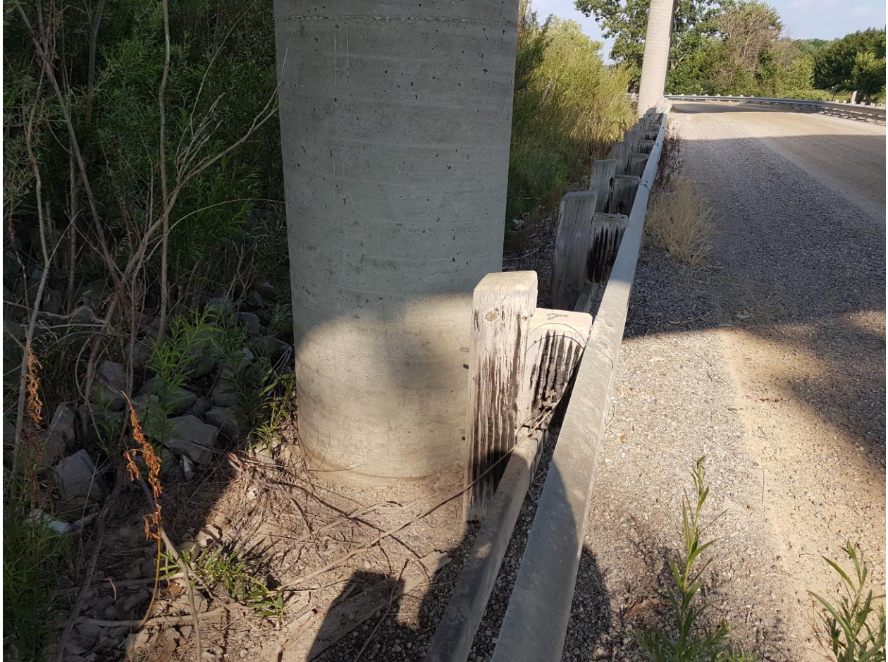
Photograph 5: Looking at the northerly column of Pier No. 1 of the CNR EBL Structure. Slight erosion at the foot of the pier was observed (July 27, 2016).
