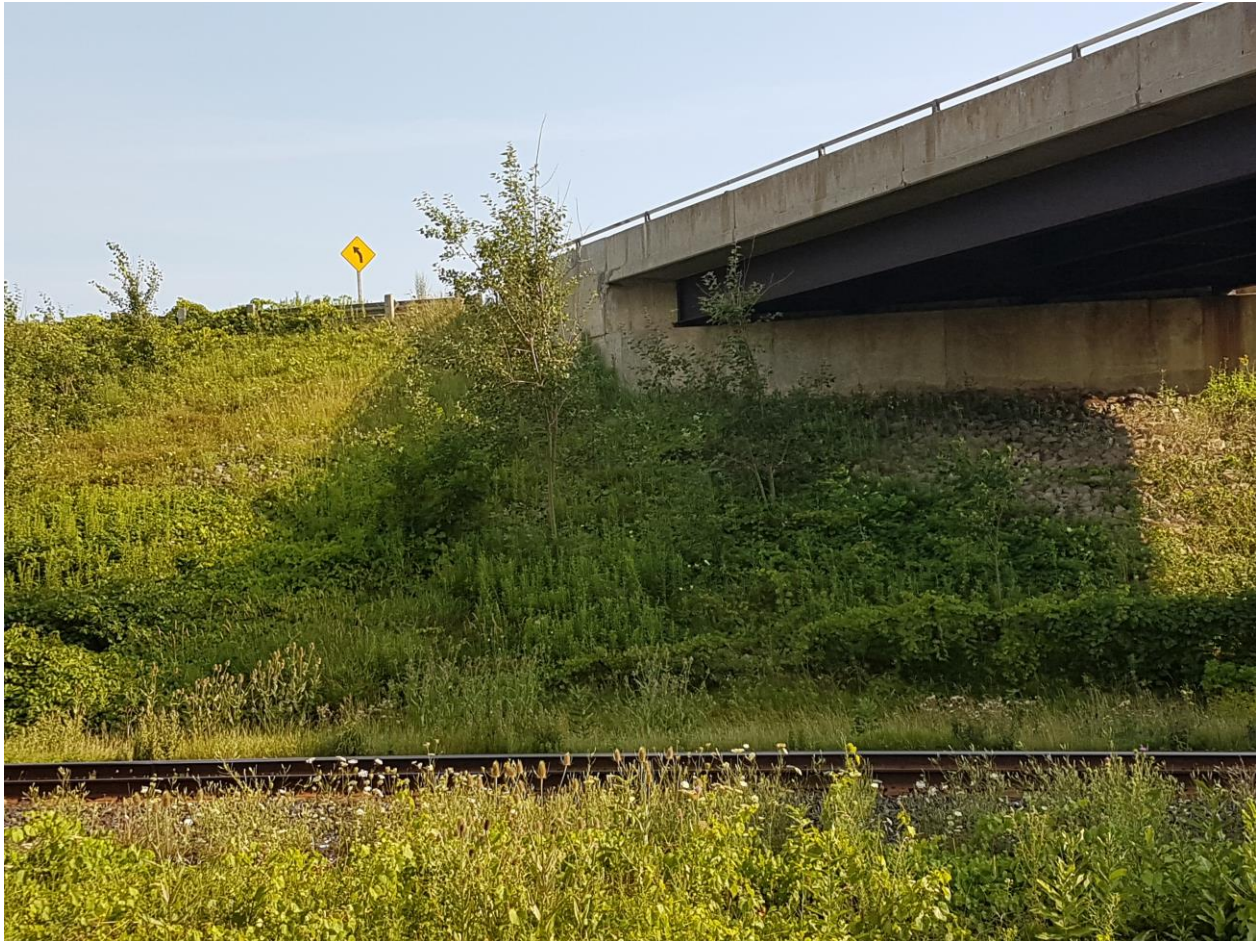
Photograph 10: Looking at the north wing wall of the east abutment of the CNR EBL structure, the slope adjacent to the east abutment and the single CNR track. Surficial cracks were observed on the wing wall. Also, a local concrete spalling area was observed at the corner of the wing wall. The adjacent slope is vegetated and effect of erosion on the slope face was not observed (July 27, 2016).
