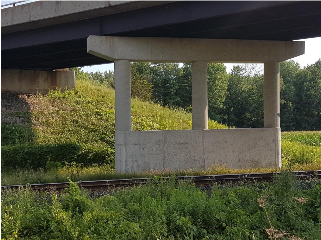
Photograph 7: Looking at the Pier No. 3 with the crash wall and east abutment of the CNR EBL structure and the single CNR track from the service road. Surficial cracks were observed on the pier and the crash wall (July 27, 2016).
