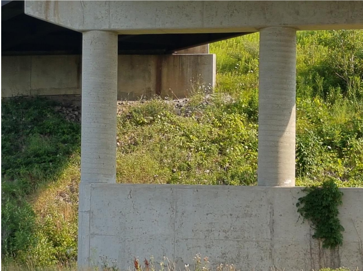
Photograph 16: Looking at the Pier No. 3 with the crash wall of the CNR WBL structure from the service road. Surficial cracks were observed on the pier and the crash wall. The ground around the crash wall was vegetated and effect of erosion was not observed (July 27, 2016).
