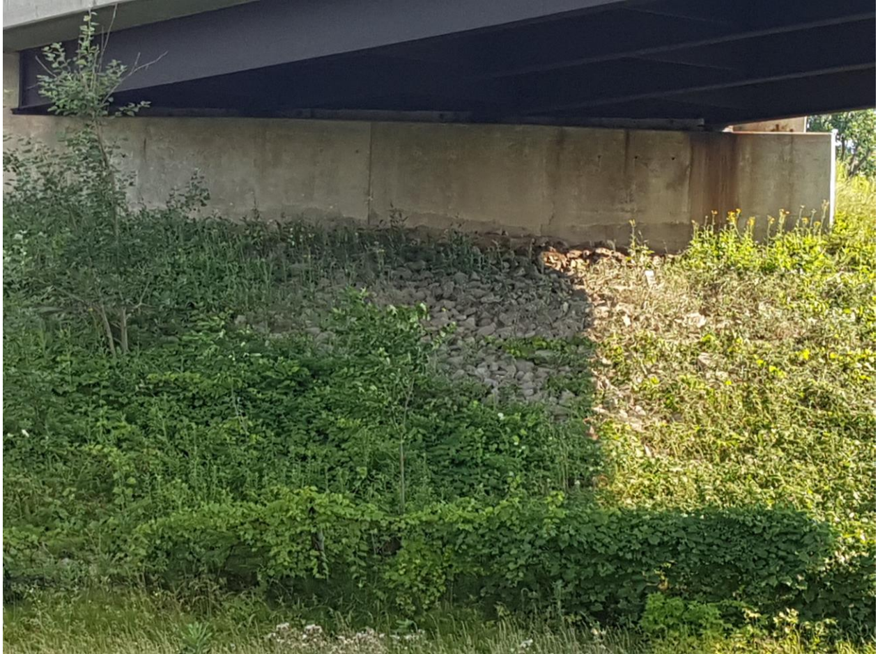
Photograph 8: Looking at the east abutment with the front slope of the CNR EBL structure from the service road. Surficial cracks were observed on the abutment wall. The front slope of the east abutment is covered with crushed rock. Effect of erosion on the slope face was not observed (July 27, 2016).
