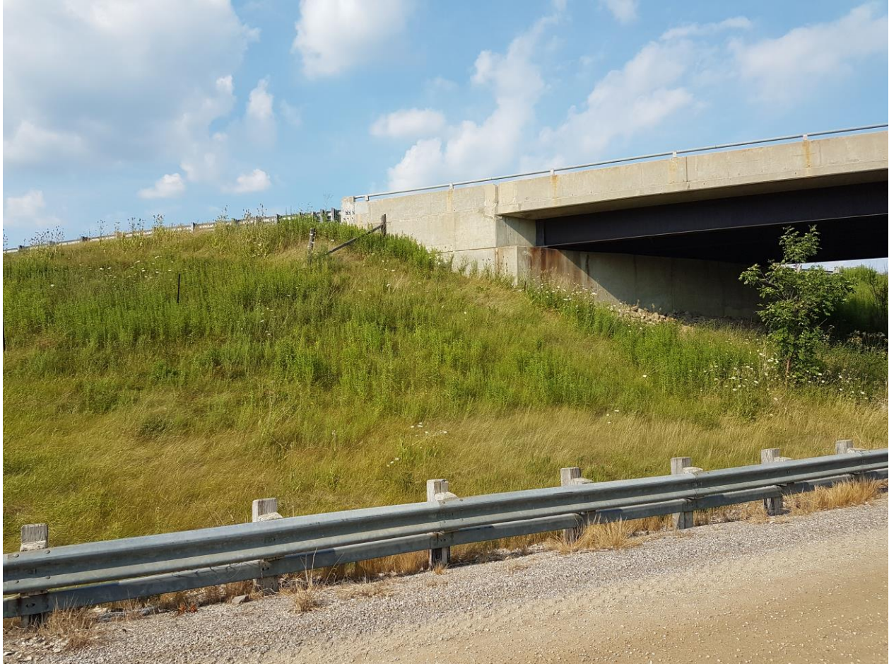
Photograph 2: Looking at the south wing wall and the adjacent slope of west abutment of the CNR EBL structure from the service road. Surficial cracks were observed on the abutment wall and the wing wall. The adjacent slope is vegetated and effect of erosion on the slope face was not observed (July 27, 2016).
