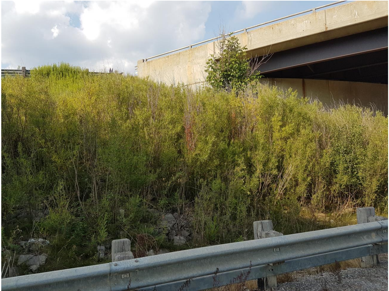
Photograph 12: Looking at the south wing wall and the adjacent slope of west abutment of the CNR WBL structure from the service road. Surficial cracks were observed on the wing wall. The adjacent slope is heavily vegetated and effect of erosion on the slope face was not observed (July 27, 2016).
