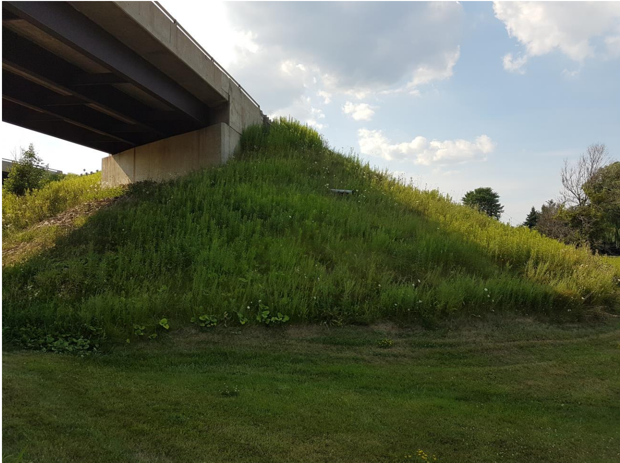
Photograph 13: Looking at the north wing wall and the adjacent slope of west abutment of the CNR Overhead WBL structure from the service road. Surficial cracks were observed on the wing wall. A C.S.P. was observed on the side slope. The slope is vegetated and effect of erosion on the slope face was not observed (July 27, 2016).
