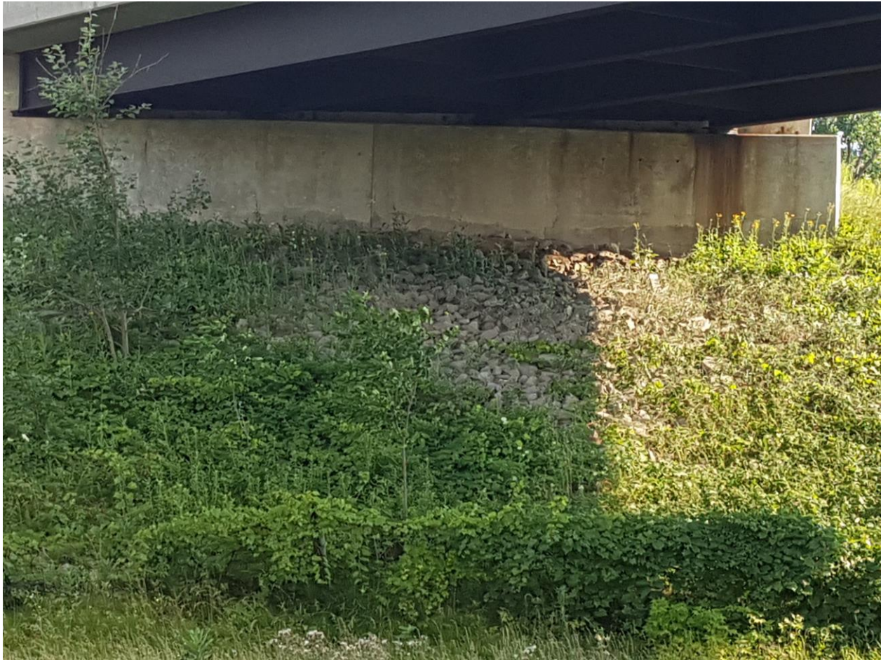
Photograph 17: Looking at the east abutment of the CNR WBL structure from the service road. Surficial cracks were observed on the abutment wall. The front slope is covered with crushed rock and effect of erosion was not observed (July 27, 2016).
