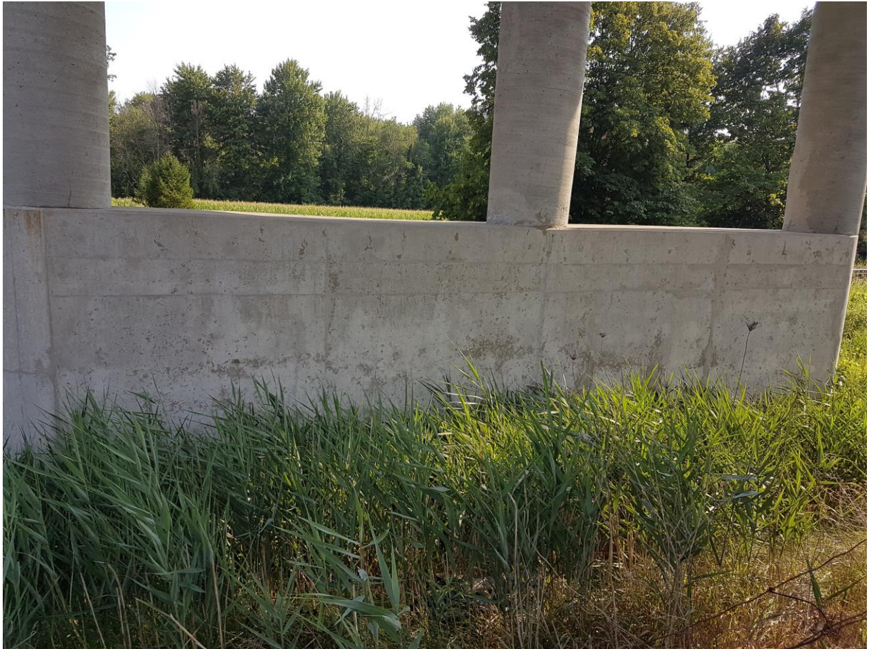
Photograph 6: Looking at the Pier No. 2 with crash wall of the CNR EBL structure from the service road. Surficial cracks were observed on the columns and crash wall. The ground was vegetated and effect of erosion was not observed (July 27, 2016).
