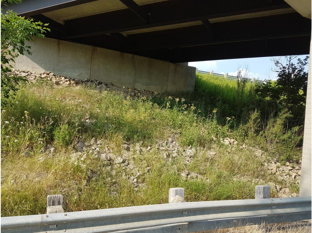
Photograph 1: Looking at the west abutment of the CNR EBL structure from the service road. Surficial cracks were observed on the abutment wall. The front slope was covered with crushed rock (July 27, 2016).
