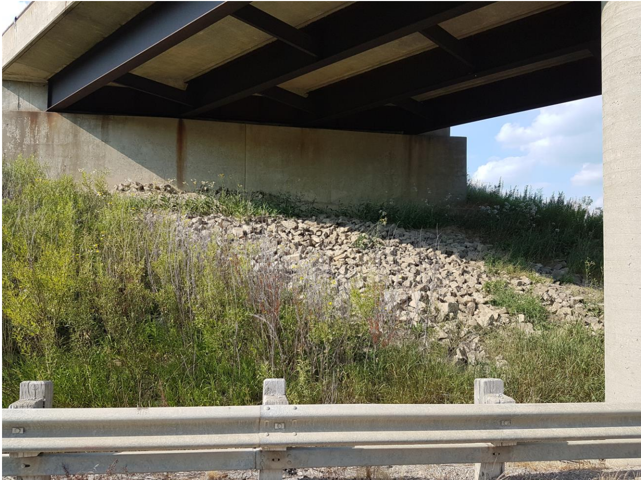
Photograph 11: Looking at the west abutment of the CNR WBL structure and the front slope. Surficial cracks were observed on the abutment wall from the service road. The slope is covered with crushed rock and effect of erosion on the slope face was not observed (July 27, 2016).
