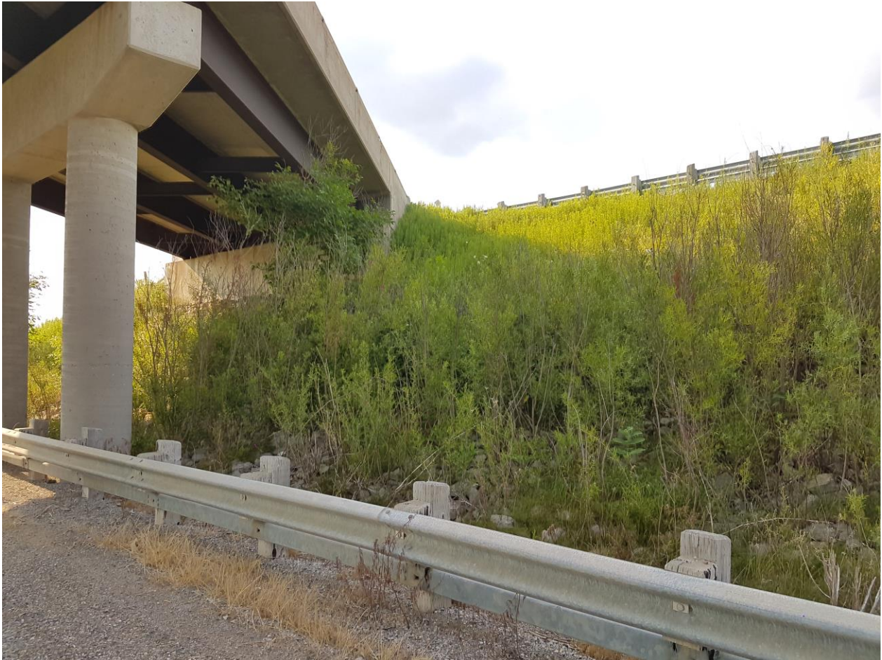
Photograph 3: Looking at the north wing wall and the adjacent slope of west abutment and the Pier No. 1 of the CNR EBL Structure from the service road. Surficial cracks were observed on the abutment wall, wing wall and pier. The adjacent slope is vegetated and effect of erosion on the slope face was not observed (July 27, 2016).
