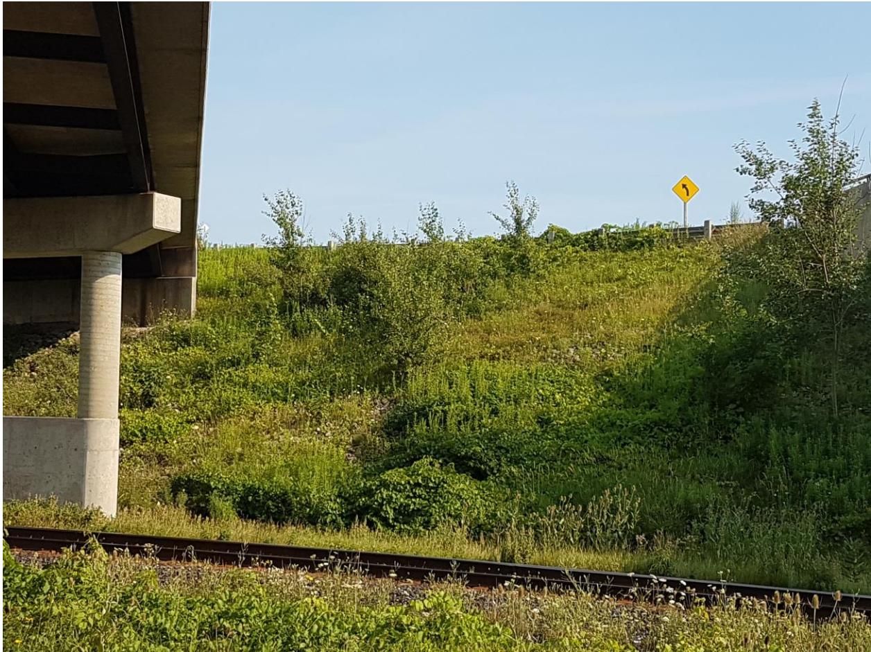
Photograph 18: Looking at the south adjacent slope of east abutment of the CNR WBL structure and single CNR track from the service road. The adjacent slope is vegetated and effect of erosion on the slope face was not observed (July 27, 2016).
