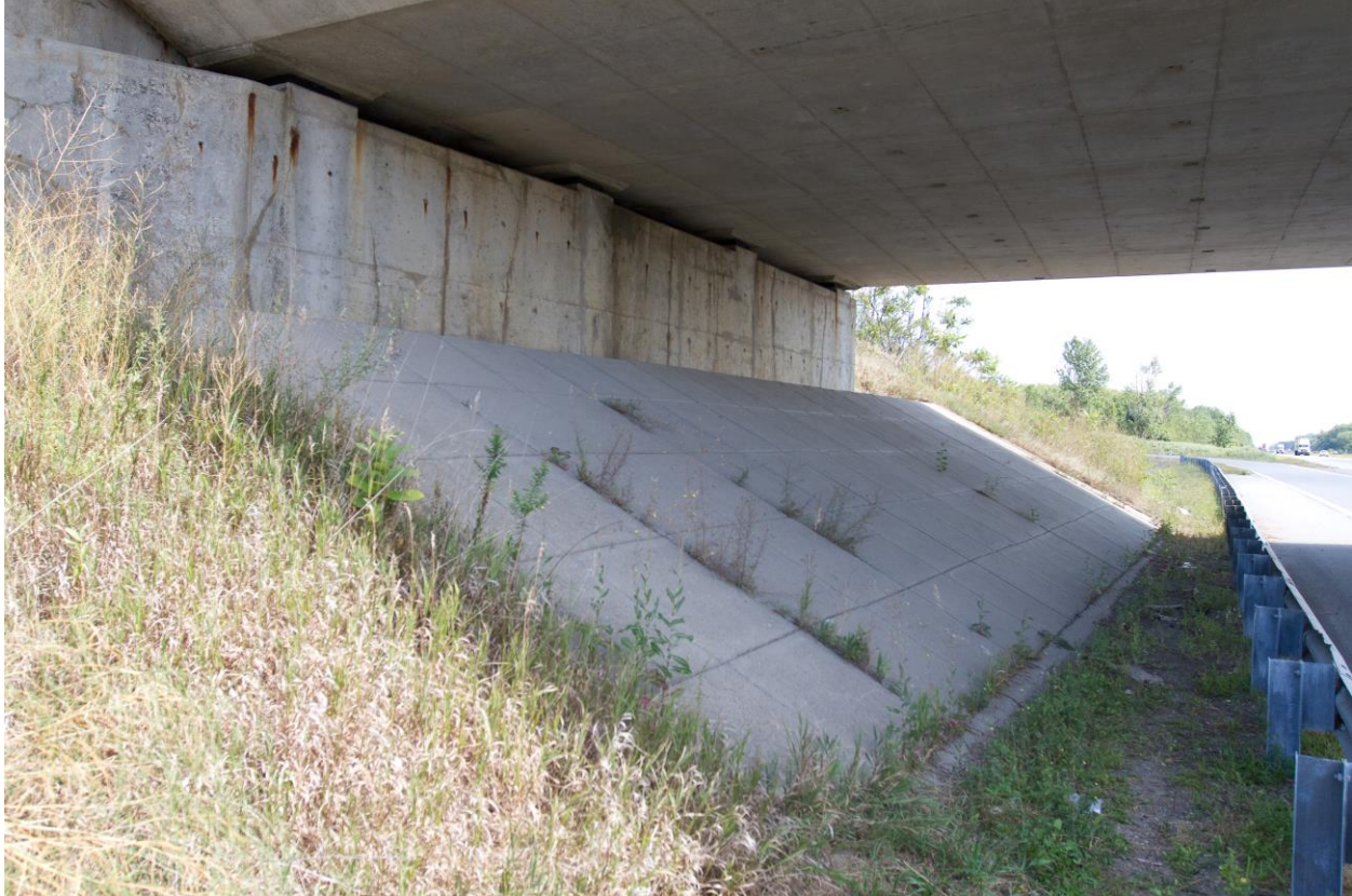
Photograph 2: Looking at the north abutment of the Brant Road 25 Underpass Structure. Random cracks were observed on the abutment wall. Sealant between the concrete panels appeared degraded at locations where grasses are growing. Weep holes were observed in the abutment wall. The toe of the front slope was vegetated with localized erosion of soil at ground surface (August 28, 2015).
