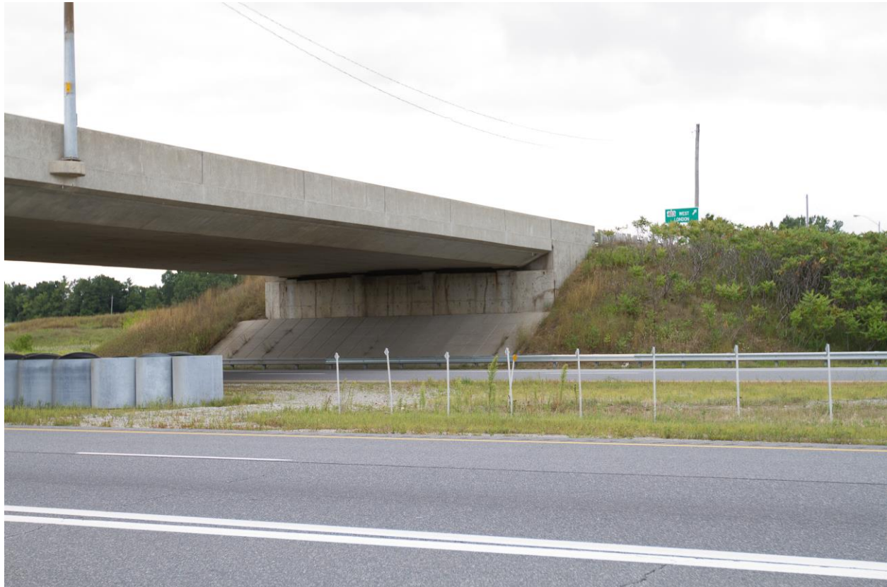
Photograph 7: Looking at the east wingwall and the adjacent slope of the north abutment of the Brant Road 25 Underpass Structure. Minor surficial cracks were observed on the wingwall. The slope is vegetated and effect of erosion on the slope face was not observed (August 28, 2015).
