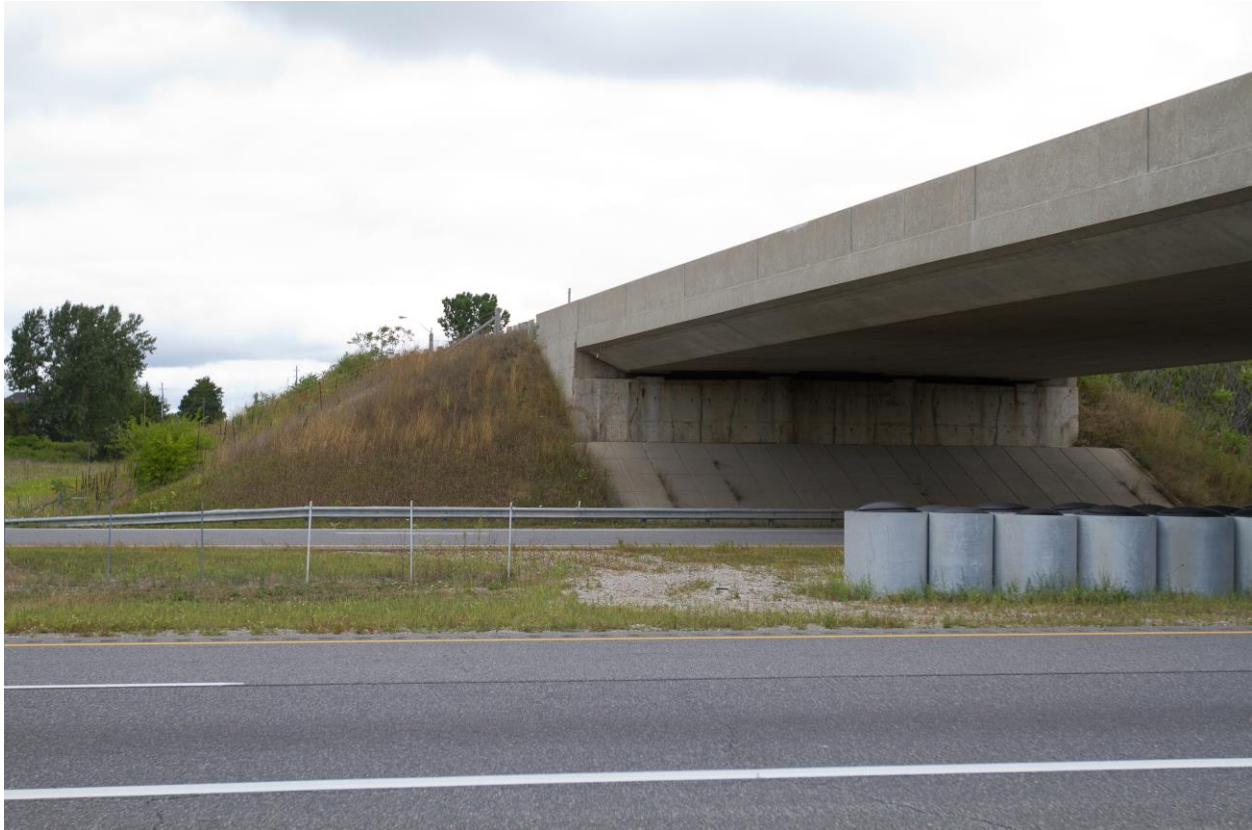
Photograph 6: Looking at the west wingwall and the adjacent slope of the north abutment of the Brant Road 25 Underpass Structure. Surficial cracks were observed on the wingwall. The slope is vegetated and effect of erosion on the slope face was not observed (August 28, 2015).
