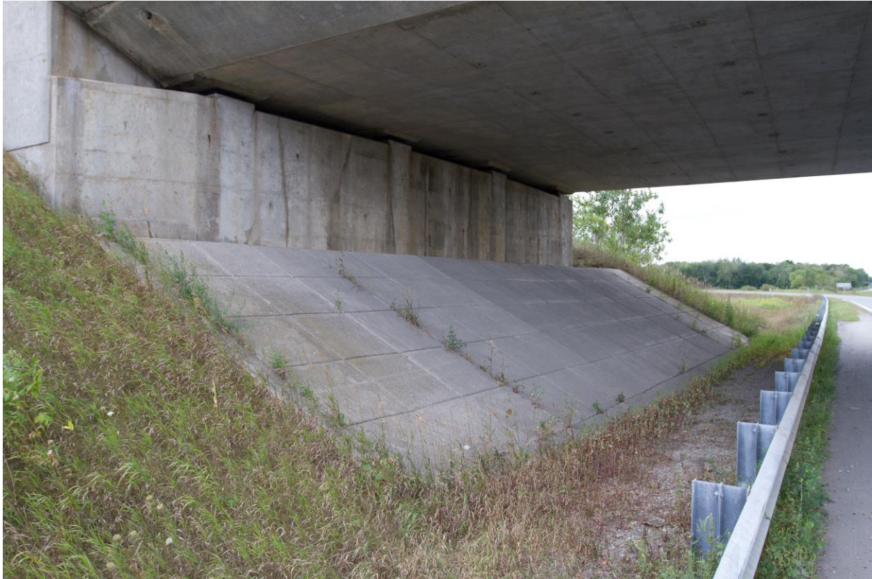
Photograph 1: Looking at the south abutment of the Brant Road 25 Underpass Structure. Random cracks were observed on the abutment wall. Sealant between the concrete panels appeared degraded at locations where grasses are growing. Weep holes were observed in the abutment wall. The toe of the front slope was vegetated with localized erosion of soil at ground surface (August 28, 2015).
