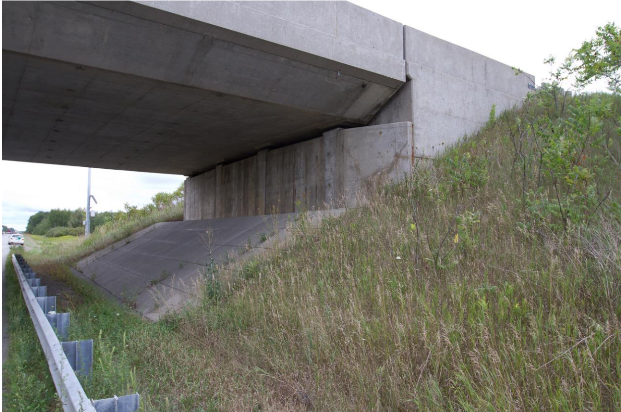
Photograph 5: Looking at the west wingwall and the adjacent slope of the south abutment of the Brant Road 25 Underpass Structure. Surficial cracks were observed on the wingwall. The slope is vegetated and effect of erosion on the slope face was not observed (August 28, 2015).
