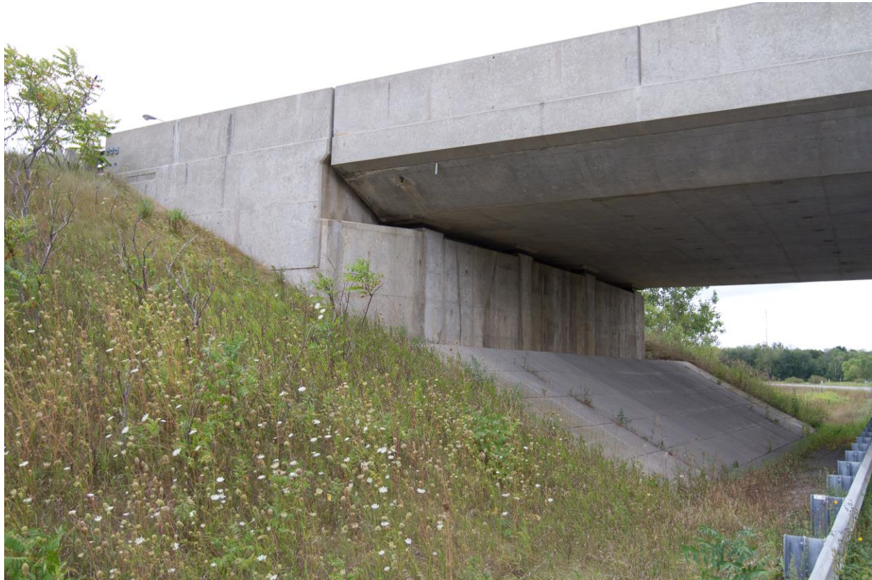
Photograph 4: Looking at the east wingwall and the adjacent slope of the south abutment of the Brant Road 25 Underpass Structure. Surficial cracks were observed on the wingwall. The slope is vegetated and effect of erosion on the slope face was not observed (August 28, 2015).
