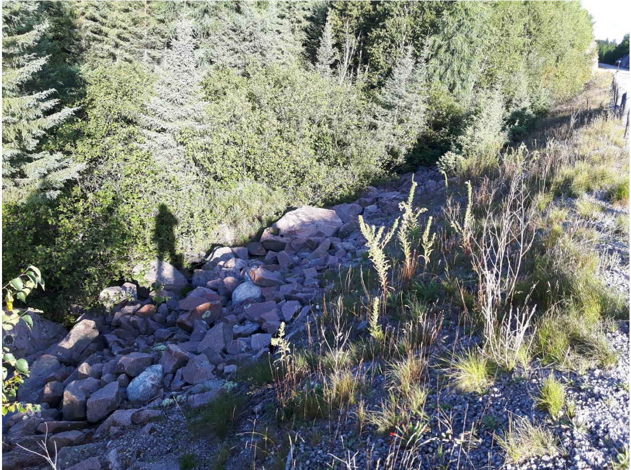
Photograph 3 –Rock fill at the toe of the embankment near the existing culvert
