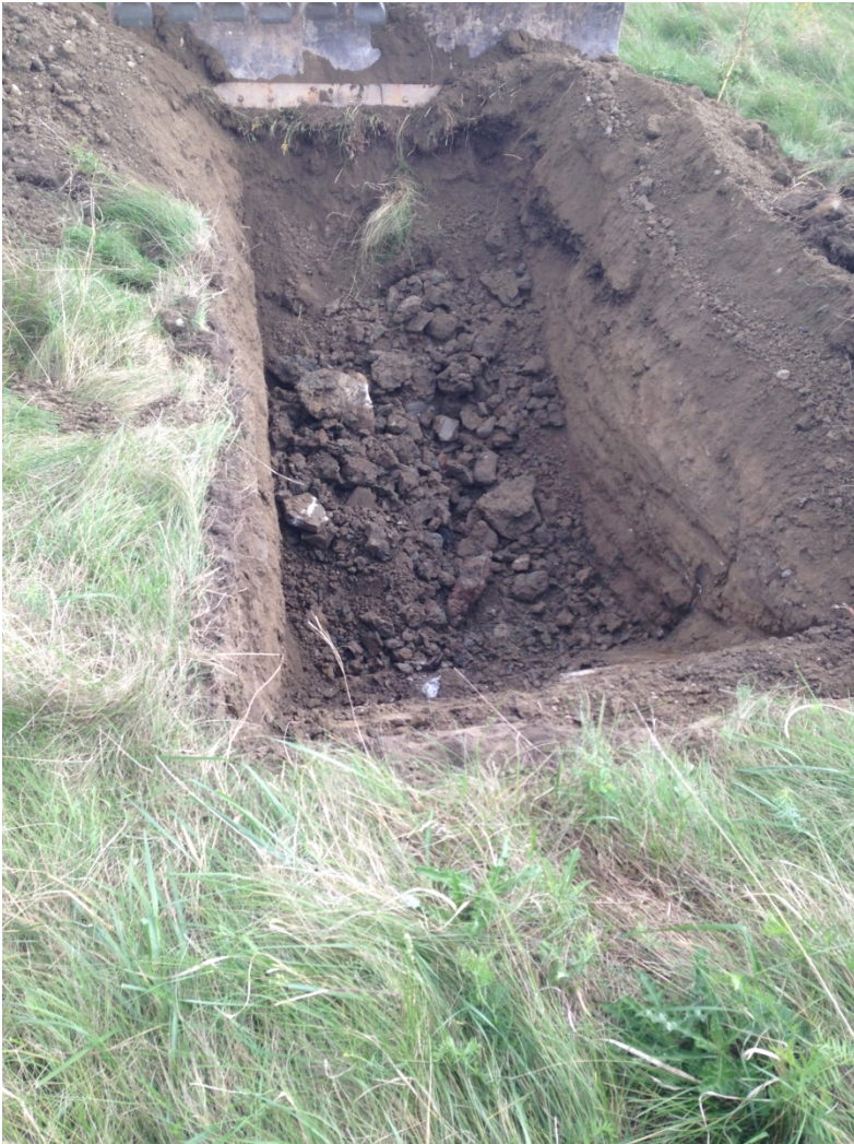
Photograph G1: Test Pit 1 during excavation. Cobbles and boulders were encountered in the excavation.
