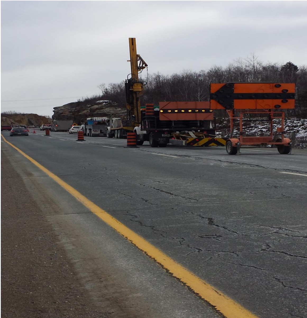
Photograph P2: Looking west from the existing Highway 17 median. Borehole 101-2 advanced using the Sonic drilling techniques at this location. (December 1, 2014)
