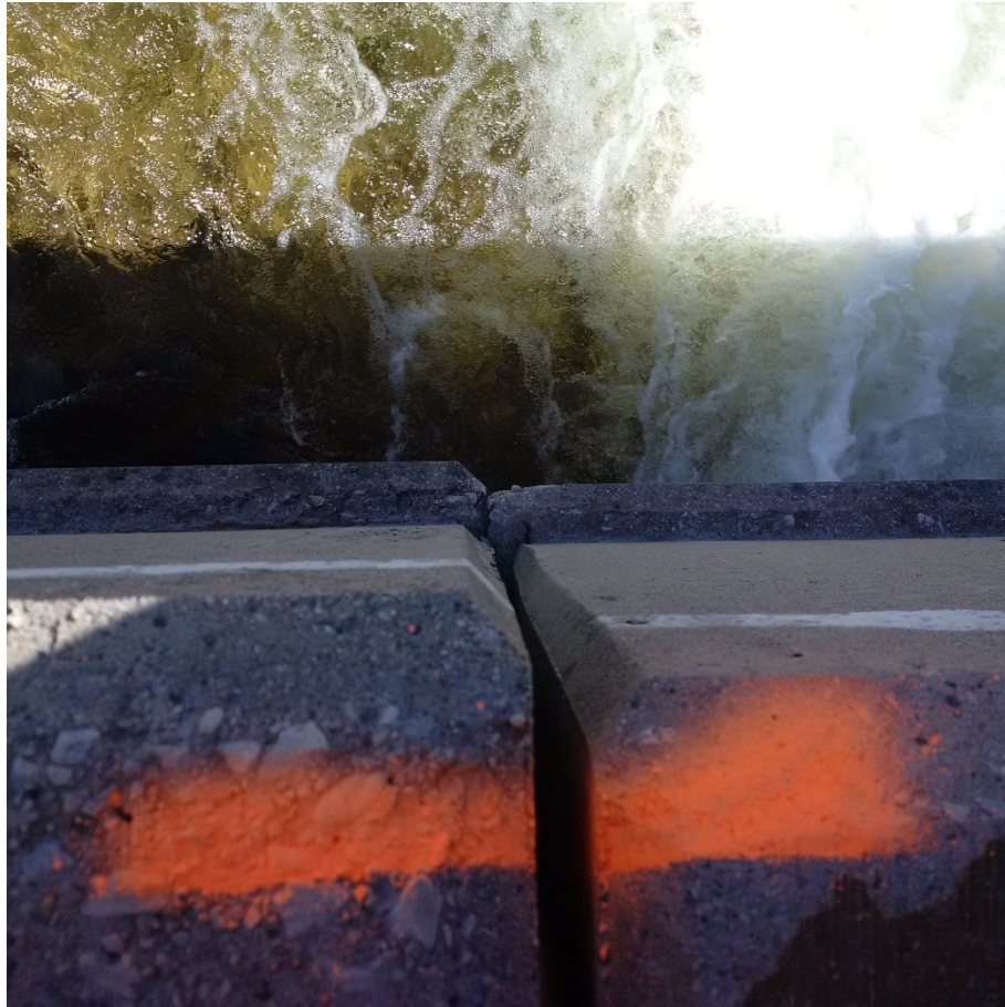
Photograph 6: Note retaining wall movement at south elevation (outlet) of Culvert Site 8-342/C.
