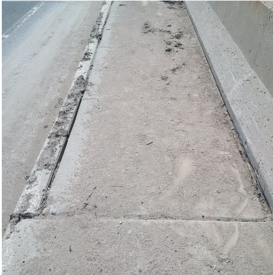
Photograph 7: Note settlement of west sidewalk at Culvert Site 8-342/C.
