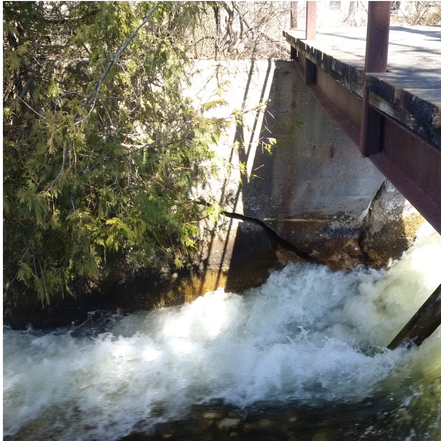
Photograph 5: Note significant cracking of north wall of spillway at inlet of north culvert.
