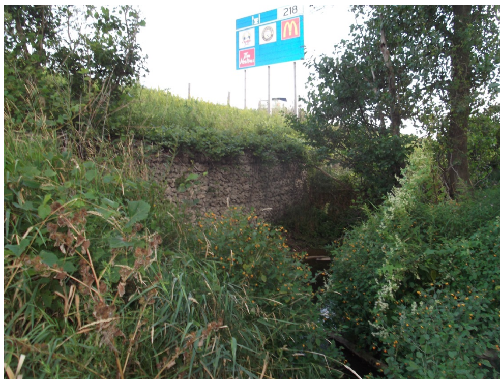
Photograph 2: Northeast gabion retaining wall.
