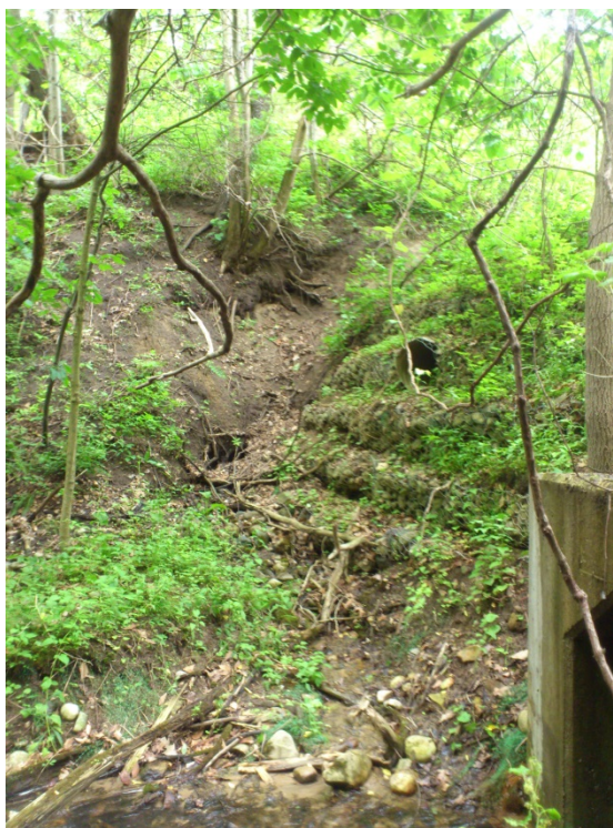
Photograph 6: Looking south at erosion channel adjacent to south edge of gabion wall (June 11, 2015).
