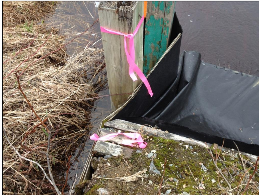
Photograph 7: Temporary Benchmark on Northeast Corner - Spike on Top of Culvert (May 2014)
