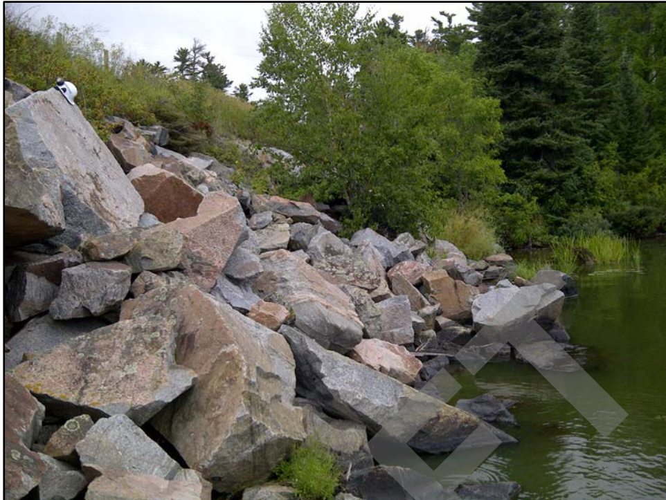
Photo 8: Large rock fill along toe of east slope (August 2012).
