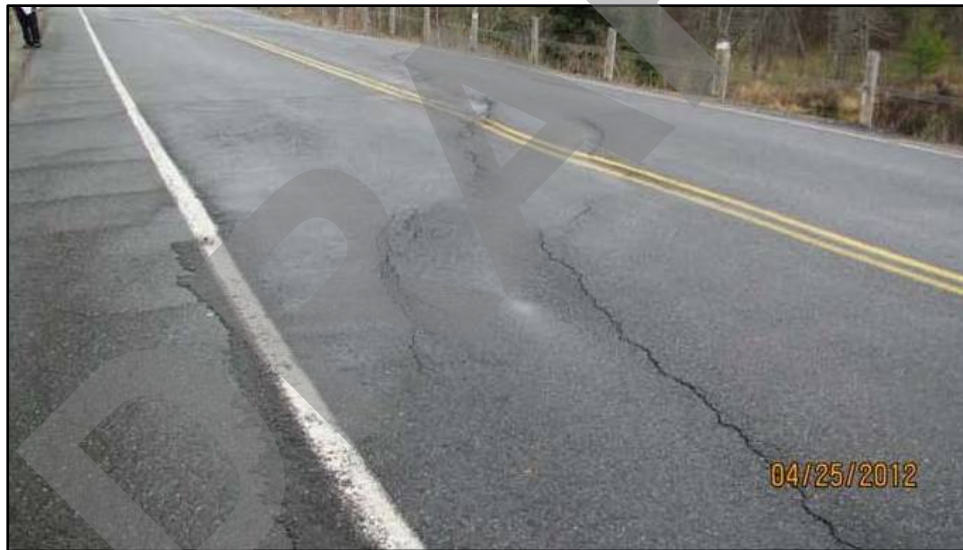
Photo 4: Cracking April 2012 (provided by MTO).
