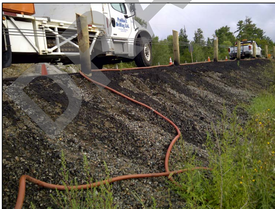
Photo 7: Erosion of East slope by surface water runoff (August 2012).
