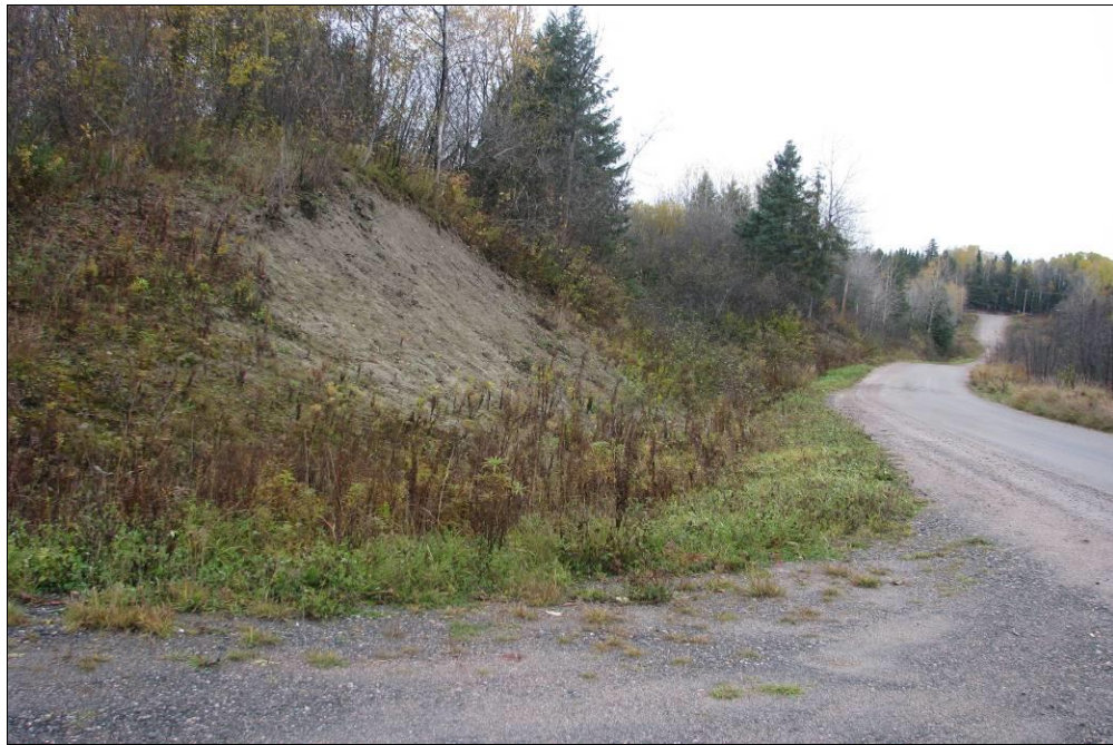
PHOTOGRAPH 27: Looking north from west shoulder of McNutt Road. Visible erosion on 3 m high sandy silt slope surface on west side of McNutt Road about 350 m south of the intersection of McNutt Road and Trunk Road. (October 17, 2012)
