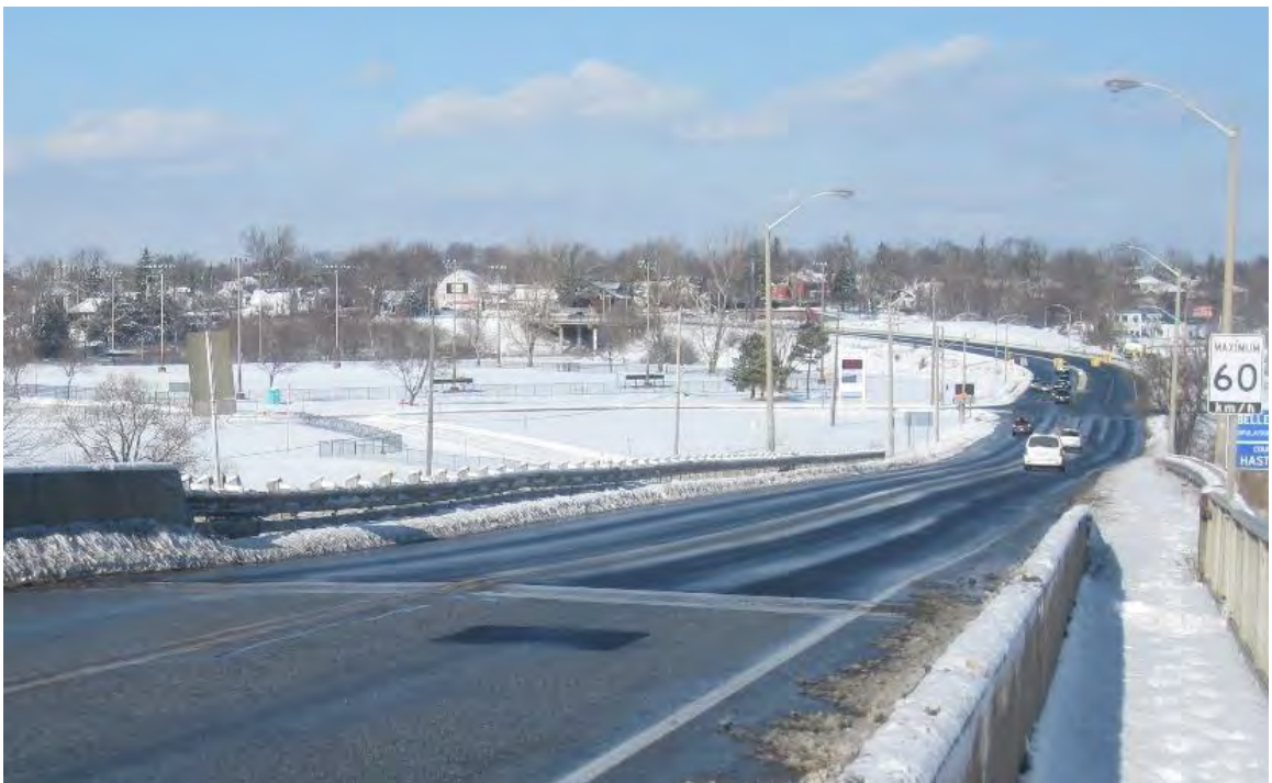
North approach looking north; possible approach settlement
