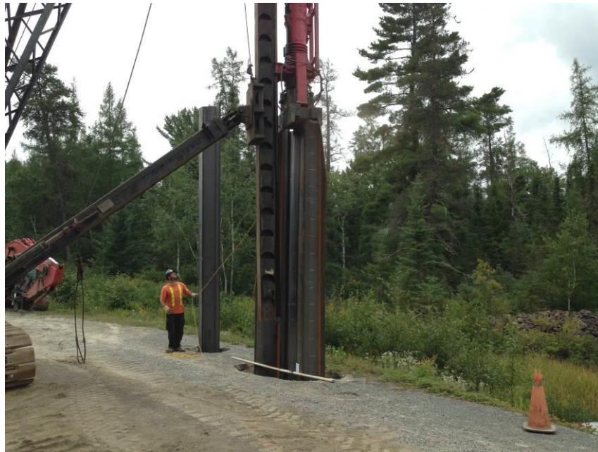
Toe of Test Pile No. 4 after Removal from Ground
