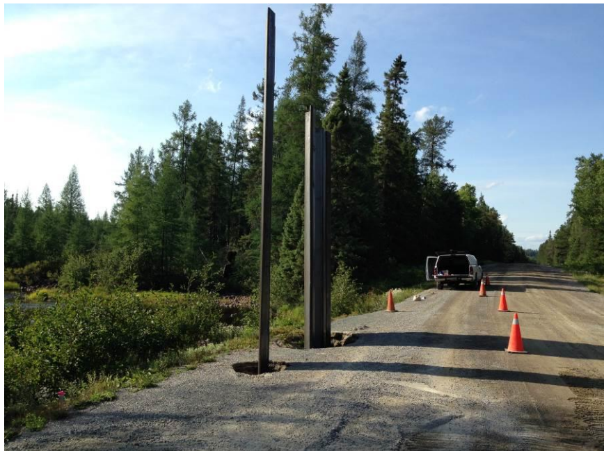
Test Sheet Piles 1 to 4 - After Vibratory Installation
