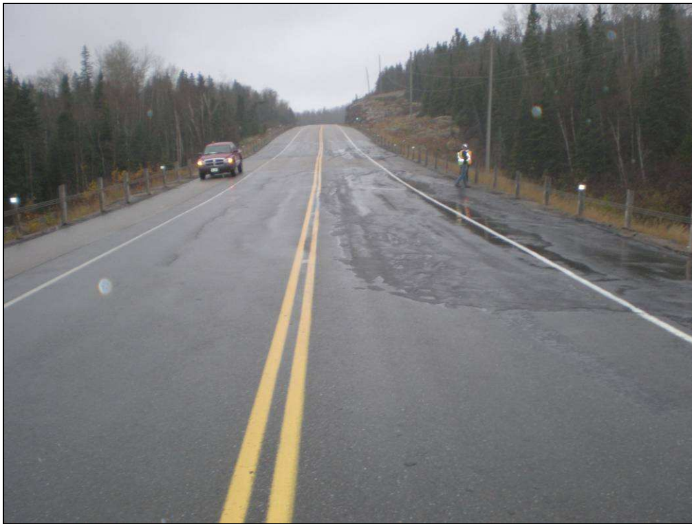
Figure 1, Patching Along West Bound Lane, Looking West
