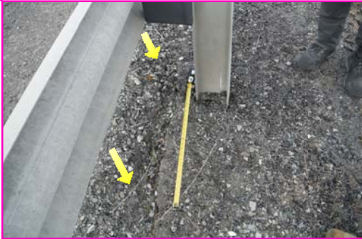
Close-up view of crack at the slope crest at approximately Sta. 15+375.
