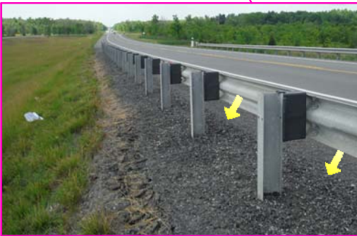
Crack along slope crest running parallel to and on the west side of the guide rail.
