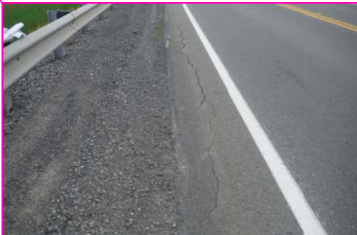
Crack on the partially paved shoulder on the east side of south embankment looking south, located about 1.5 m west of guide rail.
