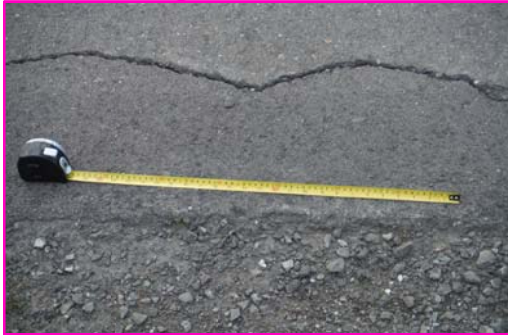
Closer view of crack on the partially paved shoulder on the east side of south embankment at approximately Sta. 15+470.
