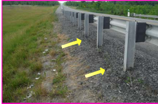
Crack along slope crest running parallel to and on the east side of the guide rail.
