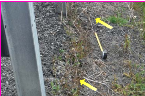
Close-up view of crack along slope crest on the west side of south embankment.
