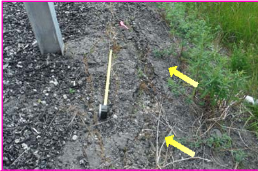
Crack along slope crest about 1 m west of guide rail on the west side of south embankment.
