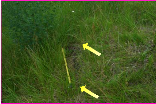
Cracks near the toe of mid-height berm on the west slope of south embankment.
