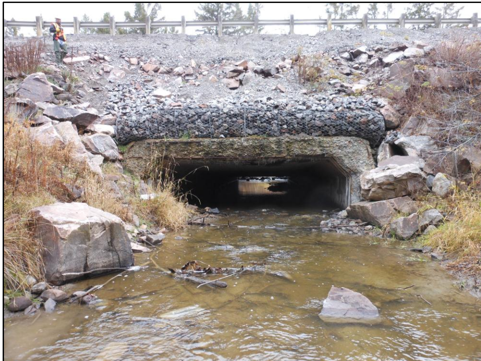
Photograph 2: Embankment north slope and culvert outlet (received from MMM December 2012).
