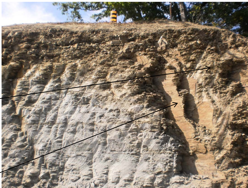
View of the North Face Showing Prominent Joint Sets and Deeper Weathering Near the River Bank
