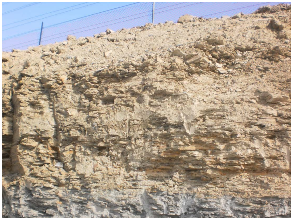
Deeper Weathered Zone on South Rock Cut
