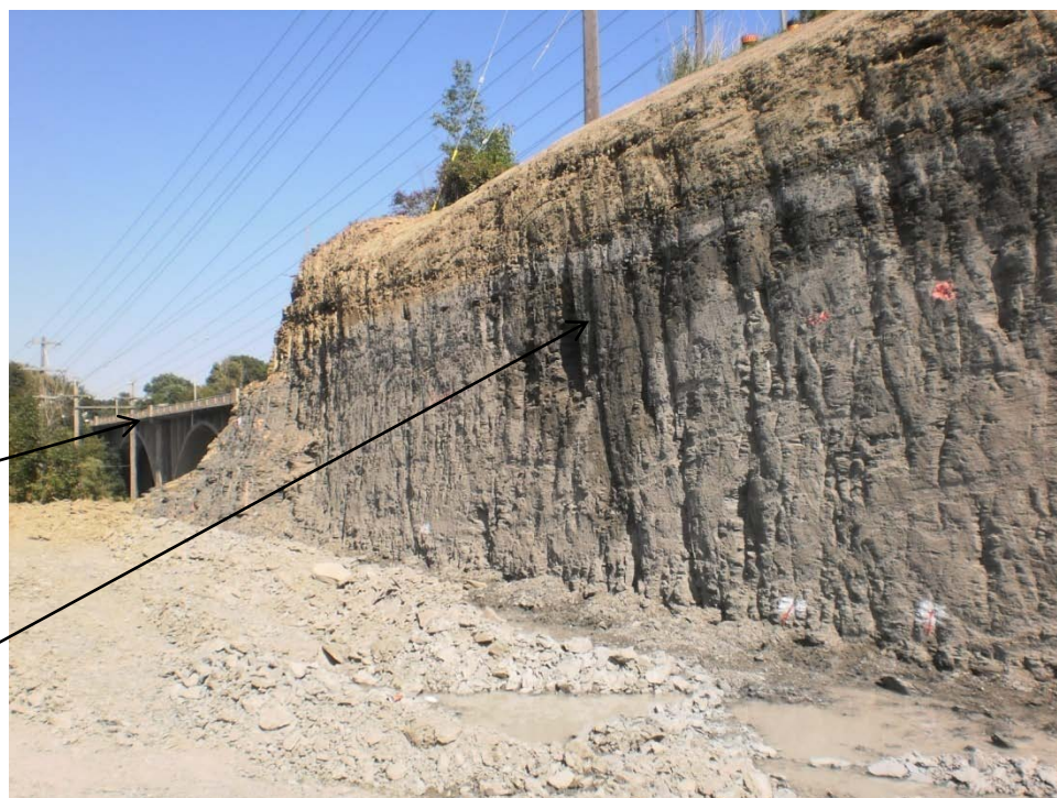
View of South Rock Face Showing Groundwater Seepage
