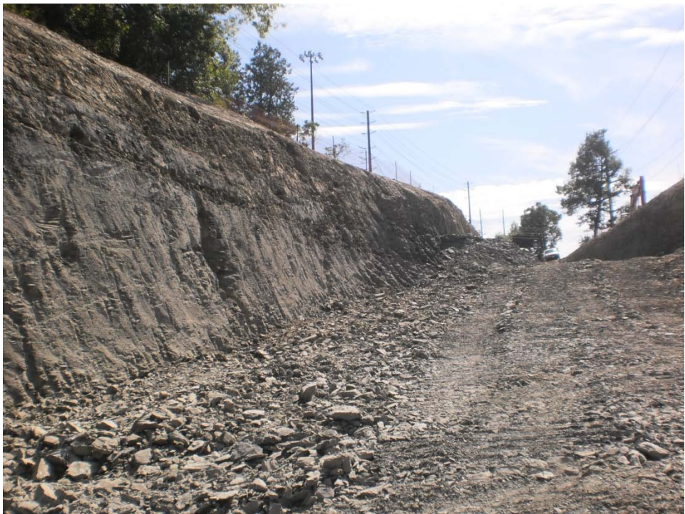
View of South Rock Cut Looking West Showing Deep Weathered Zone
