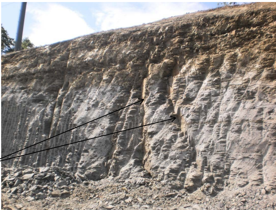
Typical Rock Cut Face Showing the Upper Weathered Zone at the Top of the Cut
