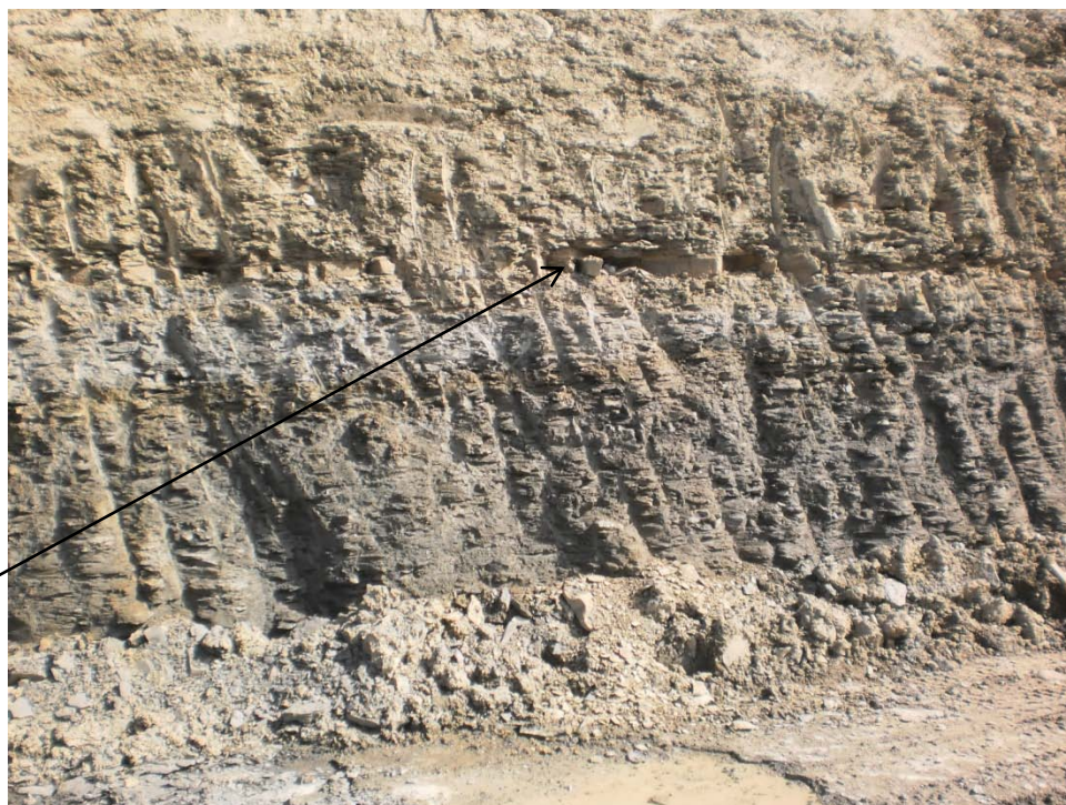
Typical Cut Face Showing Ravelling Failures and Slabs in the Harder Interbedded Layers
