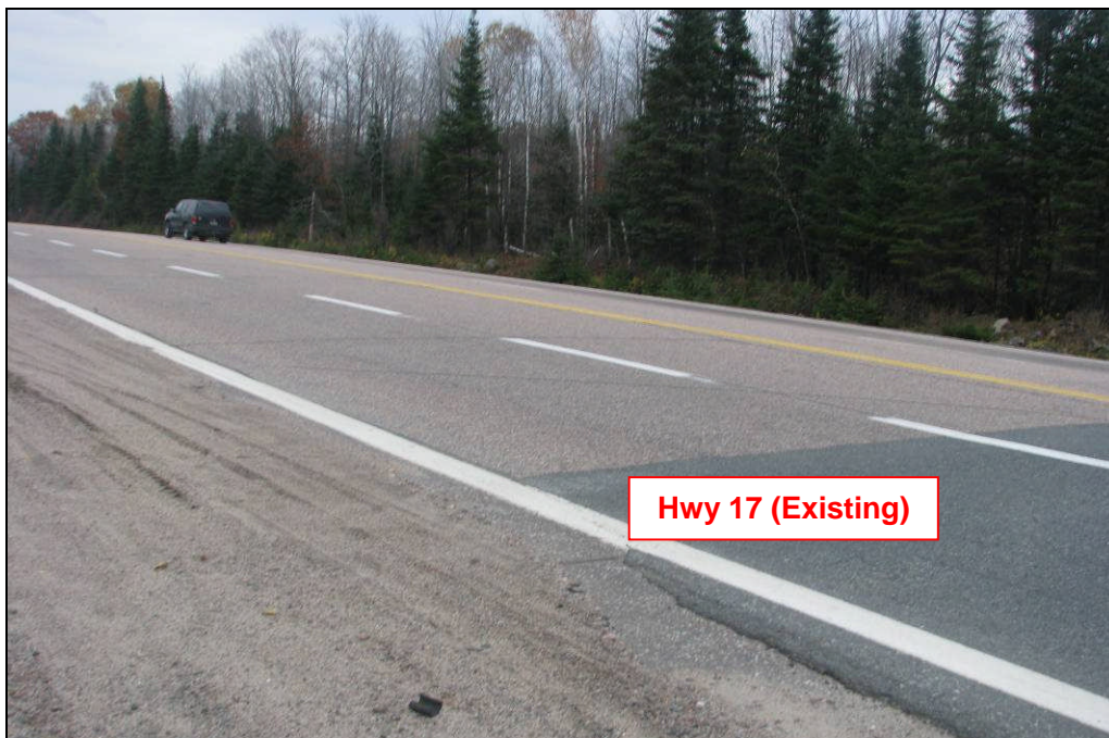
Photograph P26: Looking southwest from north shoulder of Hwy 17 (Existing) at proposed Hwy17 (preferred) east crossing area. Shallow overburden up to 2m thick over bedrock based on Geotechnical Survey Data (GWP 174-98-00). (October 18, 2012)
