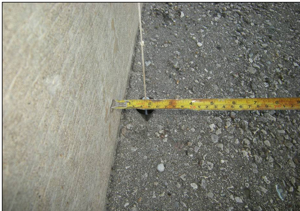
Photograph 10: Overhang measurement was taken from approximately 20 m north of the south end of the retaining wall and it was approximately 41 mm (1 5/8 in.) (October 8, 2011)
