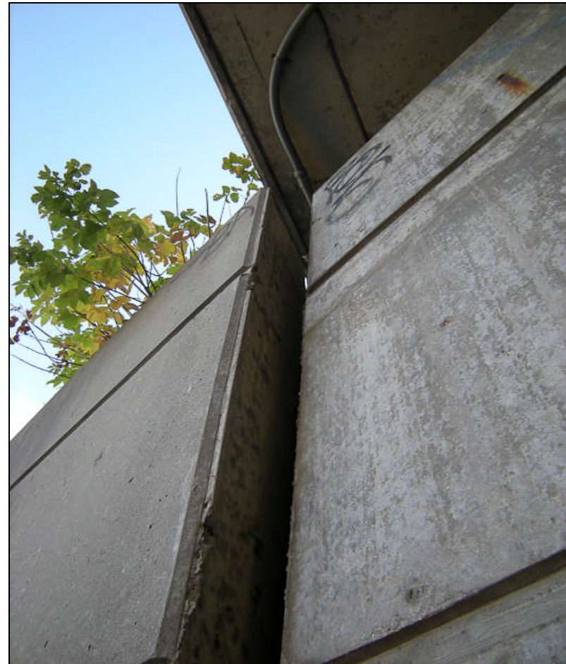
Photograph 6: Close-up view of south end of retaining wall. Measurement to face of abutment was taken at retaining wall/abutment joint, approximately 64 mm (2.5 in.) at 0.3 m (1 ft.) above ground surface, 127 mm (5 in.) at 1.8 m (6 ft.) and 230 mm (9 in.) at top of retaining wall. (October 8, 2011)
