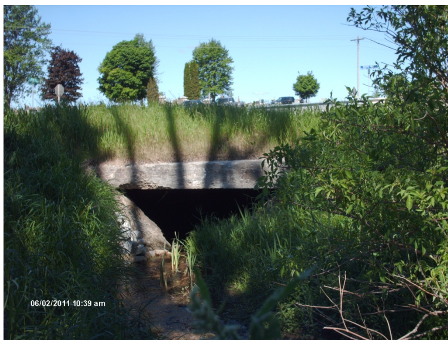
Photograph 3: Triangular inlet for Roger Drain in northeast quadrant.
