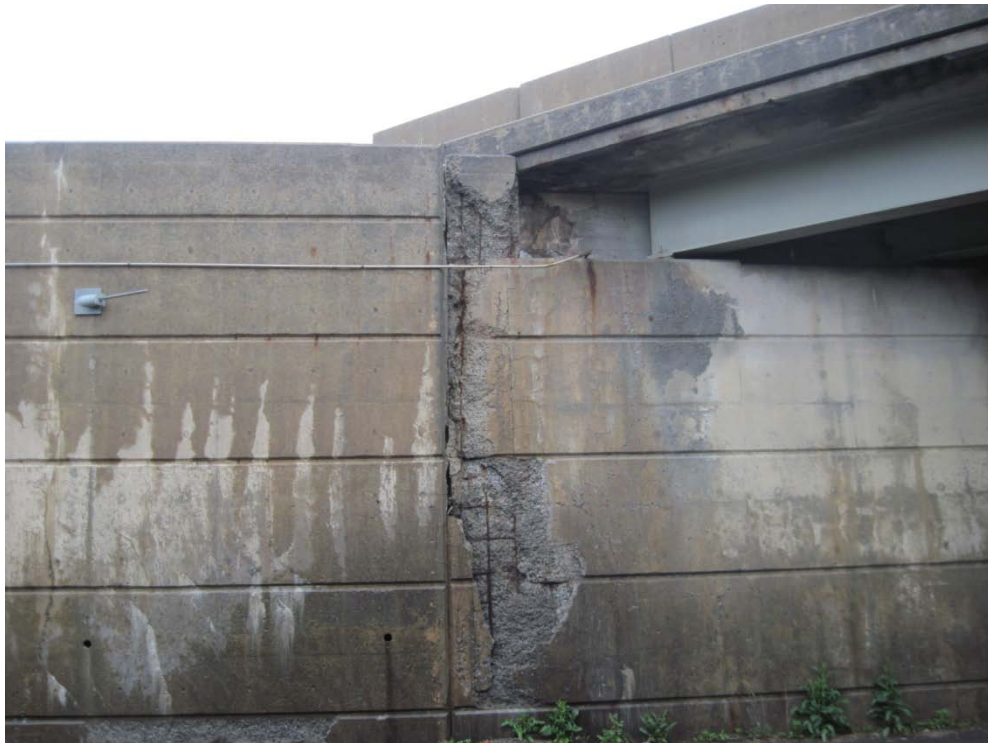
Photo 2: Severe spalling at north end of west median retaining wall.
