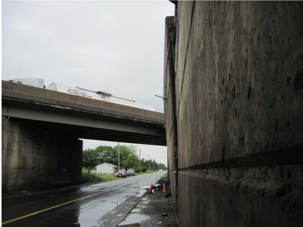
Photo 3: Cornwall Centre Road looking south from west abutment of WBL structure. Note forward tilt at west, median retaining wall.
