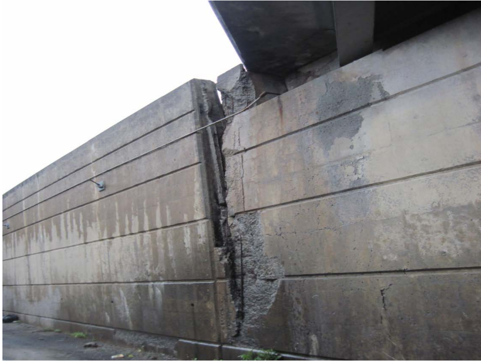
Photo 1: West median wall at west abutment of WBL structure. Note severe spalling and tilting of median wall.
