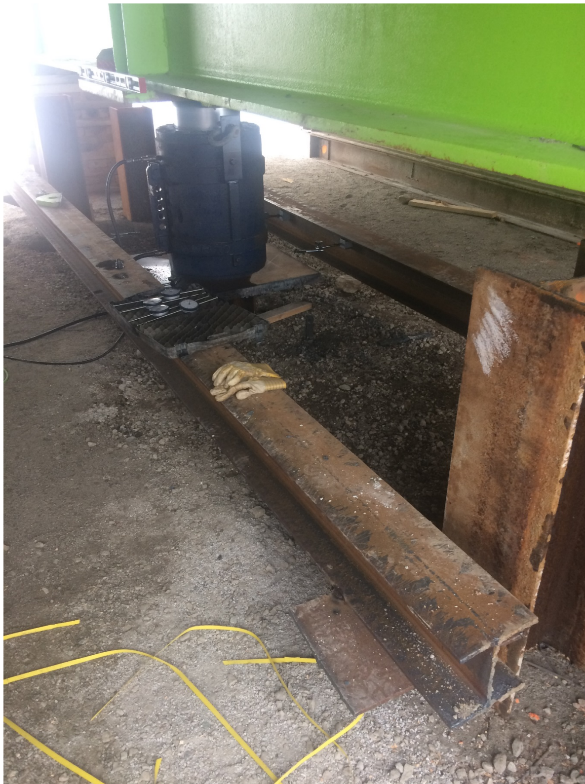
Photograph 4: Hydraulic jack set-up
