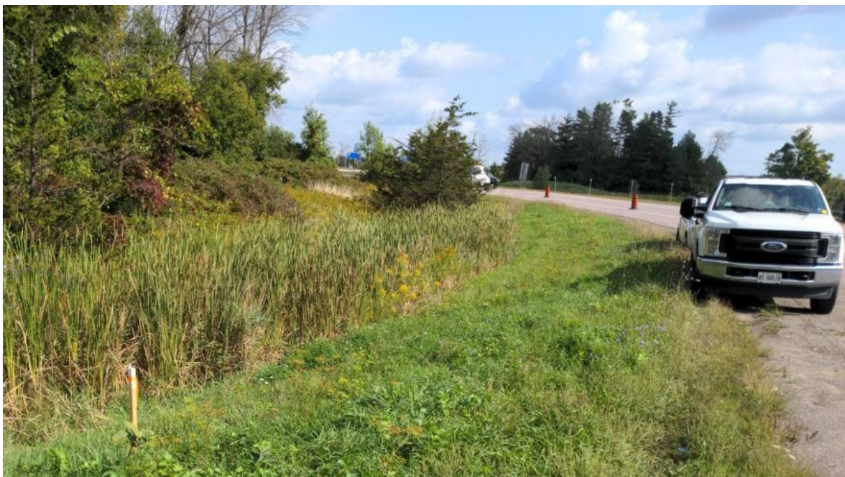
Photograph 2: Looking northeast at Borehole C-08 along Highway 401 N/S-W on-ramp near proposed culvert inlet (September 2022)
