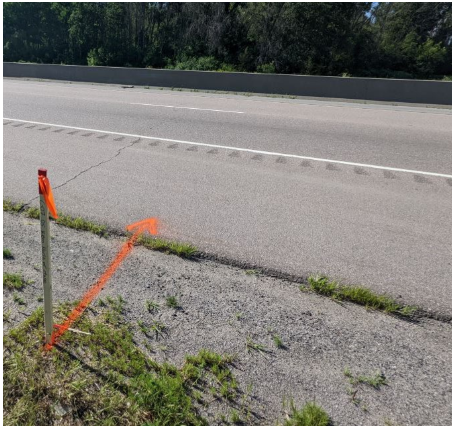
Photograph 1: Looking north across Highway 401 from Borehole C-06 along proposed culvert alignment (May 2022)
