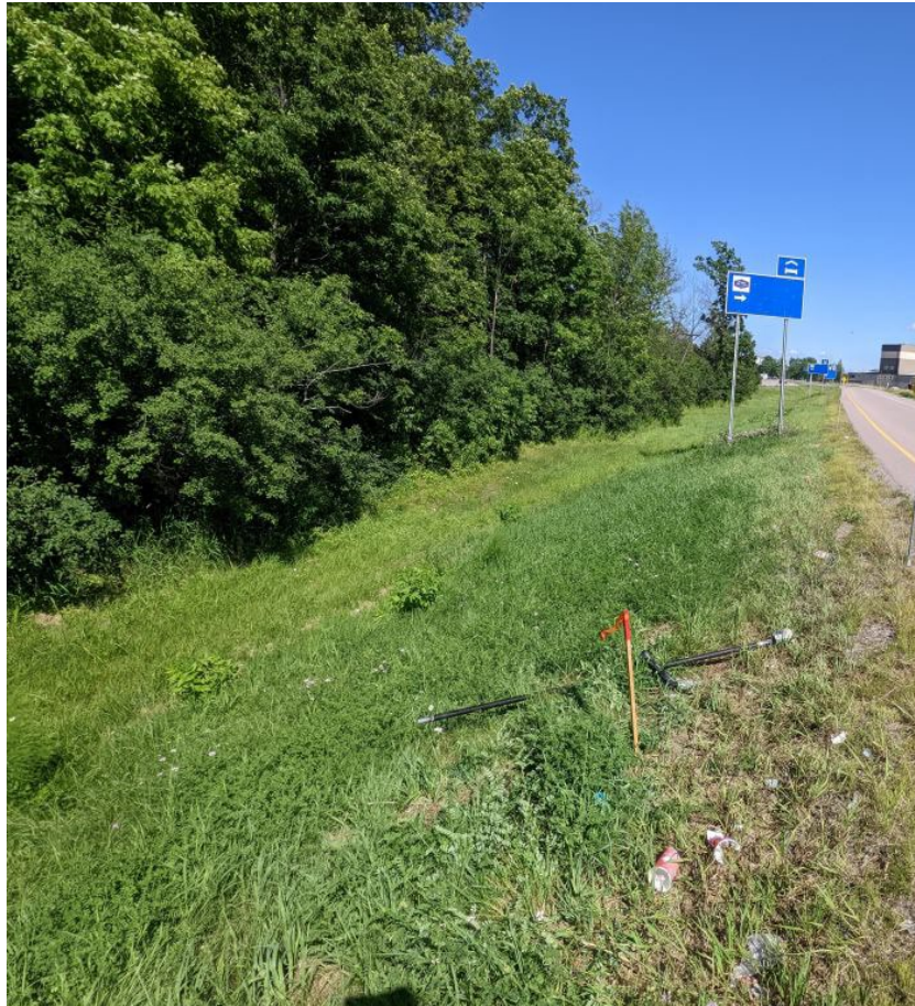
Photograph 1: Looking southeast along the Highway 401 W-N/S Ramp from Borehole C-11 (July 7, 2022)
