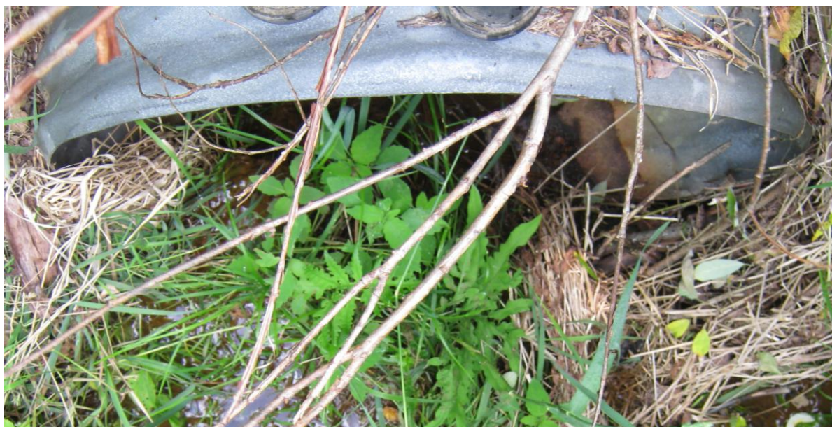
Culvert Outlet – Site A
