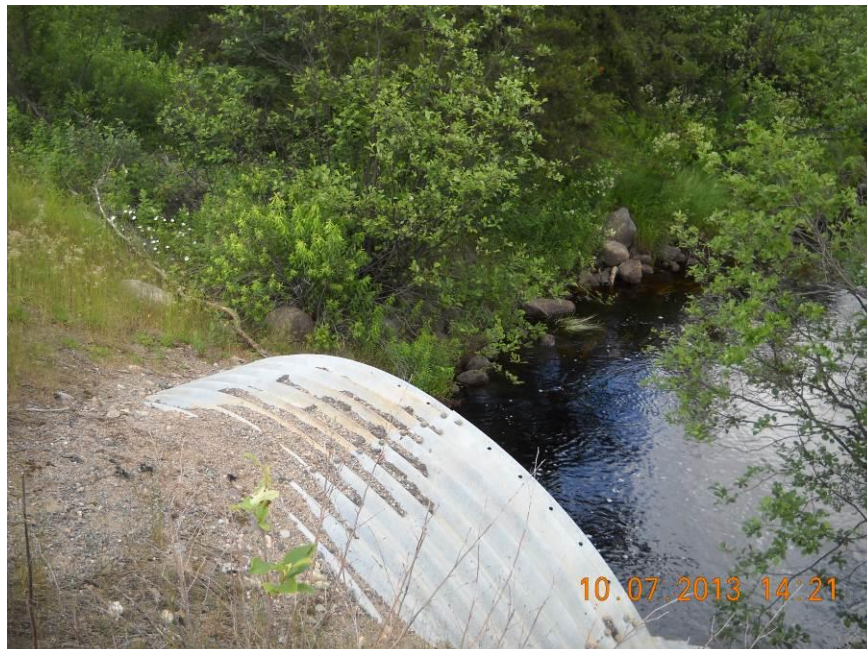
Culvert Outlet – Note cobble/boulders in and around creek
